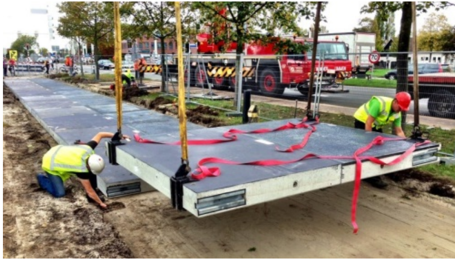
Figure 5. Solar panels that form the bike path (source: www.bbc.com/capital ).
