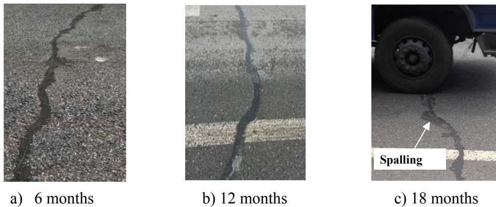
Figure 8. Cracks after repaired for certain periods of time.
