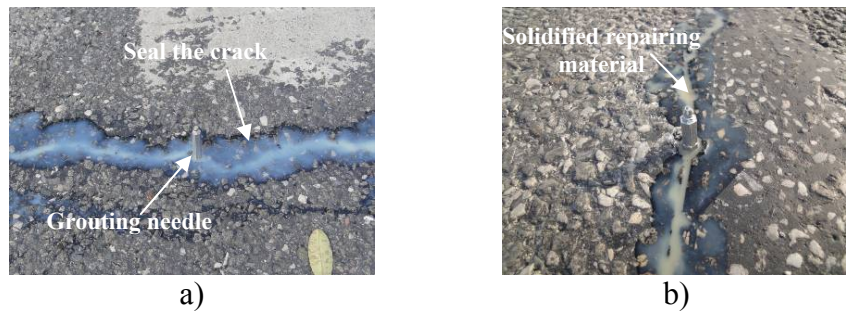
Figure 4. Crack sealed with chemical repairing material.
