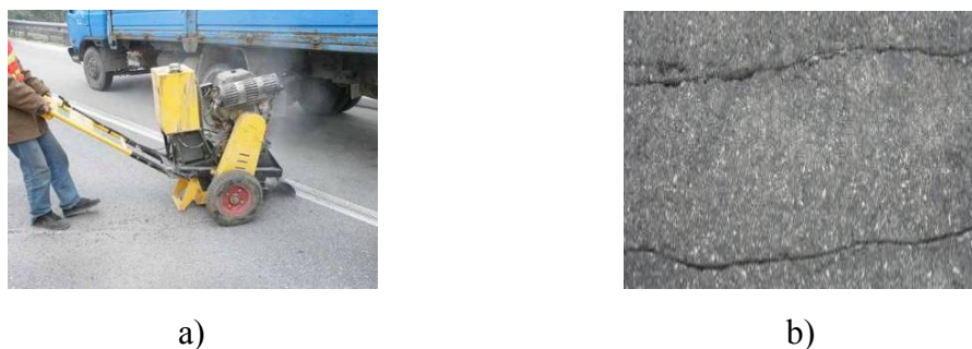
Figure 2. Grooving for cracks.
