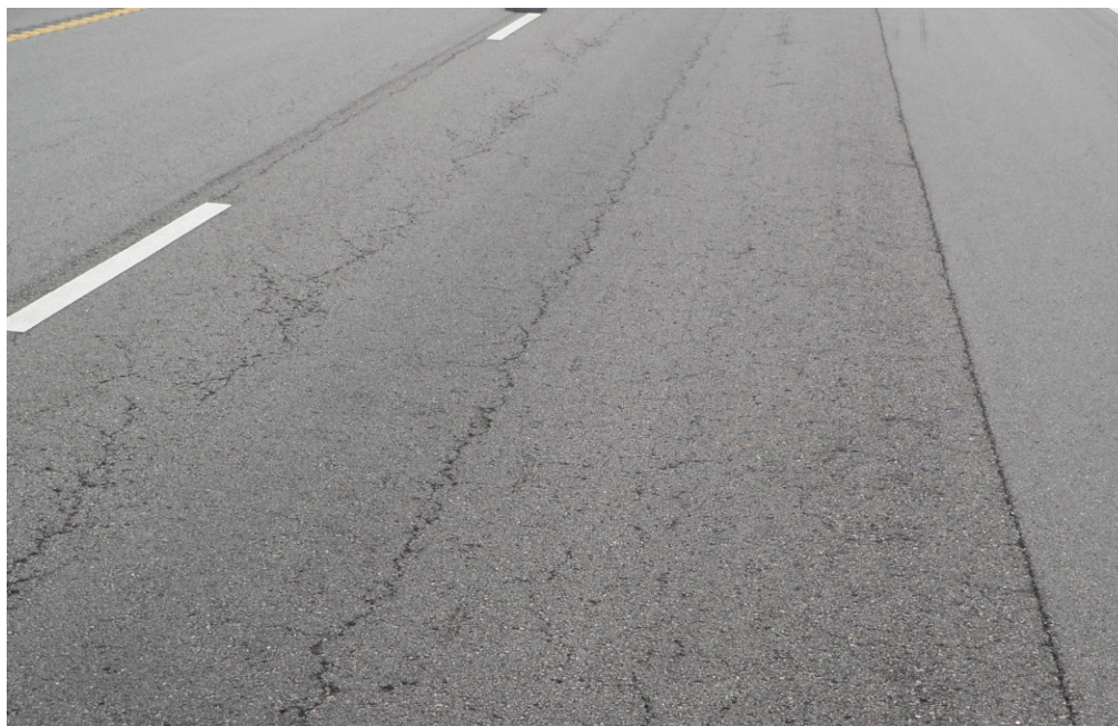
Figure 2. Fatigue cracking on missouri pavement.
