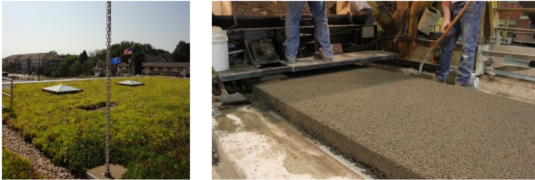
Figure 3. Bioinfiltration (left) and pervious pavement (right).
