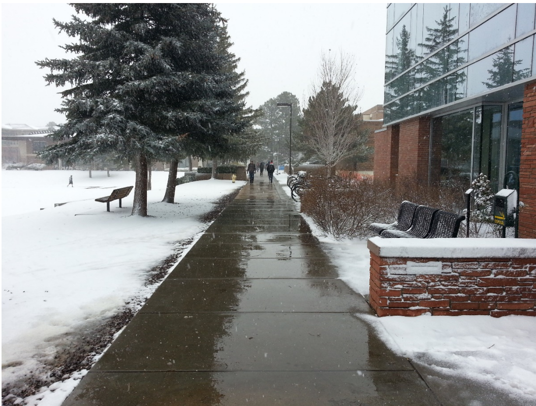
Figure 9. Heating Concrete Slabs in a snow say at 11 am (12/04/2013).
