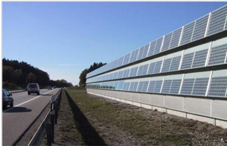
Figure 6. Zigzag patterns of solar panels on the sound barrier walls (source: www.photovoltaiik.eu ).
