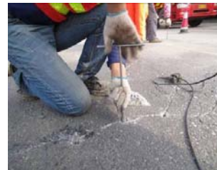
Figure 3. Installation of grouting needles.
