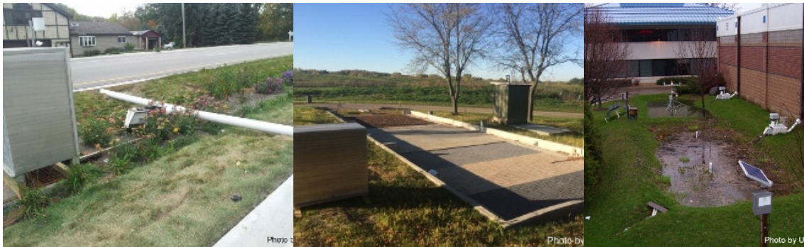
Figure 2. Bioswales, permeable pavement, and rain garden (courtesy of USGS).
