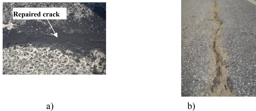
Figure 7. Curing for the repaired crack.
