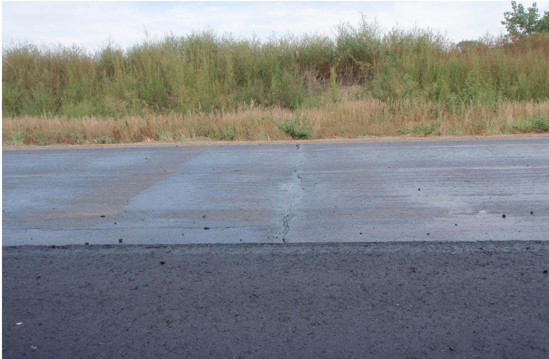
Figure 4. Inconsistent tack application.
