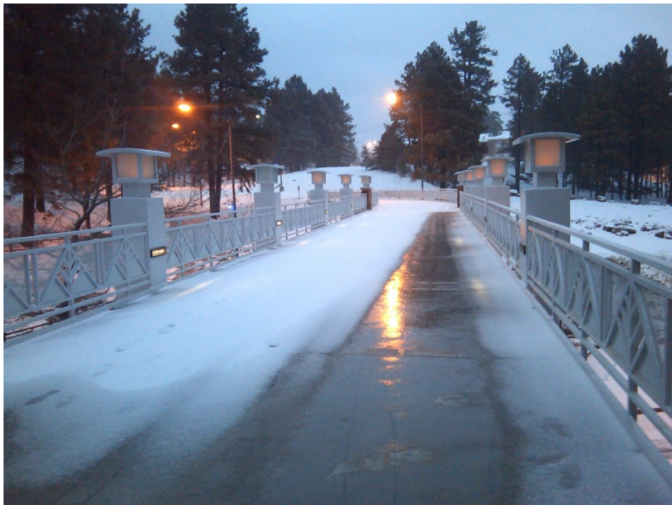
Figure 7. Heating and non-heating bridge deck comparison at the Suites Student Apartment, taken at 7am (01/28/2013).
