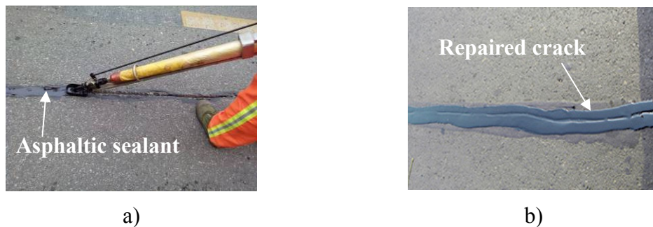
Figure 1. Conventional crack repairing method.
