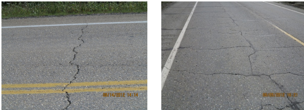
(a) Major transverse thermal cracks. (b) Lesser transverse thermal cracks.
