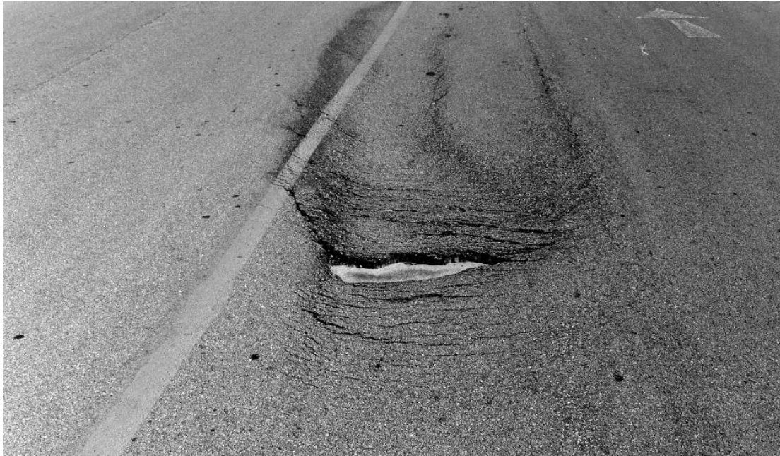
Figure 1. Slippage failure due to poor bonding.
