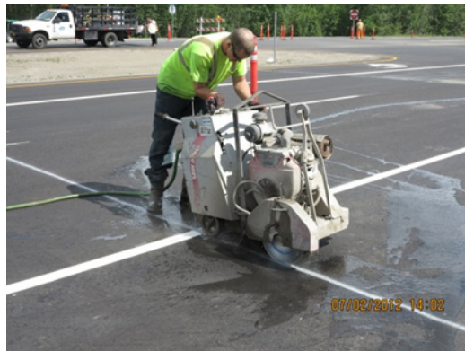
Figure 1. Precut work in the field.
