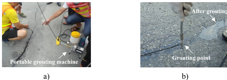
Figure 5. Grouting for the repair.
