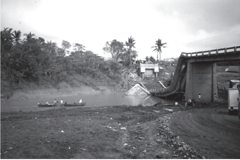
Photo 21.1 Bridge along Marhalika highway collapsing as a result of high flow discharge in deforested areas in Isabela Province, the Philippines (©DJ Snelder)
