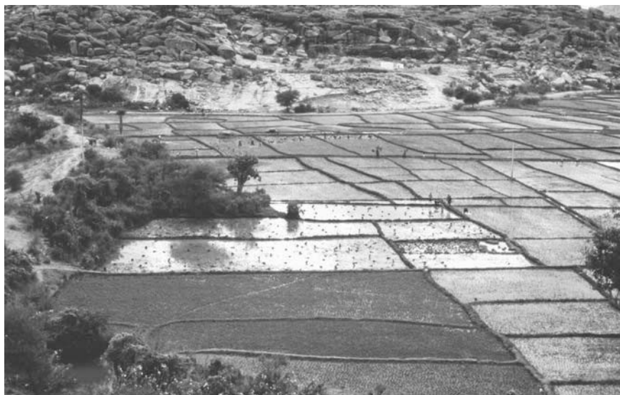
Figure 4.3 Abandoned Reservoir (left side of the image) Made Redundant by the Sixteenth Century Anegondi Channel. Fed by the Tungbhadra River, This Canal Made Rice Production Near the City Possible North of the River and Has Continued in Use until Today.
