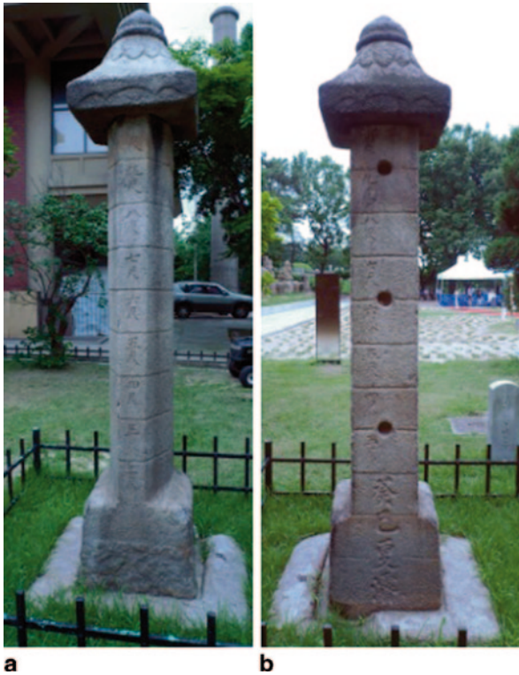
Fig. 8 Water-level Marker made of granite stone in 1773. a Front surface of the marker, ten Jucheok were inscribed each spaced a cheok about 21 cm and marked numbers from 2 to 10 cheok . b The holes bored into the back marker indicate the water-level as “flood,” “moderate,” “draught” from top down. Also inscribed “Dredge again at 1773”, 3 m high and 20 cm wide. Collection of the King Sejong Memorial Society, Seoul. (Photo courtesy of Nam MH)
