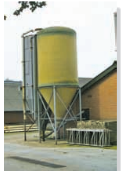
The volume of fertilizer contained within this silo can be determined using the second theorem of Pappus and Guldinus. (© Russell C. Hibbeler)
