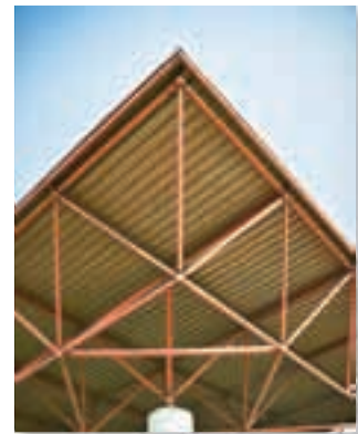
Typical roof-supporting space truss. Notice the use of ball-and-socket joints for the connections. (© Russell C. Hibbeler)
