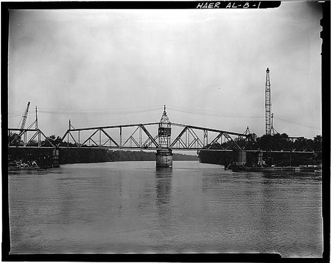
Figure 8-2. Bridgeport Swing Span Bridge, Bridgeport, AL (demolished), built 1890 (HAER ALA,36-BRIPO.V,1-).
