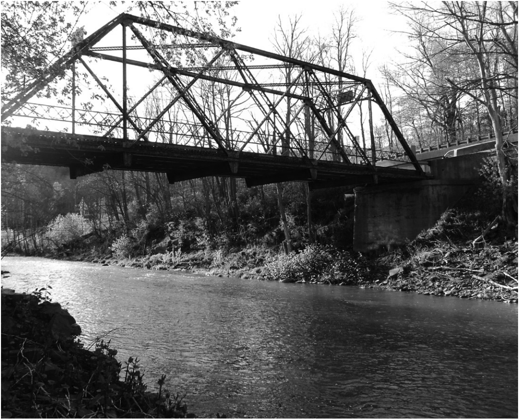
Figure 1-7. Double Warren truss bridge (1907), Bronson Road over Sugar Creek, near Troy, PA. Source: Photograph by the author.
