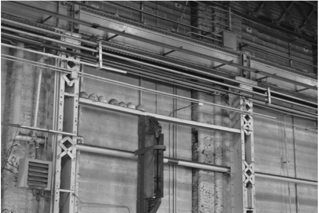
Figure 8-4. A continuous crane girder in the Pennsylvania Railroad Juniata Locomotive Shops (1889). Source: Photograph by Sikander Porter-Gill.
