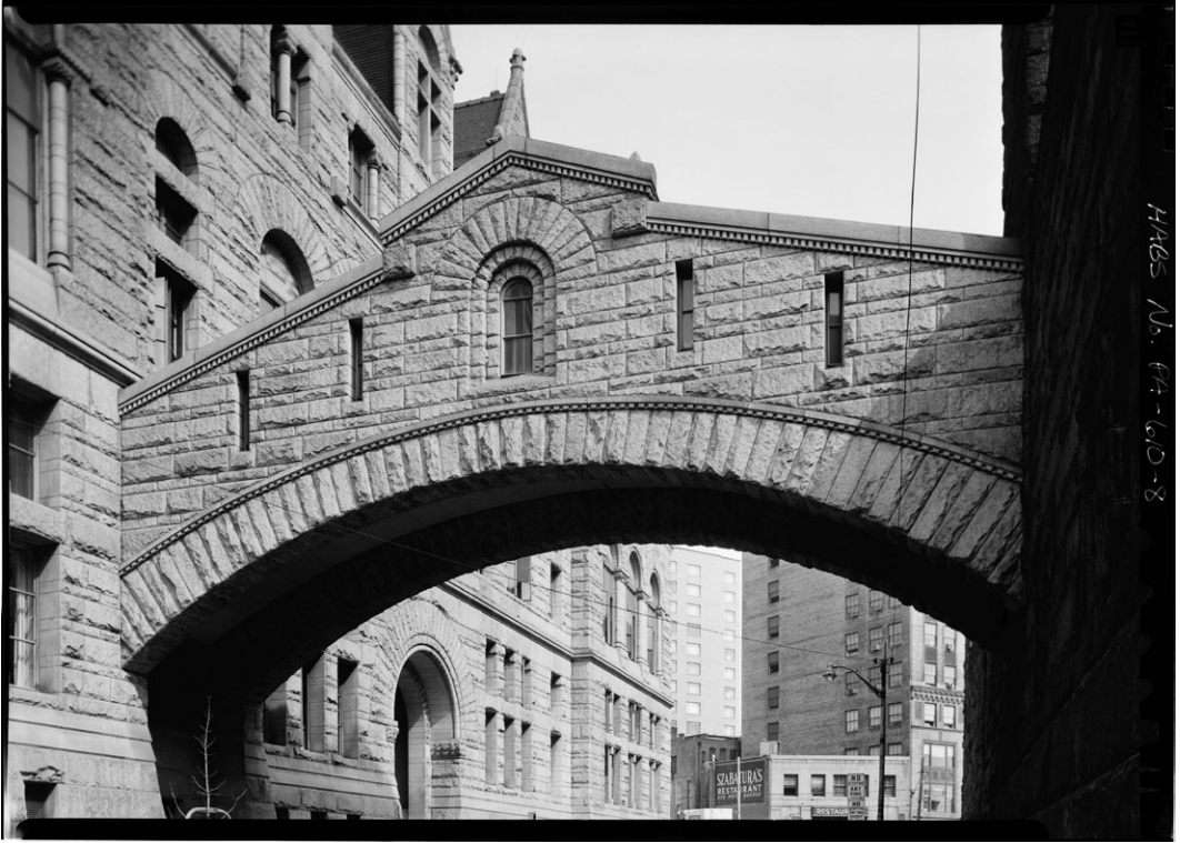
Figure 2-5. The Bridge of Sighs from H.H. Richardson’s Allegheny Courthouse and Jail, Pittsburgh, PA (1884-6) (HABS PA,2-PITBU,29-8).
