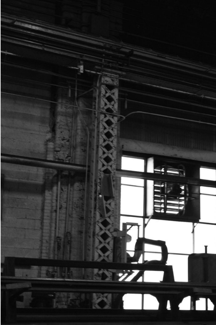
Figure 9-2. Lattice wrought-iron or steel columns at Juniata Locomotive Shops, Altoona, PA, 1889. Source: Photograph by Sikander Porter-Gill.
