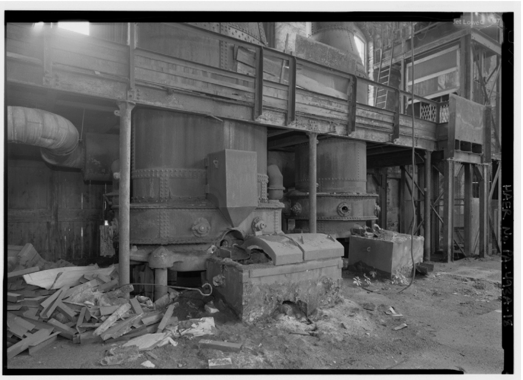
Figure 9-1. Cast-iron column at Phoenix Iron Company foundry building, 1882 (HAER PA,15-PHOEN,4A-18).
