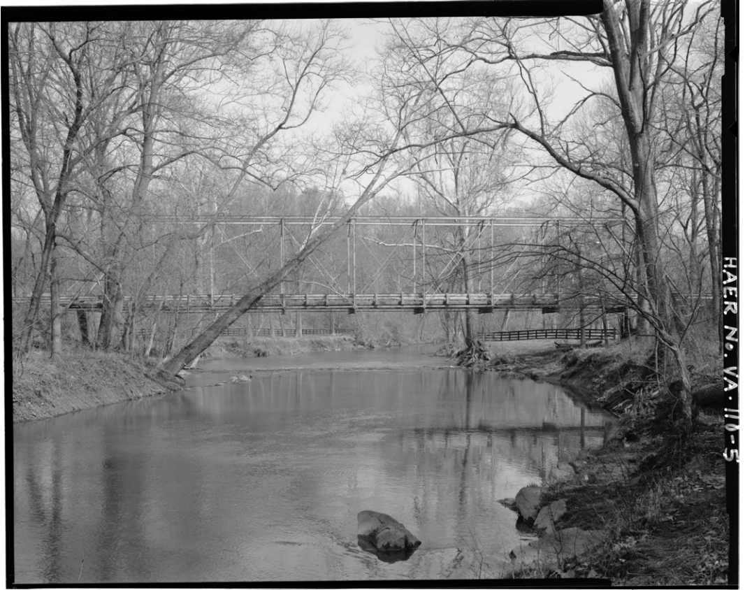
Figure 7-9. Example of eight-panel Pratt truss road bridge, Waterford, Loudon County, VA (HAER VA,20-CLARK.V,1-5), constructed in 1889.
