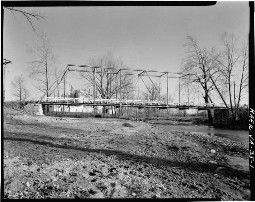
Figure 16-2. Thacher truss bridge, Rockingham County, VA, 1898 (HAER VA, 83-BROAD,2-).
