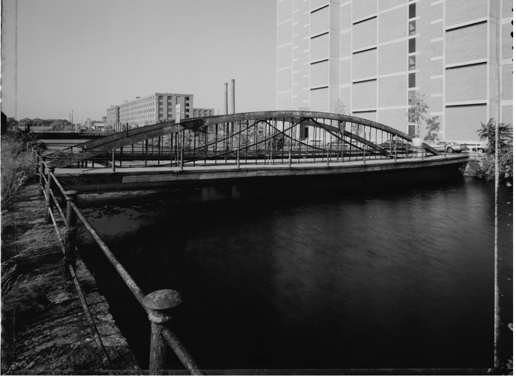
Figure 1-5. Arched wrought iron bridge by Thomas Moseley. Upper Pacific Mills Bridge moved to Merrimack College, North Andover, MA (HAER MASS,5-,LAWR,6-).
