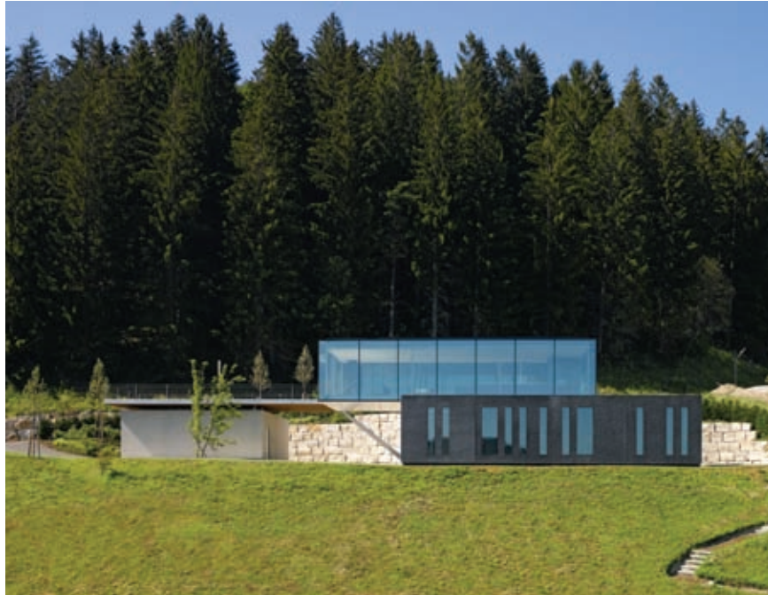
fig. 2 | House H16, Tieringen, Germany: This residential house for a family of four was envisioned as a completely transparent glass box.
