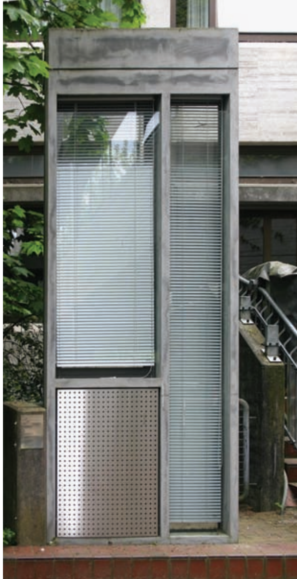
fig. 12 | A modular facade in fiber-reinforced concrete, a future field of application for this material
