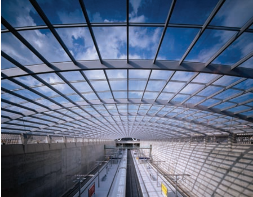
fig. 4 | ICE train station at the Cologne-Bonn Airport, Germany: Through extremely refined structural analyses, an enormous roof is supported by a minimal amount of metal.
