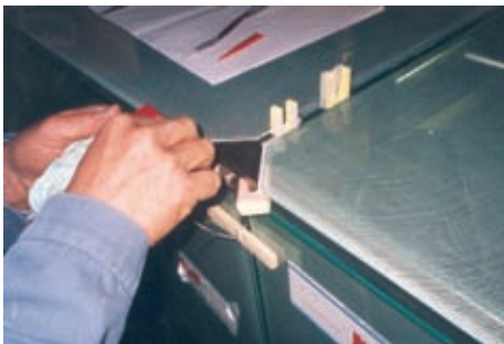
fig. 14 | Inserting the epoxy mortar
