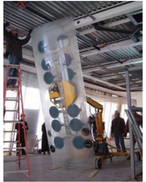
Installation of glass panel
