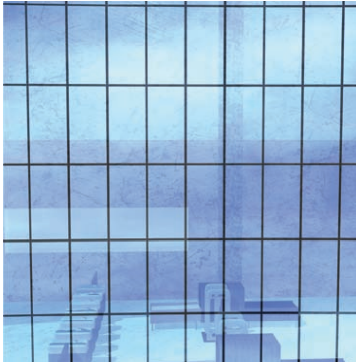
fig. 2 | Blast-resistant curtain wall that is engineered to take advantage of inherent flexibility and to withstand maximum loads transferred by the glazing
