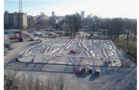
Bare roof structure during construction
