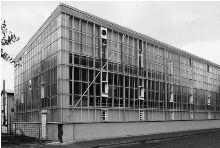
fig. 3 | Experimental curtain wall, Richard Steiff, Giengen an der Brenz, Germany, 1903
