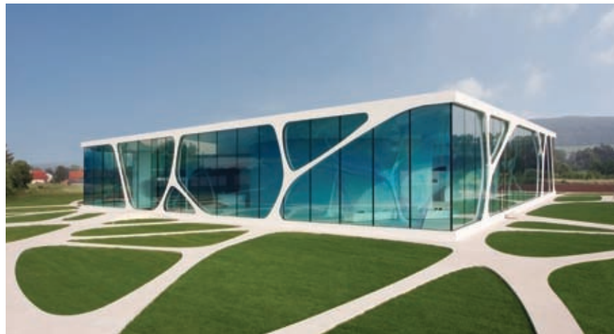
fig. 10 | Facade composed of 16 IGUs measuring 6 x 36 feet per side
