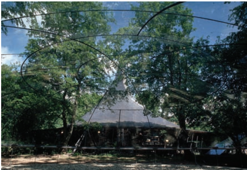
fig. 9 | Glued glass cupola, Stuttgart, Germany: Almost like building with paper, this laminated glass cupola has a clear span of 8.5 meters and a total thickness of 10 millimetres (1/10 the thickness of an eggshell).
