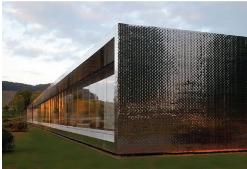
fig. 3 | SWM office building, Heilbronn, Germany: At the headquarters of the German steel industry, transparency is achieved through a facade composed of woven stainless steel struts.
