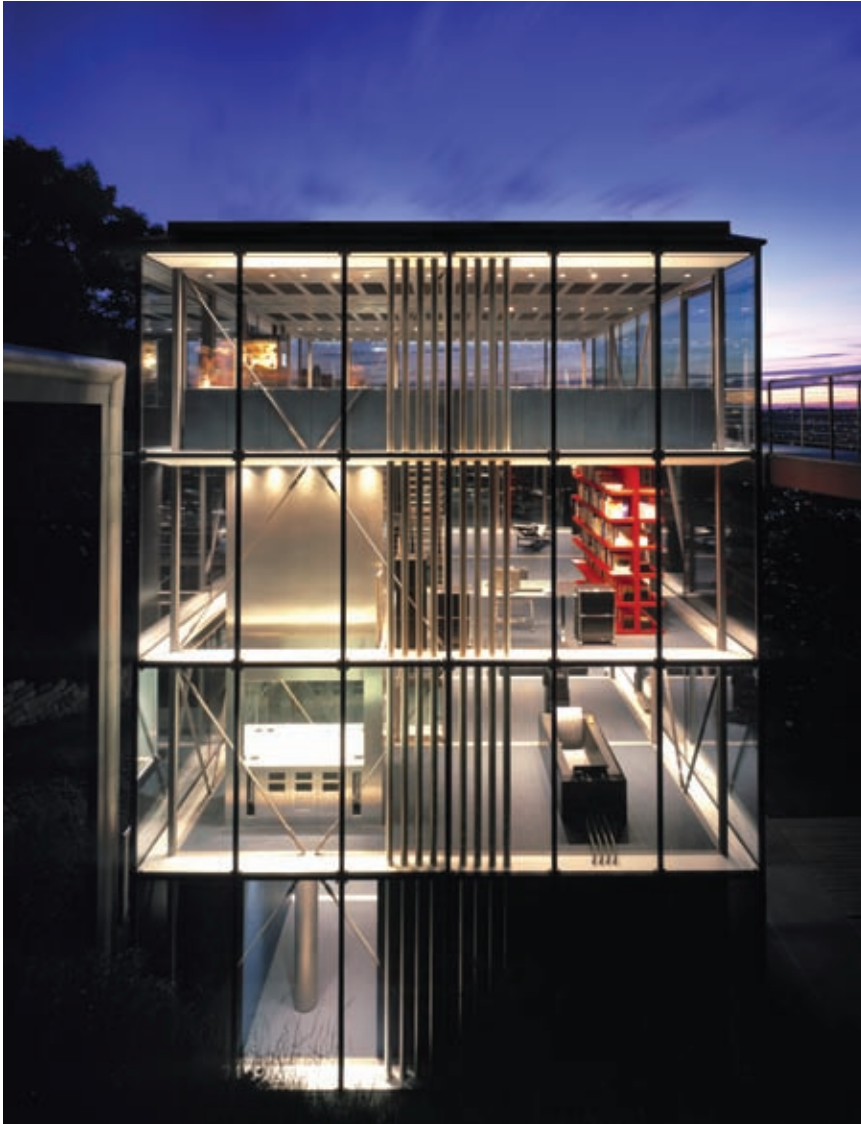
fig. 1 | R128 House, east elevation at dusk, Stuttgart, Germany: The basic idea of the house is to live in a soap bubble, surrounded by trees, fresh air, and with rain dripping down the walls. The building is completely recyclable and runs on solar energy. There are no chimneys or exhausts.
