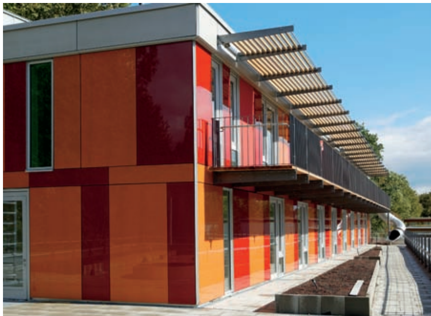
fig. 3 | A colorful facade composed of back-painted glass elements
