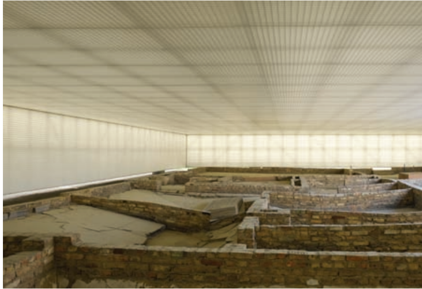
fig. 10 | Station Z, roof structure over the remains of the concentration camp in Sachsenhausen, Germany. With architect H.G. Merz, the decision was made to produce an architecture so modest that it virtually disappears. The building is stabilized by a vacuum, resulting in a long-span steel structure covering approximately 2,000 square meters of column-free space. Fabric is vacuum-sealed around a spatial truss using a tiny pump and a few square meters of photovoltaics. Vacuumatics are potential alternatives to pressurized air-inflated structures because they allow for reduced heat transfer while producing a homogenous surface that is free of details and can easily decompose or be recycled.
