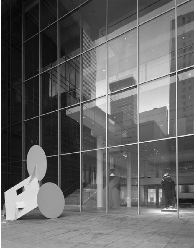
fig. 4 | Self-supporting wall with solid-steel mullions spanning sixty feet vertically, view from the sculpture garden at the Museum of Modern Art, New York, N.Y.
