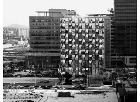
fig. 9 | Construction view of Trutec, Seoul, Korea, Barkow Leibinger with Schlaich Bergemann, 2007
