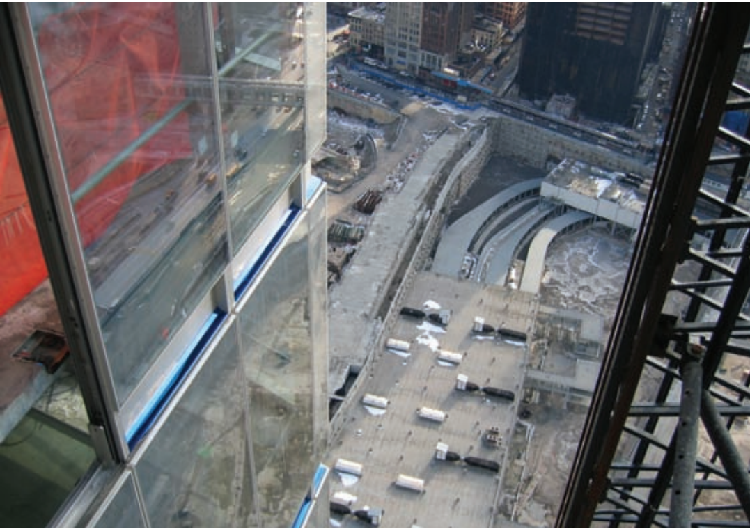
View of the curtain wall during installation
