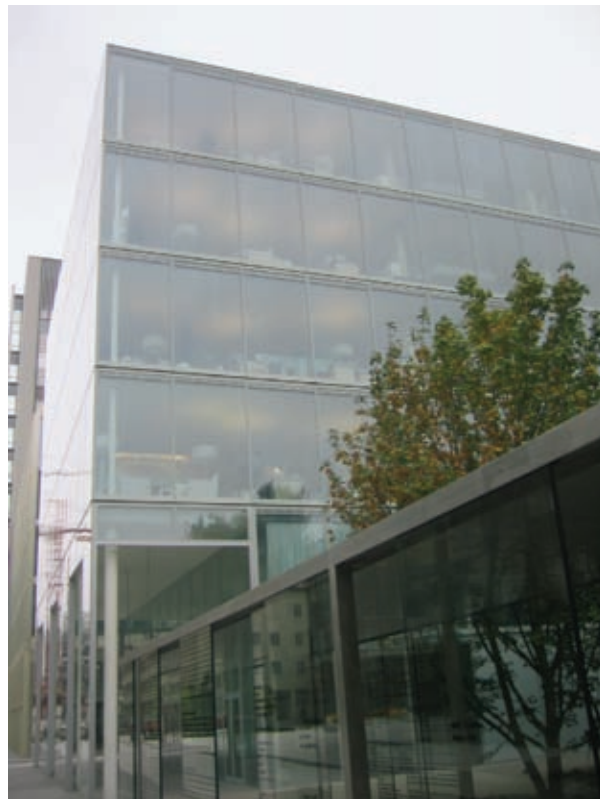
fig. 4 | View of variegated glazing, Novartis Office Building, SANAA
