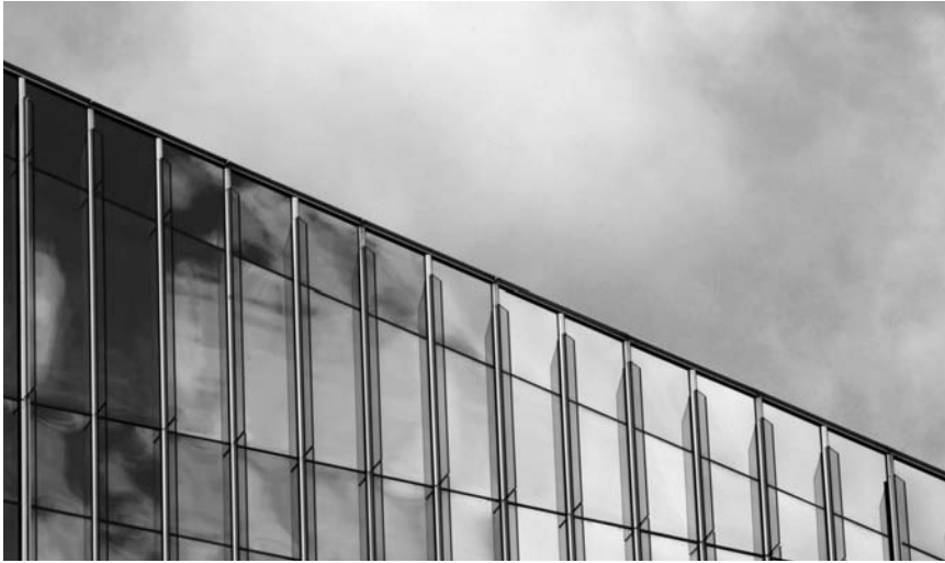
fig. 1 | Facade detail, Gannett/USA Today Corporate Headquarters, Kohn Pederson Fox and R.A. Heintges and Associates, McLean, Va., 2003
