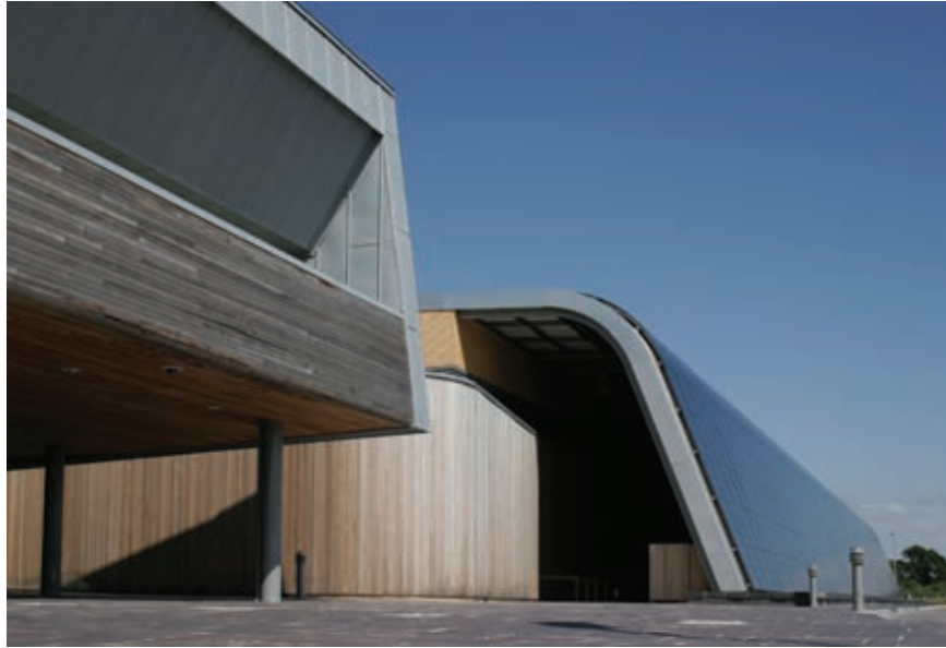
fig. 2 | Integrated CIS thin-film modules curve from the top of the roof to a water harvesting pool, OpTIC Centre, St. Asaph, North Wales, United Kingdom
