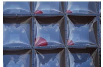
fig. 6 | Proposed sun-shading devices for facade constructions
