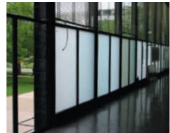
fig. 10 | interior, existing conditions
