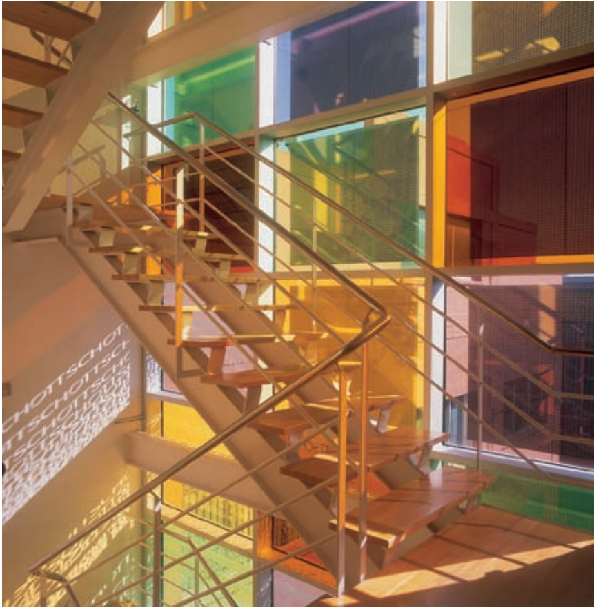
fig. 4 | The interior of double-glazed windows containing thin-layer modules of colored amorphous silicon
