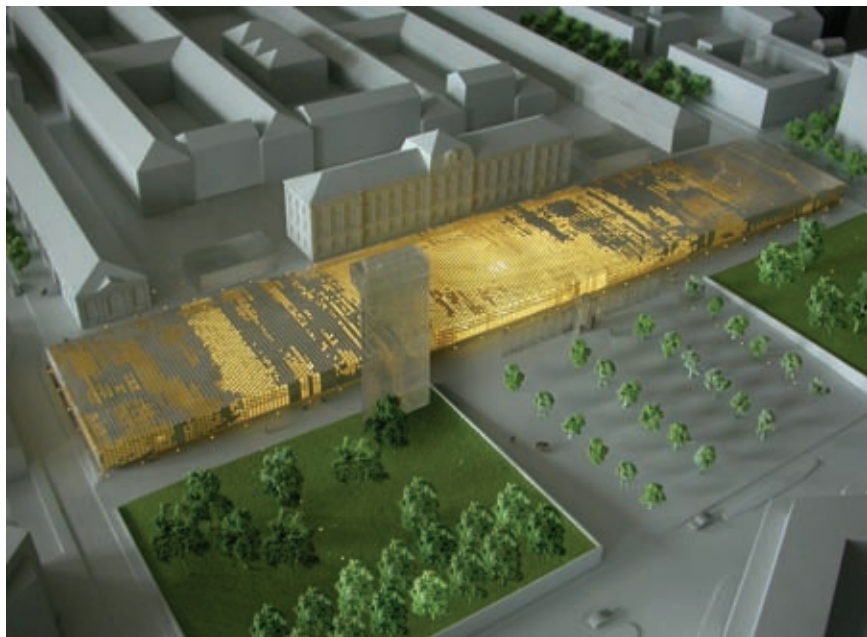
fig. 7 | Cité du Design, St. Etienne, France: Designed by Finn Geipel, the skin is a combination facade and roof composed of 14,000 triangular elements grouped according to function. Some provide heat insulation, others transmit light or produce energy.
