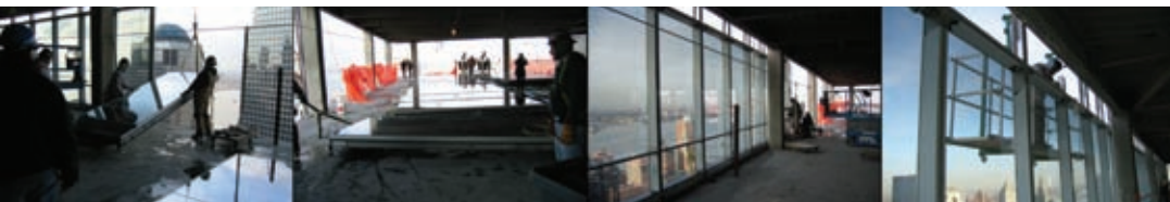
Sequence of photographs showing the installation process of the curtain-wall panels
