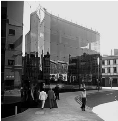
fig. 2 | Willis Faber and Dumas, Norman Foster and Associates, Ipswich, England, 1975
