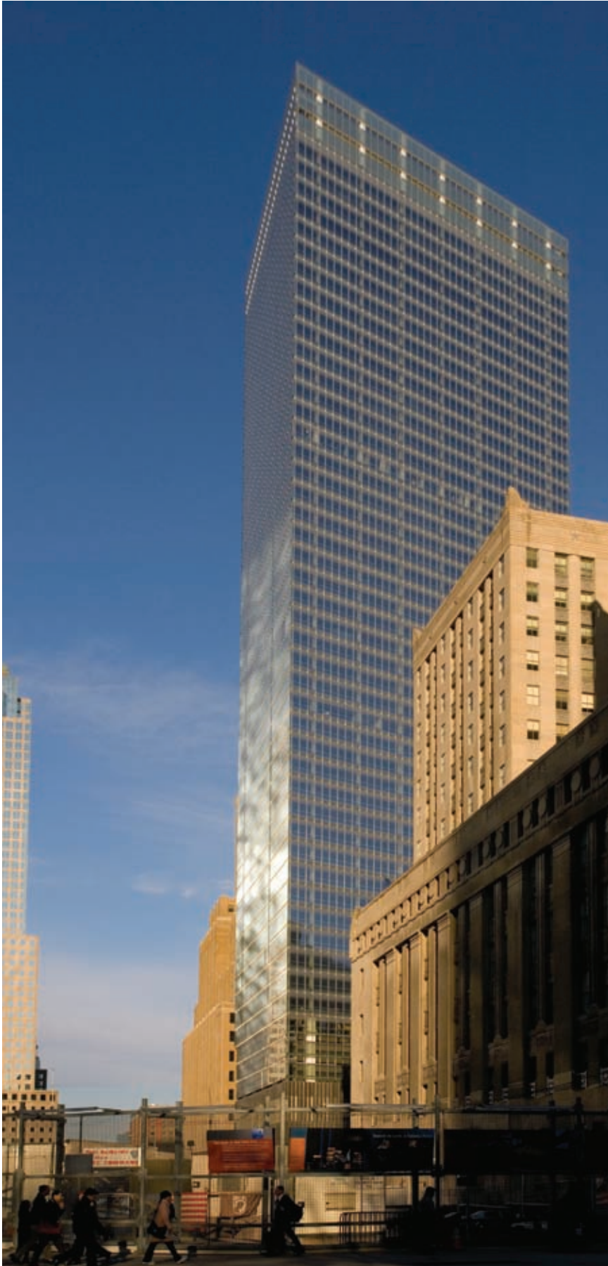
The curtain wall combines low-iron glass with a reflective coating, allowing light to enter the tower and reflecting it into the public realm.
