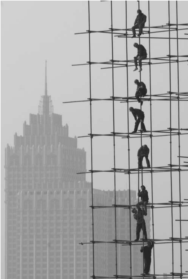
Figure 4.6 Workers on scaffolding in Shenyang, China, 2009.
