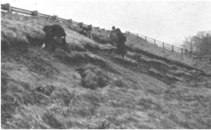
Figure 4.4 Shallow slides near Reading, Berks. The failure plane is clearly visible.
