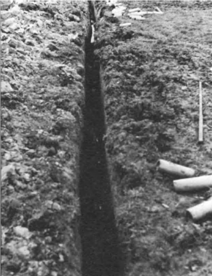
Figure 3.18 Tile drainage in progress.
