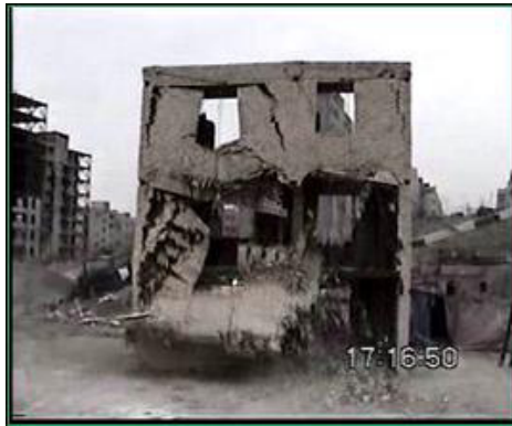
Figure 2: The demolishing masonry building.
