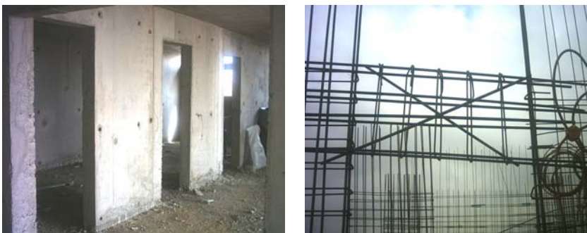
Figure 2: Typical deep coupling beams above the door opening and diagonal reinforcement without confining ties in a tunnel form building.
