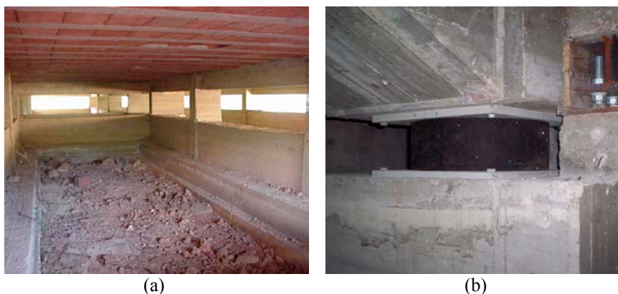
Figure 19: Squat columns in the original building before (a) and after (b) the insertion of the seismic isolators (After Calìo and Marletta [28]).
