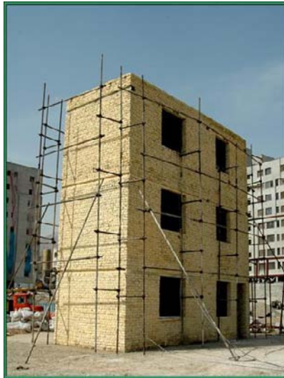
Figure 1: The three storey masonry building.
