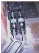
Figure 21: Left: some of the 47 SMADs installed in the Upper Basilica of St. Francis at Assisi in 1998-99, during its restoration after the damages caused by the 1997-98 Umbria and Marche earthquake, to connect both tympana to the transept roof. Centre and right: two of the 34 STs installed inside the Upper Basilica, during the aforesaid restoration, to stiffen it.
