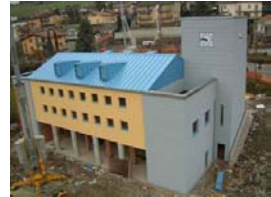
Figure 17: The new Civic Room / Red Cross Headquarters of Gaggio Montano (Bologna, seismic zone 3), quite an irregular structure that was seismically isolated by means of 33 HDRBs and 4 SDs in 2006.
