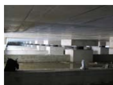
Figure 30: The “La Luz” new hospital at Lisbon (Portugal), which was seismically isolated, together with a residence for old people in 2006; view of some of the 315 HDRBs installed at the buildings base, which were manufactured in Italy.
