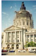
Figure 11: San Francisco City Hall, erected in 1912, which was damaged by the 1989 Loma Prieta earthquake and was seismically retrofitted with 530 LRBs and 62 SDs in 2000.
