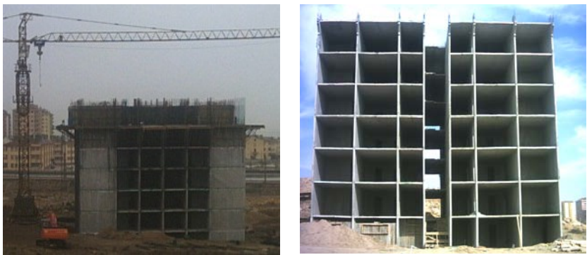
Figure 1: Typical tunnel form systems at construction stage.
