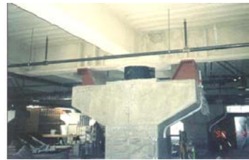
Figure 12: The new 911 Emergency Communications Centre at San Francisco, protected by HDRBs in the years '90s so as to remain fully functional to 8.3 magnitude. This is the design earthquake level for all strategic buildings in California. In any case, also the existing public buildings shall be retrofitted so as to withstand very large quakes (e.g. of 8.0 magnitude). This imposes the use of SI, in spite of its large cost in the USA.
