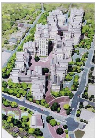
Figure 3: Sketch of the complex of twenty one 6- to 14-storey buildings, all erected on an isolated artificial ground at Sagamihara (Tokyo area) with LRBs, Sliding Devices (SDs) and Ball Bearings.
