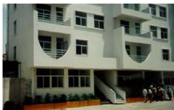
Figure 7: R.c. dwelling building at Shantou that was the first Chinese application of HDRBs (1991). It withstood a significant earthquake with no damage in 1994.
