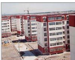
Figure 8: The complex of 60 new masonry dwelling buildings that was erected in Western China with HDRBs in 1996.
