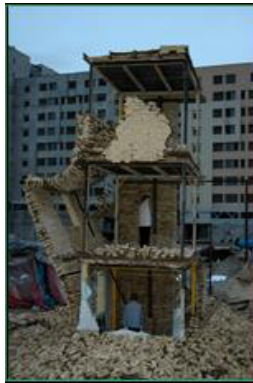
Figure 3: Operation of the safe rooms after collapsing the load bearing walls.
