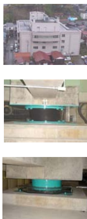
Figure 1: Ojiya City building that withstood the 2004 Mid Niigata quake without any damage; its rubber bearings and SDs.
