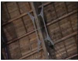
Figure 22: The Cathedral of Santa Maria di Collemaggio at L'Aquila, a unique example of Romanic style in Abruzzo, and view of one of the elastic-plastic dampers (EPDs) installed in its roof after the walls had vibrated during the 1997-98 Marche and Umbria earthquake, in spite of the very large distance from the epicentre.
