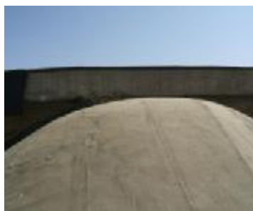
(a) the solid concrete tie-beam
