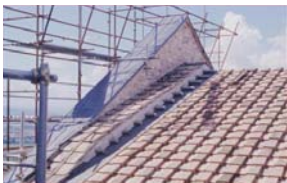
Figure 21: Left: some of the 47 SMADs installed in the Upper Basilica of St. Francis at Assisi in 1998-99, during its restoration after the damages caused by the 1997-98 Umbria and Marche earthquake, to connect both tympana to the transept roof. Centre and right: two of the 34 STs installed inside the Upper Basilica, during the aforesaid restoration, to stiffen it.
