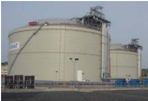
Figure 31: The two 140,000 m 3 LNG tanks of Egegaz at Aliaga, Turkey, protected by 112 LRBs and 241 LDRBs.
