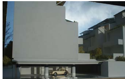
Figure 19: Plastic model of 6 dwelling buildings to be erected on the same artificial ground slab supported by 40 HDRBs and 12 SDs in the framework of the demolition / reconstruction project of the present very degraded Pontecitra 11-buildings complex at Marigliano (Naples). Erection of over 60 buildings on 16 slabs, supported 400–450 HDRBs and 360–380 SDs, has been planned.
