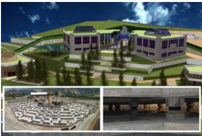
Figure 18: Plastic model of the two buildings of the new Francesco Jovine school being reconstructed at San Giuliano di Puglia, Campobasso (supported by an unique isolated slab), after the collapse of the previous primary school during the 2002 Molise and Puglia earthquake, and view of its SI system, formed by 61 HDRBs and 12 SDs, during construction in 2006-2007.
