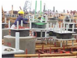
Figure 32: The two 160,000 m 3 LNG tanks at Guandong (P.R. China), each with 360 HDRBs in 2006.
