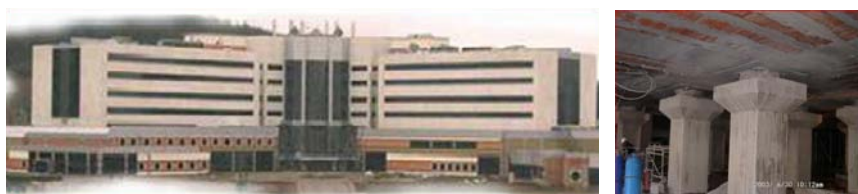
Figure 28: The Kocaeli University Hospital (Turkey), which was seismically isolated with the Friction Pendulum System (FPS) in 2006.
