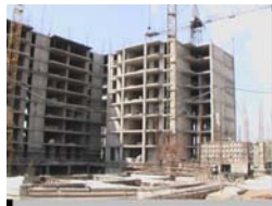
Figure 27: The 16-storey "Our Yard" multifunctional complex, seismically isolated by means of Increased Damping Neoprene Bearings, during its construction at Yerevan (Armenia) in 2006.
