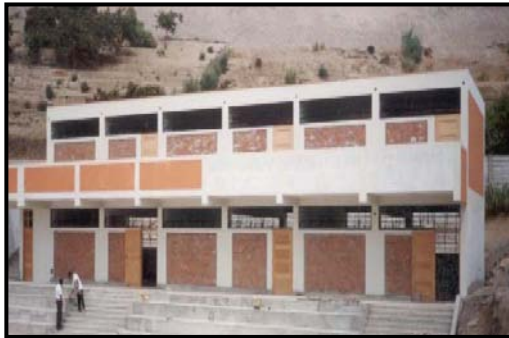
Figure 3: 780 pre Seismic Design 1997 Code buildings.
