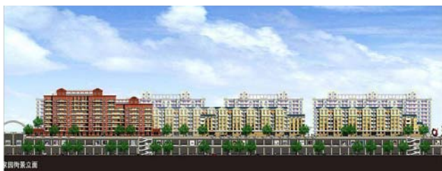
Figure 9: The “Isolation House Building on Subway Hub”, the new residential centre of Peking formed by 50 7–9-storey buildings ( 480,000\text{ m}^2 ) supported by a unique 2-storey ( 1500\text{ m} \times 2000\text{ m} ), containing all facilities and been isolated by means of HDRBs.
