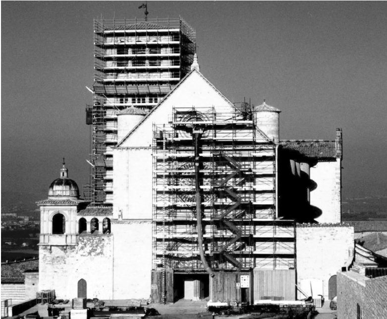
Figure 8.19 The Basilica of St Francis of Assisi after the 1997 Umbria–Marche earthquake, exterior view. The tower and the tympanum to the south transept sustained repairable damage. The temporary works on the east façade are to provide access to the roof space for repair of the vaulting
