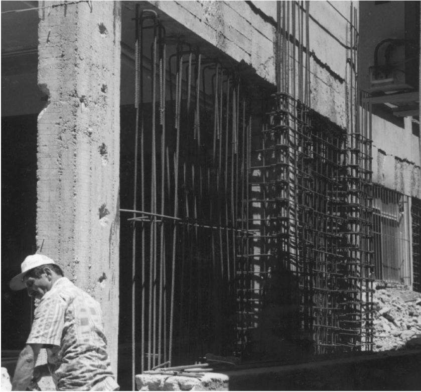
Figure 8.16 Strengthening existing reinforced concrete buildings – adding reinforced concrete shear walls in Bolu, Turkey, following minor damage in the 1999 Kocaeli earthquake
