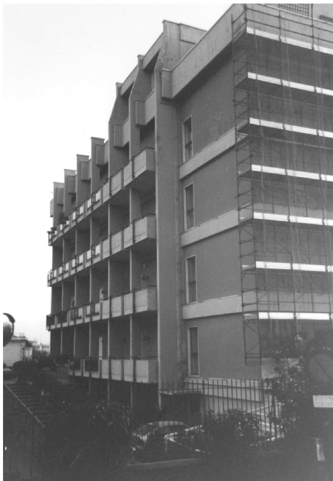
Figure 8.17 Retrofitting of reinforced concrete frame buildings: adding shear walls by external buttressing reduces the impact on the internal organisation of the building and may reduce the time during which the building needs to be empty. Residential reinforced concrete block in Naples, Italy
