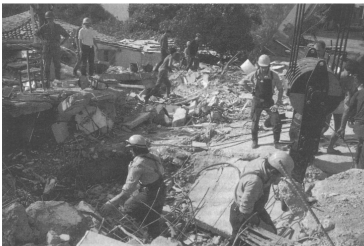
Figure 4.5 Search for victims buried in collapsed structures can continue for many days. Search and rescue activities in the collapse of a reinforced concrete framed apartment building, 1986 Kalamata earthquake, Greece. (Reproduced by permission of A. Pomonis)
