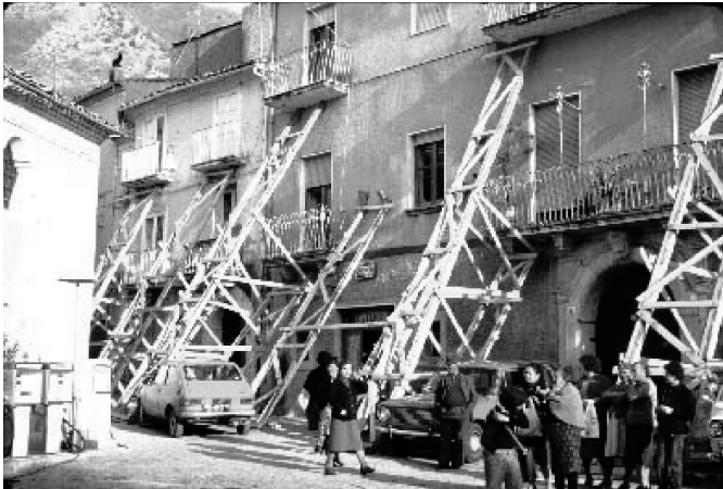
Figure 4.14 Use of timber to prop unstable masonry. Aftershocks may continue for several weeks, and propping of the façades of damaged masonry buildings is essential to maintain safety for the public. Propping in Bagnoli Irpino, after the 1980 Irpinia earthquake in southern Italy
