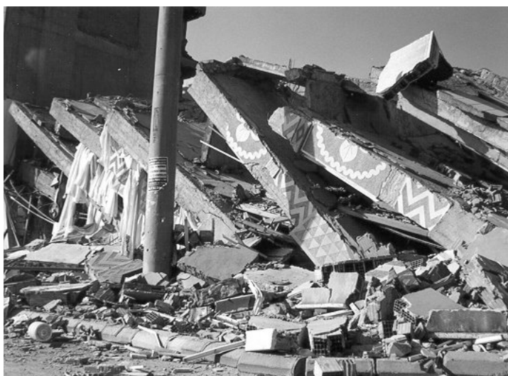
Figure 1.8(f) EMS damage state D5 (destruction)
