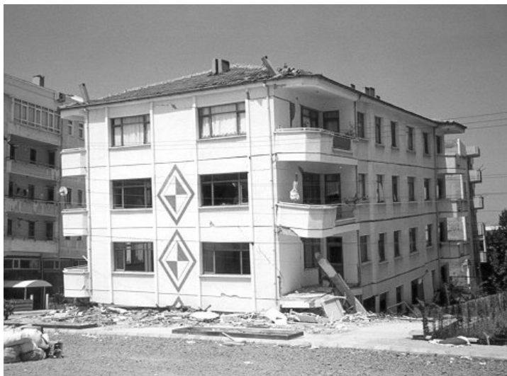
Figure 1.8(e) EMS damage state D4 (very heavy damage/partial collapse)
