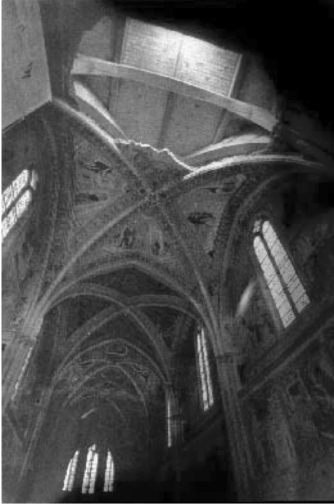
Figure 8.20 The Basilica of St Francis of Assisi after the 1997 Umbria–Marche earthquake, interior view. One of the two collapsed sections of the vaulting, containing early Renaissance frescoes of great importance to the history of art, showing the twentieth-century reinforced concrete supports for the roofing which may have contributed to the vault failure (Spence 1998). The vaulting was reconstructed with additional external supports (Crocì 1998), and the Basilica was reopened in 2000
