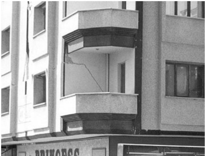
Figure 1.8(c) EMS damage state D2 (moderate damage)
