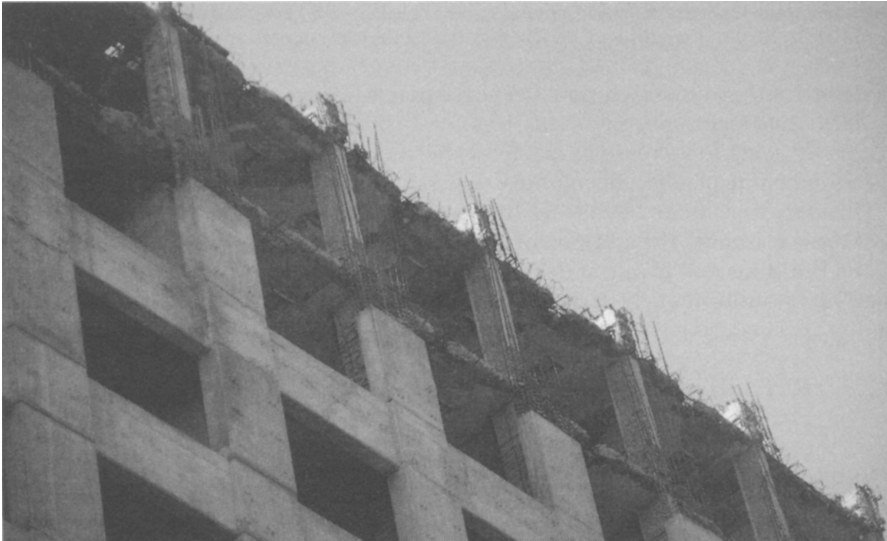
Figure 8.18 Strengthening a reinforced-concrete-framed building can be achieved by encasing the old frame within a new structure. Shear wall structure being cast around a frame to upgrade the earthquake resistance of the Tribunal Law Court building in Mexico City
