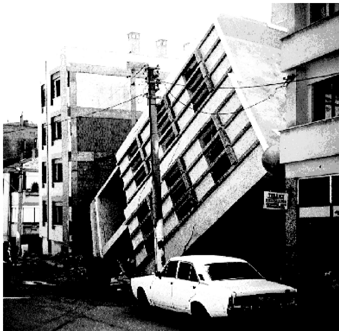
Figure 7.1 Building failure caused by liquefaction. This recently completed building in Adapazari, Turkey, overturned when the soil below its shallow foundations liquefied in the 1999 Kocaeli earthquake. The building, otherwise little damaged, is nevertheless a complete loss
