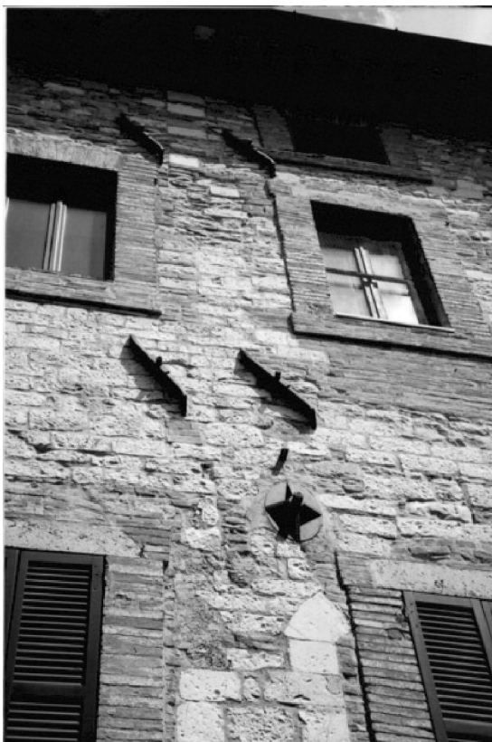
Figure 8.22 Addition of tie rods is an effective and relatively low-cost way to strengthen existing masonry buildings – buildings in Assisi, Italy, strengthened following the 1997 Umbria–Marche earthquake
