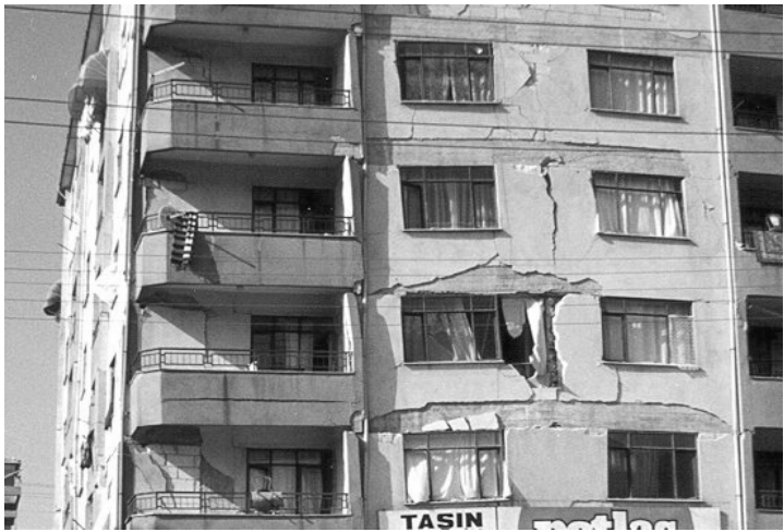
Figure 1.8(d) EMS damage state D3 (heavy damage)
