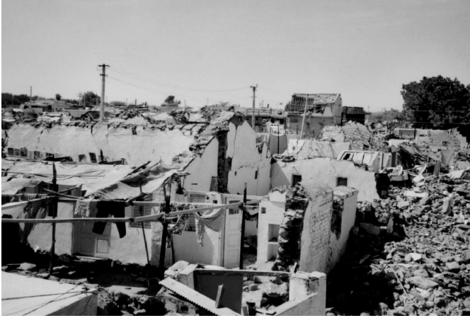
Figure 8.8 Destruction of rubble stone masonry in Bhuji, in the 2001 earthquake. Buildings of this type have been found to be highly vulnerable to earthquake damage in many countries
