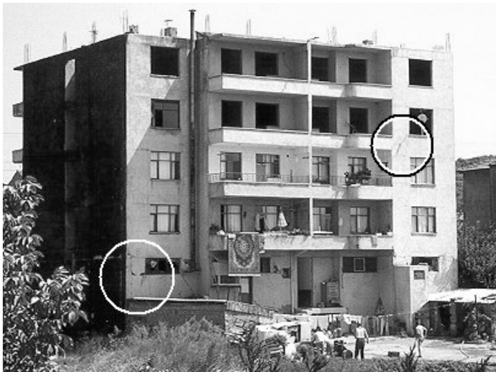
Figure 1.8(b) EMS damage state D1 (slight damage)
