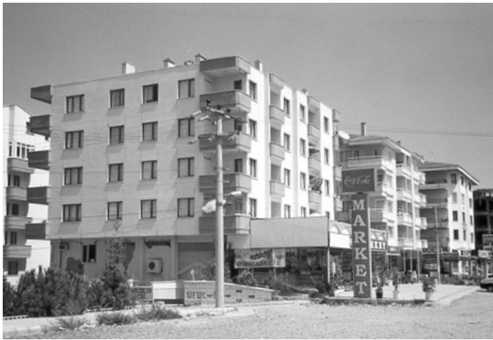
Figure 1.8(a) EMS damage state D0 (undamaged)
