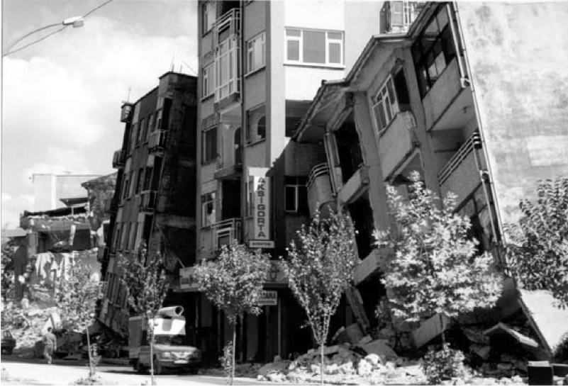
Figure 8.6 Collapse of reinforced concrete buildings in Adapazari, Turkey, in the 1999 Kocaeli earthquake
