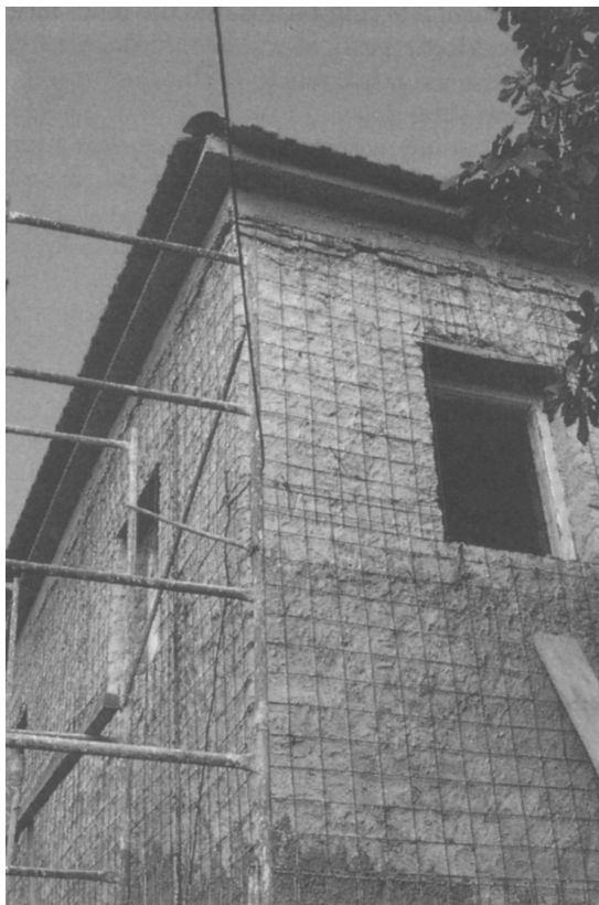
Figure 8.15 An external and internal skin of wire mesh and cement render is a common method of reinforcing old or damaged masonry. Reconstruction after the 1982 Corinth earthquake, Greece
