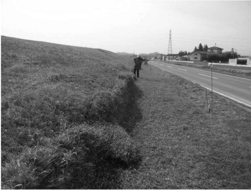
Figure 4. Naruse River, R12.0k (River division, NILM). The levee spread laterally on the surface of foundation soil toward hinterland side. There was not any detected deformation outside the levee toe.
