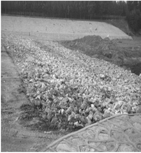
Figure 11. Reinforcement of Bashan reservoir dam.
