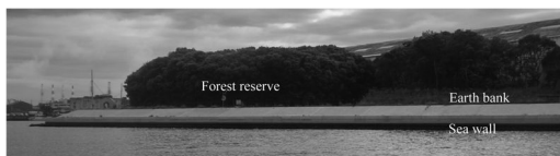
Photo 11. Concrete example of design concept combining sea wall with earth bank planted at Osaka Bay Area.
