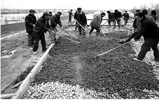
Figure 10. Installation of composite soft geomembrane mattress at Xinjiawan of Anhui Province.
