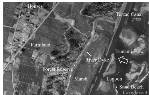
Photo 1. Aerial view around the river dyke damaged slightly at Idoura in Sendai City.
