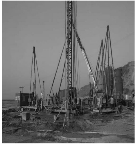
Figure 13. Reinforcement of Xiakou dam using vibro replacement stone column method.
