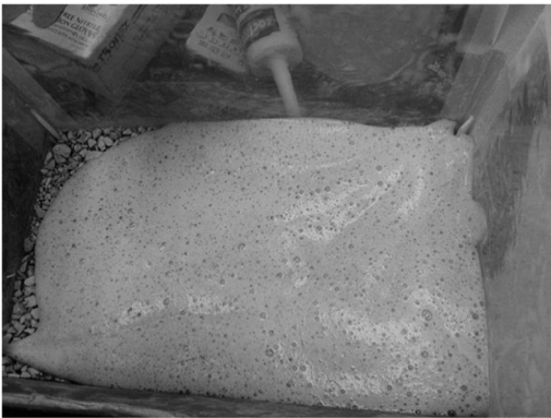
Figure 16. Applying the biogrout directly on top of base and subbase of the road.
