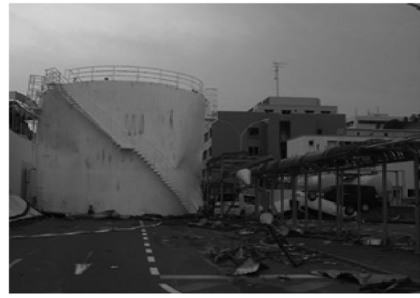
Figure 8. Heavy fuel oil tank swept up by the tsunami and blocking the road (Diameter: 11.7 m Height: 9.2 m).
