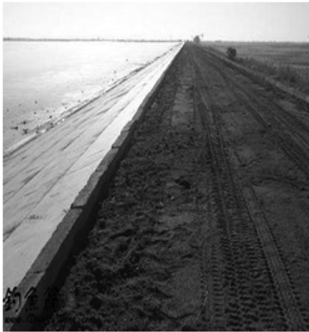
Figure 12. Reinforcement of Qingan reservoir dam.
