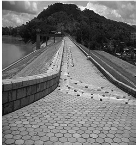
Figure 14. Reinforcement of Donger reservoir using vibro replacement stone column method.
