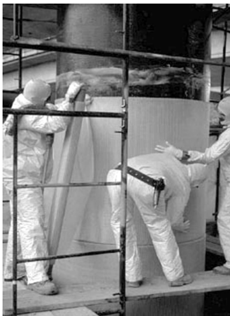
2.4 Use of wet layup for installation of a fiber-reinforced polymer jacket for seismic retrofit of columns.
