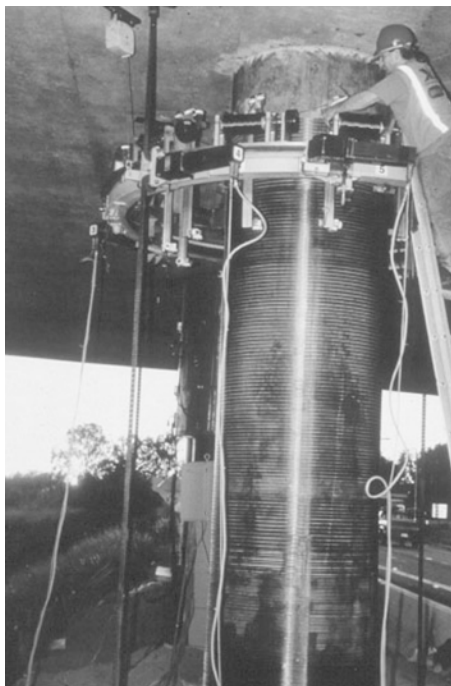
2.6 Automated winding of prepreg tow for seismic retrofit of columns.
