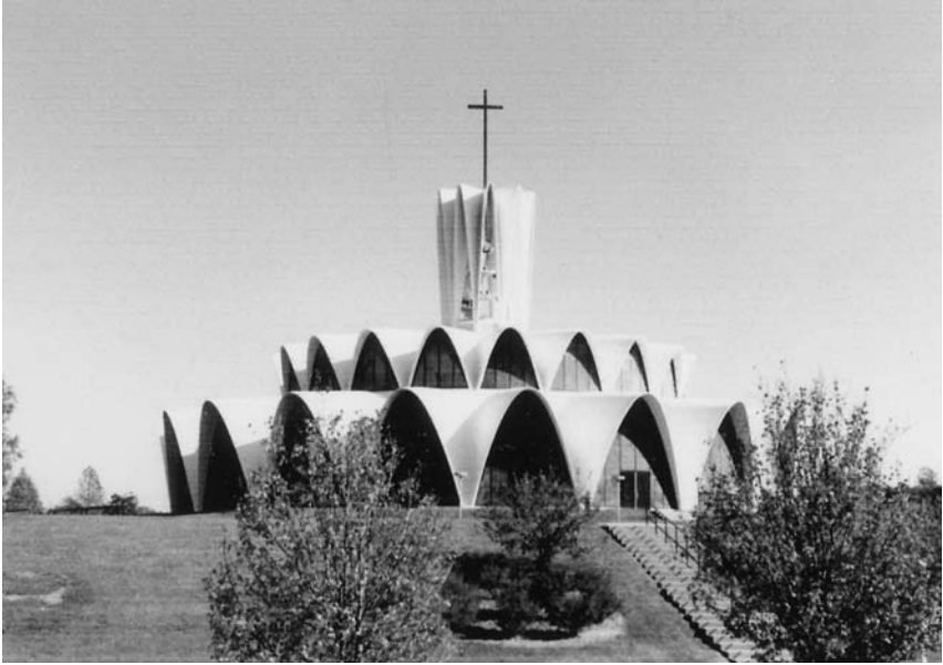
Figure 8. St. Louis Priory, designed by Gyo Obata and made of parabolic shells of reinforced concrete and fiberglass walls, 1962. (St. Louis Priory)
