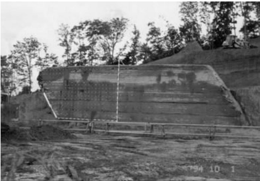
Fig. 7.4 Removing the fill supporting the overhanging cliff (Step 2)
