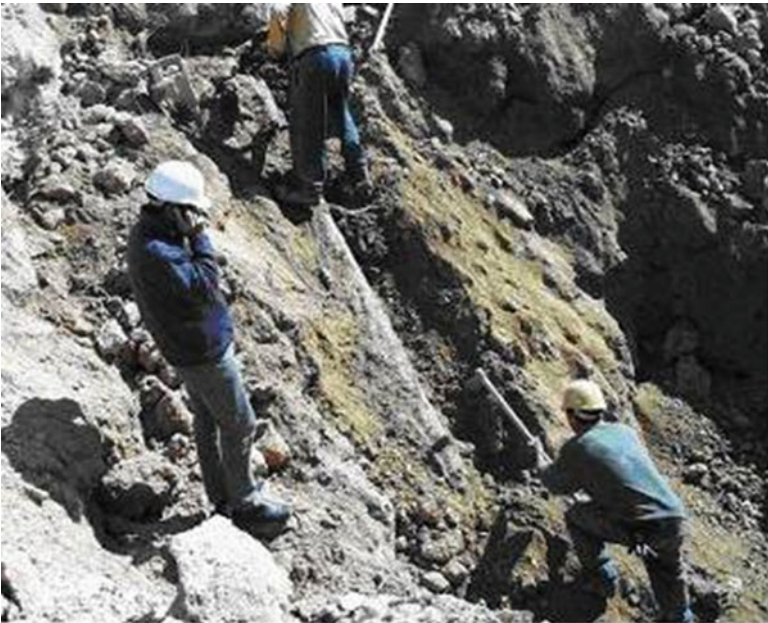
Fig. 17.24 Close view of anchor excavation
