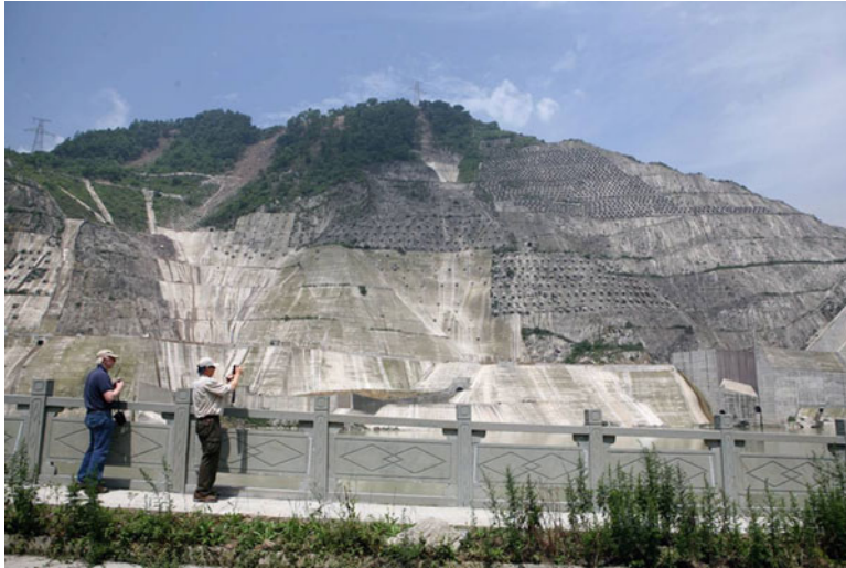
Fig. 5.12 The right bank slope at the Zipingpu dam site
