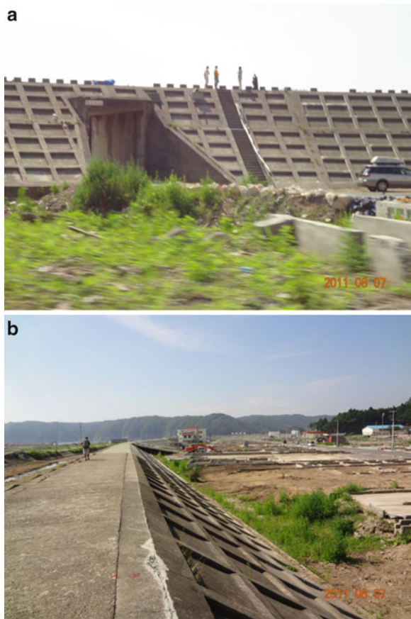
Fig. 1.5 Areas heavily protected by seawalls. (a) Huge seawall at Taro, Miyako. (b) Inland area behind the seawall at Taro
