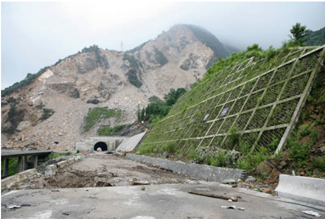
Fig. 5.8 Behavior of anchored concrete frame along the Dujiangyan-Yingxiu expressway
