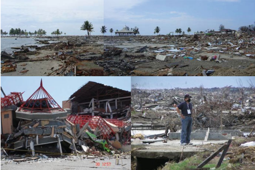
Fig. 3.4 The damages of buildings and facilities due to the 2004 Aceh Earthquake
