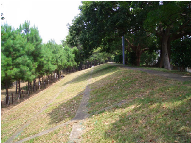
Fig. 1.6 Protective seawall embankment at Hiro
