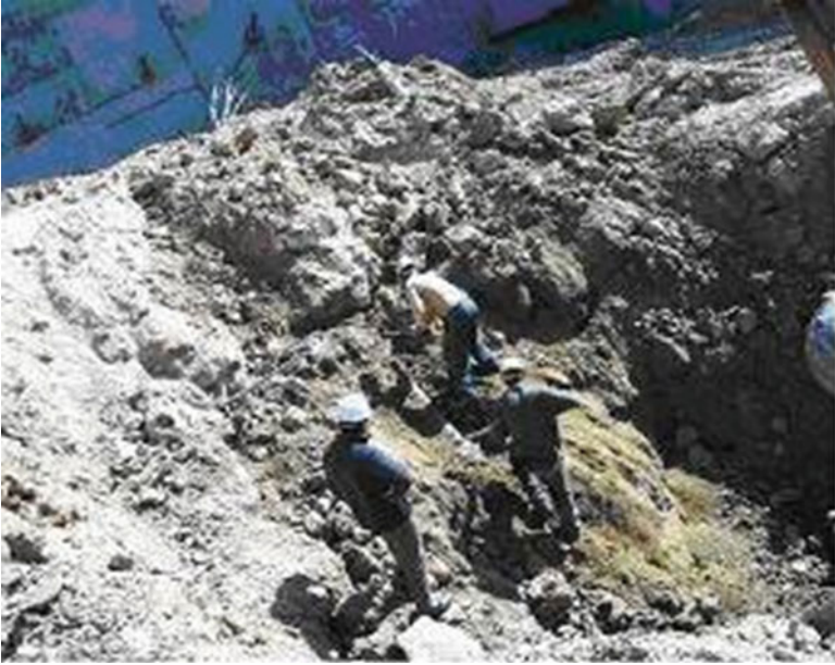
Fig. 17.23 Anchor excavation
