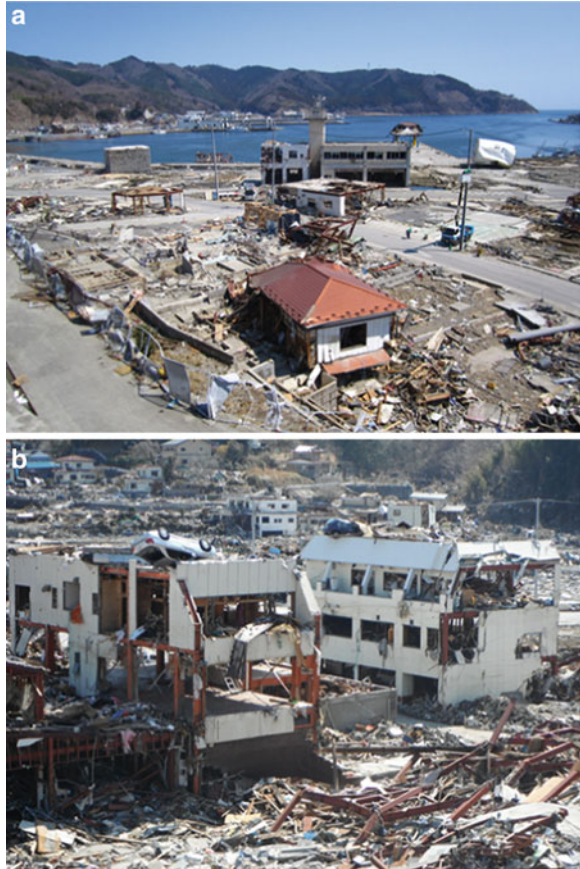
Fig. 1.3 Onagawa immediately after suffering from the tsunami disaster. (a) Onagawa harbor completely washed out. (b) Cars on top of two buildings
