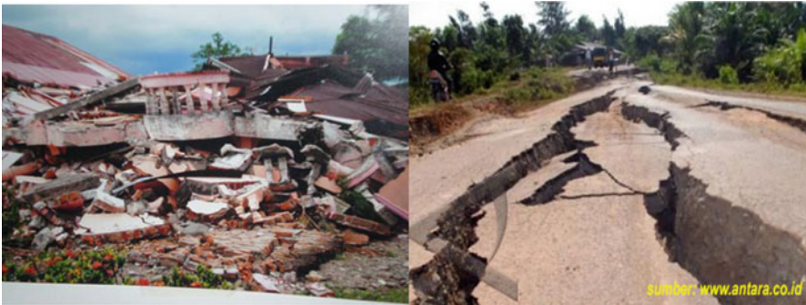
Fig. 3.5 Buildings failures and ground cracking due to the 2007 West Sumatera Earthquake (Source: Bappenas 2007)
