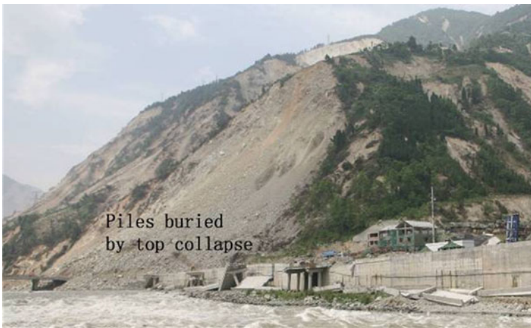
Fig. 5.11 Buried piles in Yingxiu town along the Dujiangyan-Yingxiu expressway
