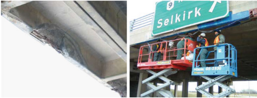
Fig. 7.30 Bridge girder strengthening, Winnipeg (Canada), courtesy of Prof. Dr. Y. Kim
