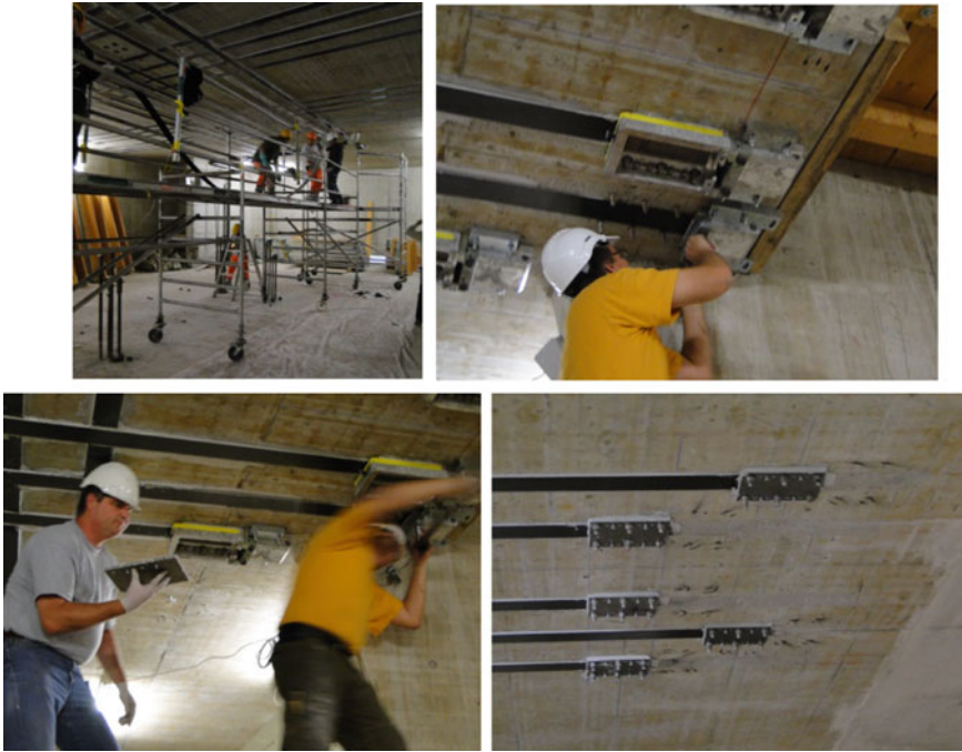
Fig. 7.27 Office building, Zurich Altstetten (Switzerland), courtesy of S&P Clever Reinforcement AG
