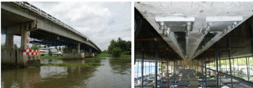
Fig. 7.26 Bridge girder strengthening, Bangkok (Thailand), courtesy of S&P Clever Reinforcement AG
