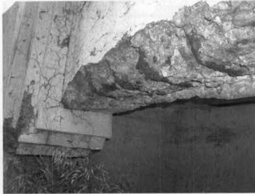
Figure 4.1 A severely deteriorated reinforced concrete bridge girder in Ontario; the deterioration is due to corrosion and the freeze and thaw effect.
