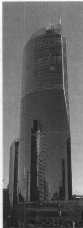
Figure 13.15 A view of the One Wall Centre building in Vancouver, British Columbia.
