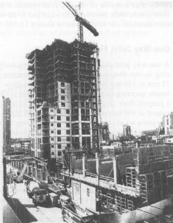
Figure 11.2 A concrete high-rise under construction uses a flyform table system.
