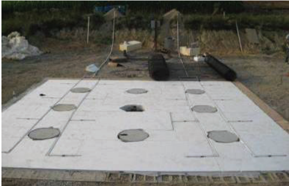
FIG. 8. CSE test facility with geofoam and geofoam dissolver delivery system.
