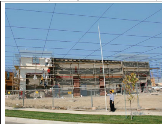
Fig.15: 200-Year WSL in South Natomas Basin (Figure courtesy of the Calif. Dept. of Water Resources)
