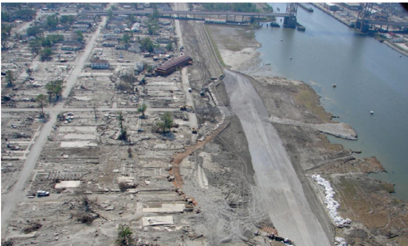
Fig. 5: Massive South Breach at the Lower Ninth Ward (Seed et al., 2008b)
