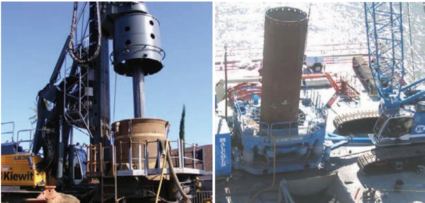
a) Drill-Mounted Oscillator
