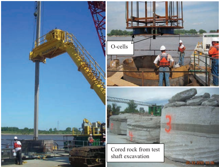
FIG. 20. Load Test Shaft for the Mississippi River Bridge, St. Louis.
