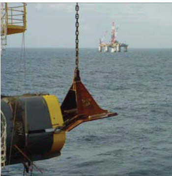
(a) Inserting SEPLA in caisson
