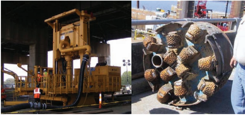
a) Restricted Headroom Drilling
