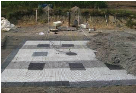
FIG. 9. Reinforced fill placement.
