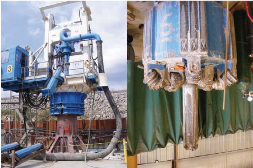
FIG. 15. Reverse Circulation Drilling for Secant Pile Cutoff Wall
