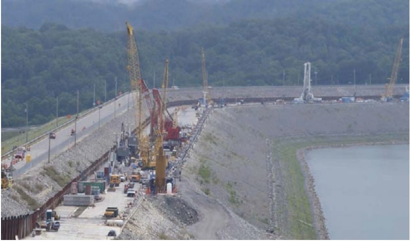
FIG. 15. Work Platform at Wolf Creek Dam.
