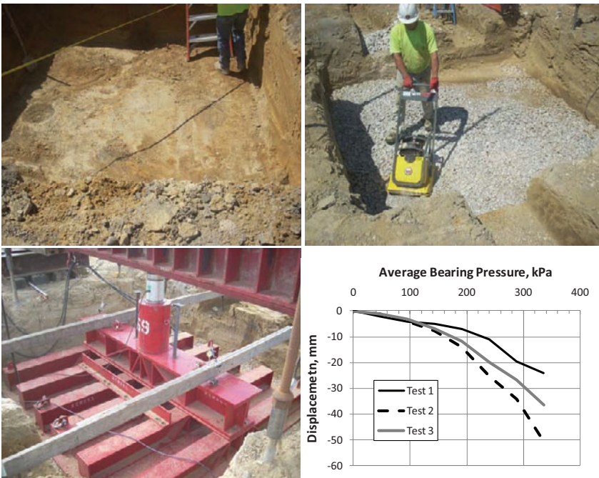
FIG. 11. Load Tests of Drilled Displacement Columns Supporting a Conventional Spread Foundation.
