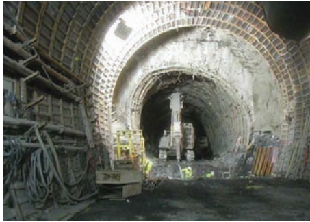
FIG. 9. Re-profiling of a highly deformed cross section is taking place in the Saint Martin access adit (Lyon-Turin Base Tunnel). After Barla et al. (2008).
