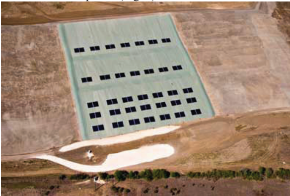
Fig. 2. Aerial view of the exposed geomembrane with arrays of solar panels at the Tessman Road Landfill (Roberts 2010)
