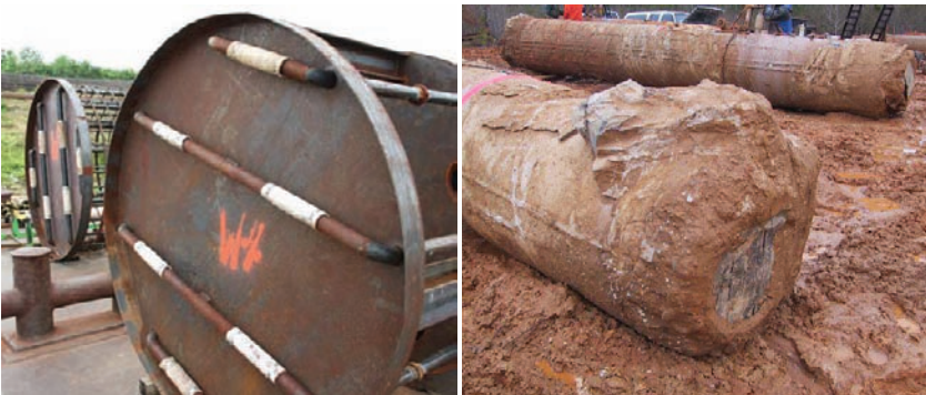
a) Sleeve Port System for Grouting
