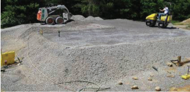
FIG. 10. Loader and vibrating roller used for fill placement and compaction.
