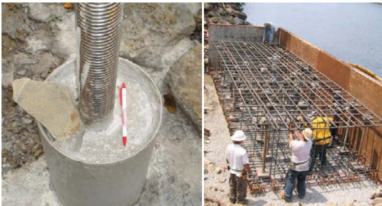
FIG. 4. Completed Micropile and Connection to Footing.
