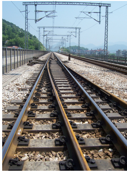
FIGURE 10.15 CWR turnout on bridge in Zhejiang–Jiangxi line.
