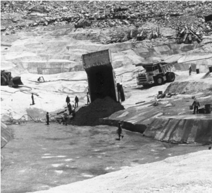
Figure 17.4. Dental concrete at Kenyir Dam (Courtesy of Snowy Mountains Engineering Corporation).
