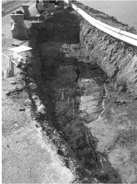
Figure 11.11. Cracking and softening due to settlement and lateral spreading at the crest of an embankment dam (courtesy Goulburn-Murray Water).
