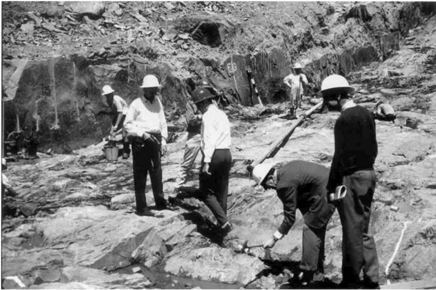
Figure 17.17. Tumut 2 concrete gravity dam foundation cleanup in progress.
