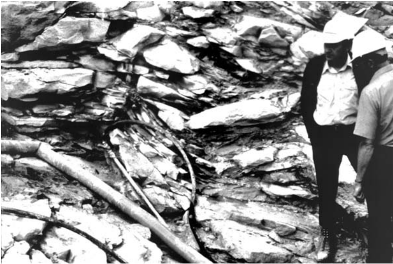
Figure 2.10. Crushed zone in Unit D (Interbedded siltstone and claystone) formed by overthrusting. Photograph courtesy G. McNally.
