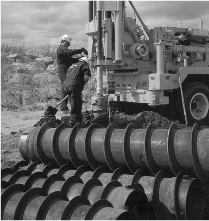
Figure 5.11. Large diameter hollow auger drill rig (courtesy CMEC).
