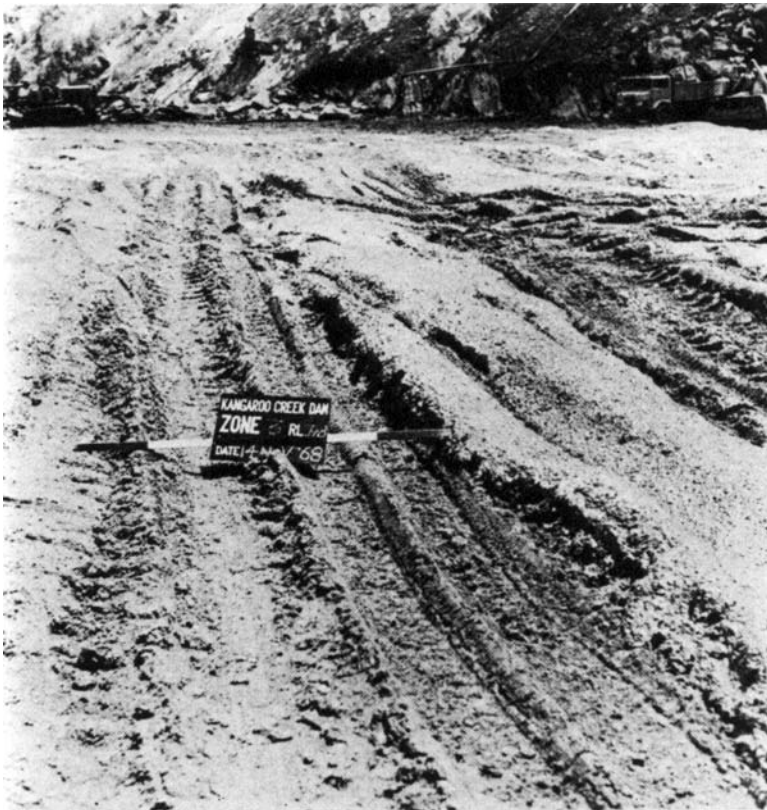
Figure 3.15. Slurry (Gravelly sandy silt) formed on the top of schist rockfill layer as a result of weathering and compaction by 4 passes of a 10-tonne vibrating roller (Trudinger, 1973).
