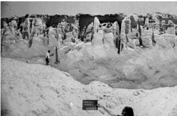
Figure 3.28. Weathering profile on very weak, porous calcarenite near Perth, Western Australia. Note the extremely irregular nature of the rock surface.
