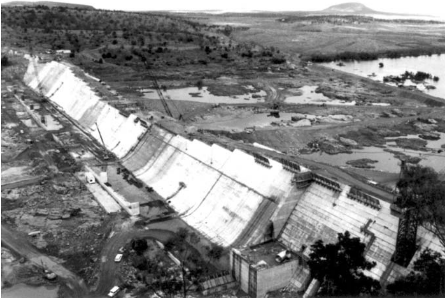
Figure 17.25. Burdekin Falls Dam, under construction, showing the 600 m. wide valley floor, formed by extremely strong, sheet-jointed rock. (Photo courtesy of Sun Water).
