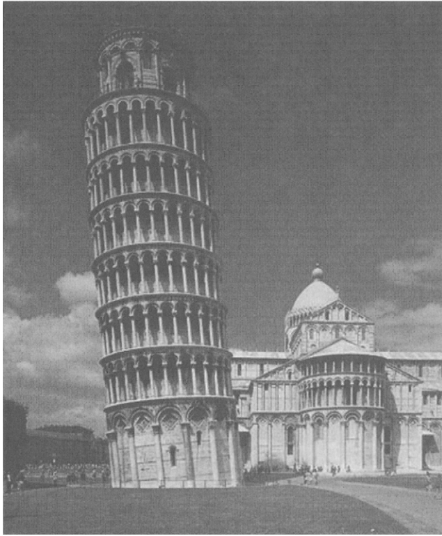
Figure 14.2 Tower of Pisa (clay consolidation)
