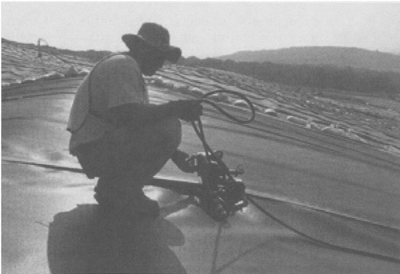
Figure 28.2 Geomembrane used for a landfill liner (Source: http://www.hallaton.com )
