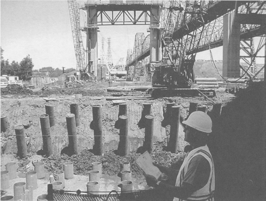
Figure 30.13 Pipe pile construction. (Source: http://www.dot.ca.gov )
