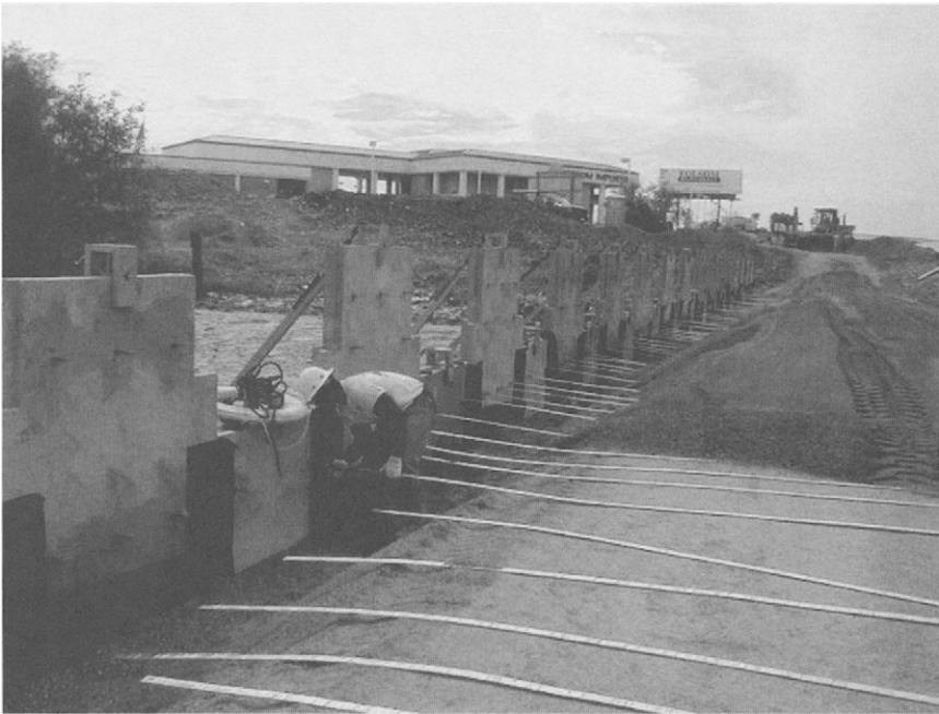
Figure 17.3 Construction of metal strips (Source: California DOT)
