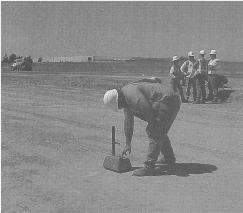
Figure 2.25 Checking the compaction status with a nuclear gauge Source: ( http://www.dot.ca.gov )
