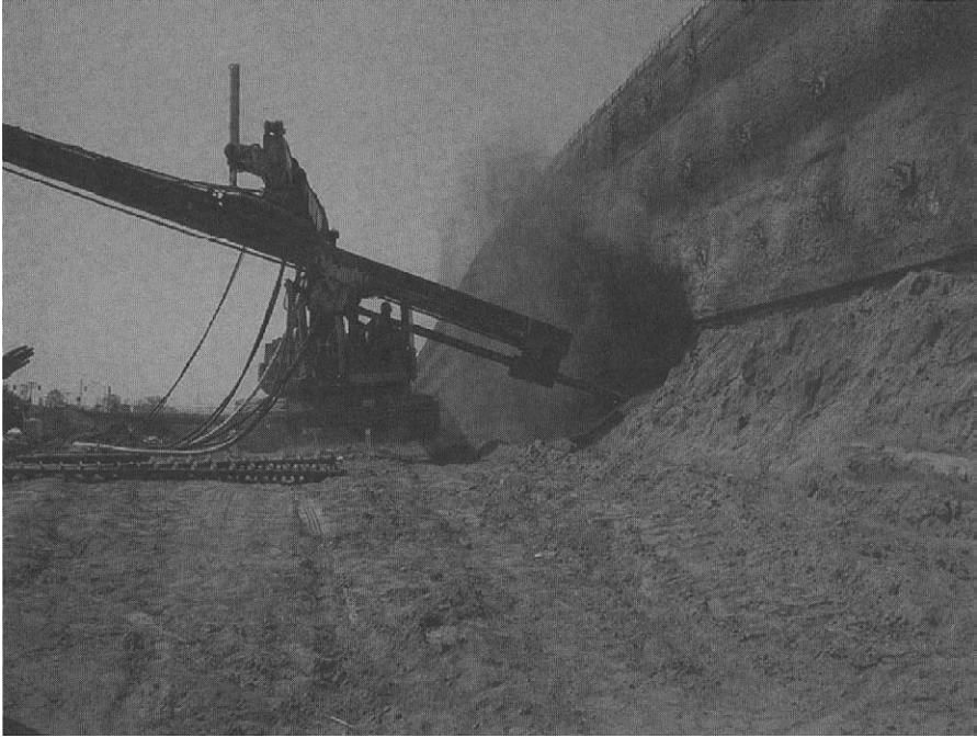
Figure 25.5 Augering for horizontal soil anchors ( Source: California DOT)
