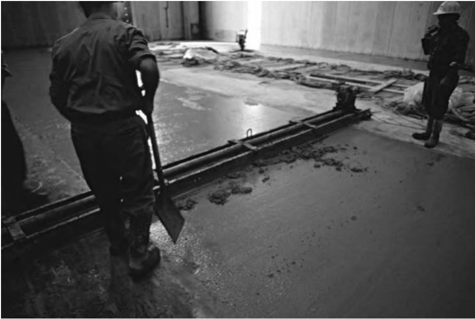
Figure 17.3 Double-beam vibrating screed
