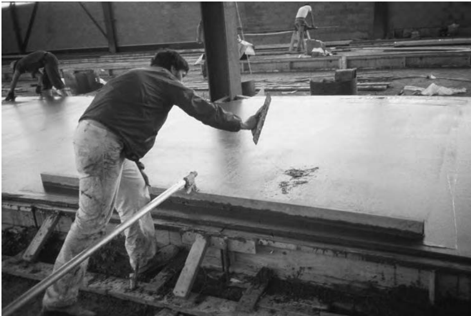
Figure 19.8 Superflat construction – filling a low spot that the highway straightedge has revealed
