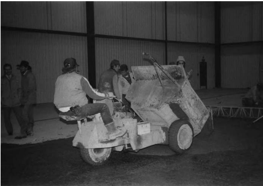
Figure 11.2 Using a power dumper (buggy) to place concrete for a thin, bonded topping
