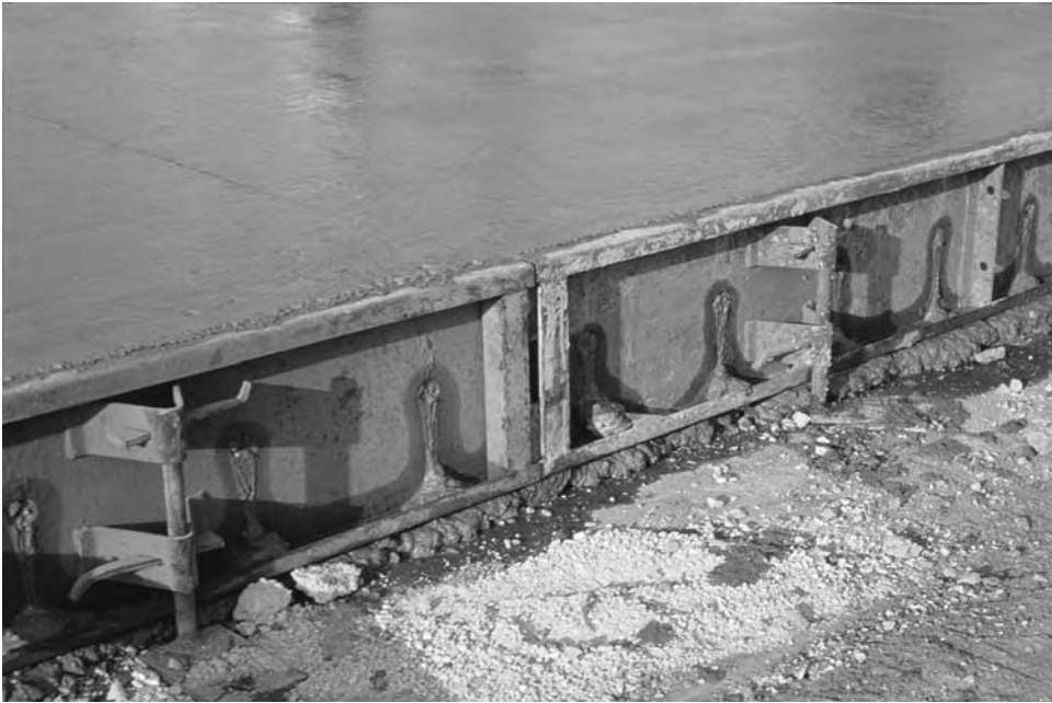
Figure 11.12 Steel form
