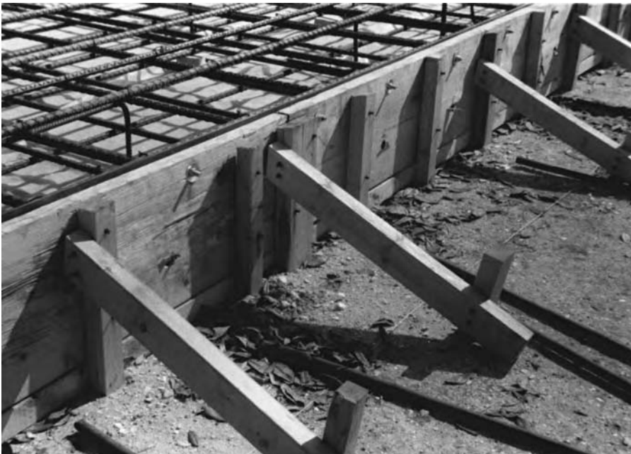
Figure 11.13 Heavily braced timber form
