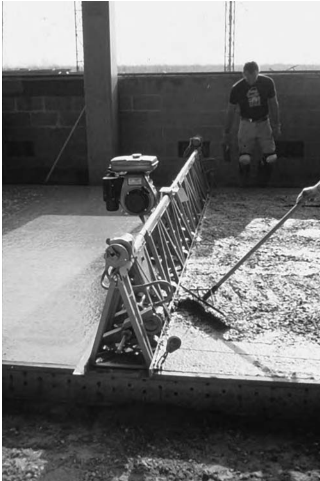
Figure 17.4 Truss-type vibrating screed
