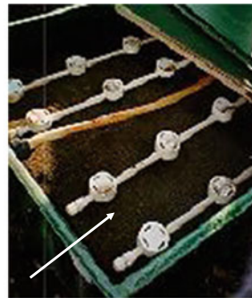
b. A layer of sand and clogging materials removed from the infiltrative surface zone of a single pass sand filter to rejuvenate its hydraulic capacity.
