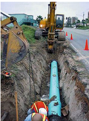
Fig. 5.3 Photographs of conventional sewer line installation
