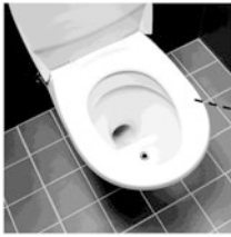
Fig. 4.11 Example of urine diversion in a residential development using urine diverting toilets with nutrient recovery via agricultural fertilizer (Jønsson et al. 2000)
