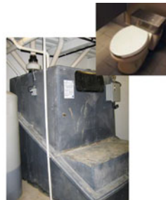
c. Photograph of a composting toilet system with a centralized composting unit suitable for 65,000 uses per year. (source: www.clivusmultrum.com/green-building-projects.php )
