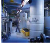
Fig. 1.19 Example of a membrane bioreactor system serving a high rise apartment building in a major urban area to produce reclaimed water for nonpotable reuse and help earn LEED certification. (Photographs are of the Solaire building in Battery Park City, NY which has 250 apartment units. http://www.werf.org/i/c/Decentralizedproject/When_to_Consider_Dis.aspx )
