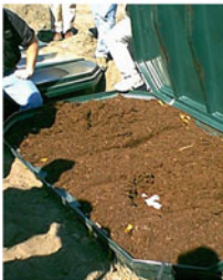
a. Peat media is containerized in a basin unit with a distribution and underdrain system built in. Effluent is intermittently dosed onto the filter surface.
