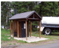
a. Photograph of a vault toilet and it being emptied by a pumper truck. (source: http://www.rvsws.com/Vaults.htm )
