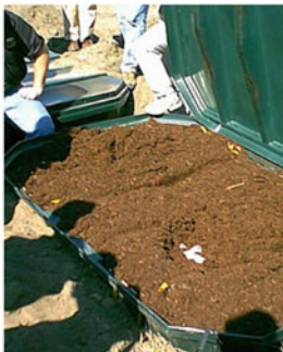
a. Example of a module for a PBF using peat manufactured by Anua Puraflo®
