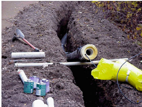
Fig. 5.27 Photograph of insulated pipe used for shallow burial of sewer pipe in a cold climate. (Photograph courtesy of R. J. Otis)
