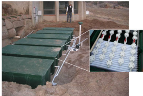
b. Example of a module for a PBF using textile sheets made by Orenco Systems® Inc.
