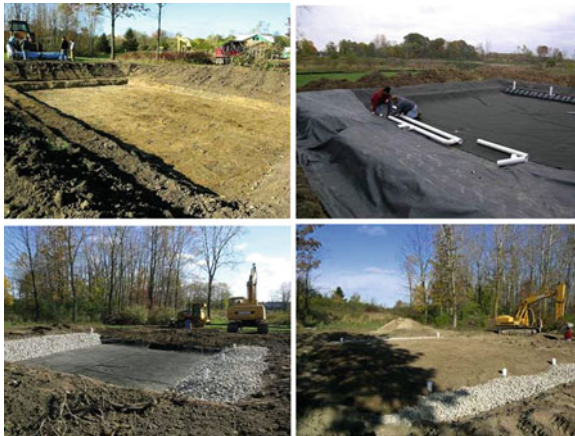
Fig. 10.18 Photographs of a VSB wetland during construction (Source: www.goshen.edu/merrylea/collegiate/riethvillage.html ) 10.64
