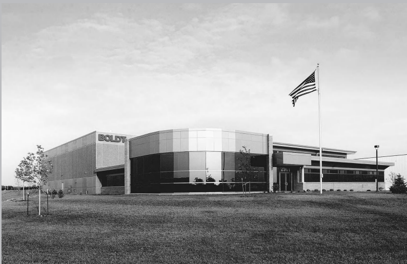
Figure 8-2 Photo courtesy of The Boldt Company.
