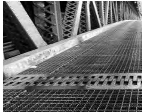
(b) Bridge expansion joint
