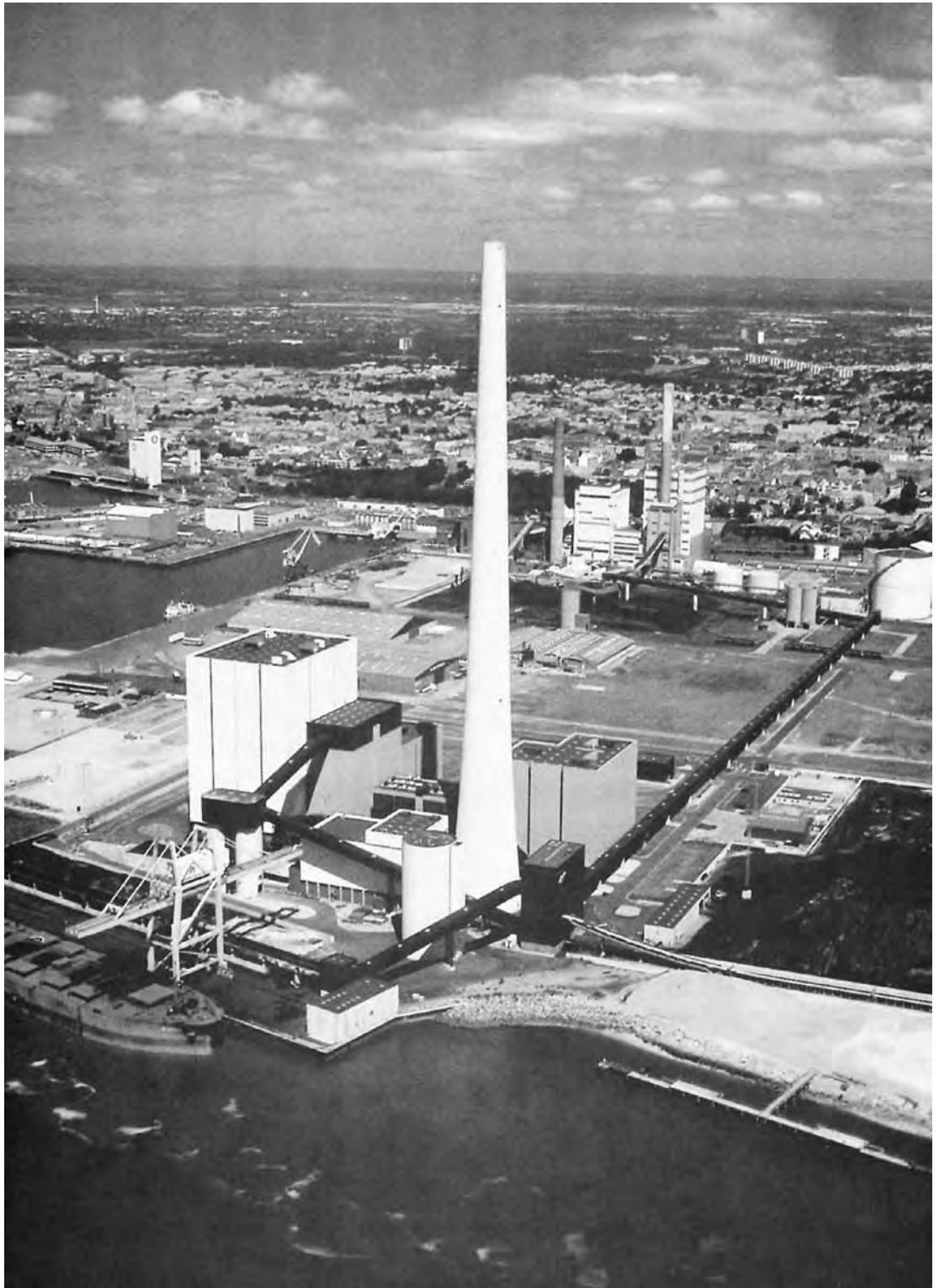
FIGURE 1.2 The Esbjerg, Denmark, power station. (Courtesy Vestkraft 1996.)
