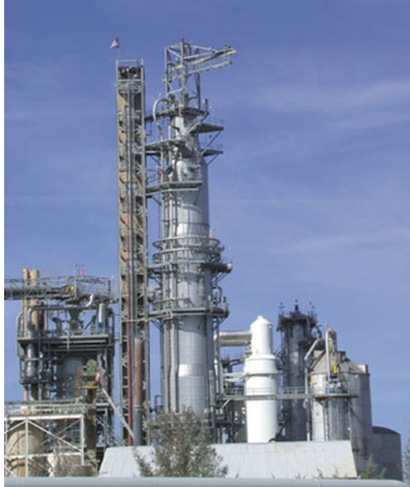
Fig. 5.12 Continuous digester, Catawba's new fibre line, uses low solids cooking for lowest kappa number and highest fibre quality (Shaw 2004. Reproduced with permission)
