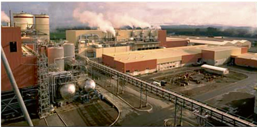
Fig. 5.4 Celulosa Arauco y Constitucion’s new facility in Valdivia Province, Chile (Rodden 2005. Reproduced with permission)
