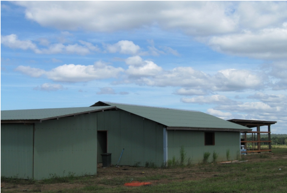
Fig. 3. The Garrathiya Dormitory and Outbuildings during Construction
