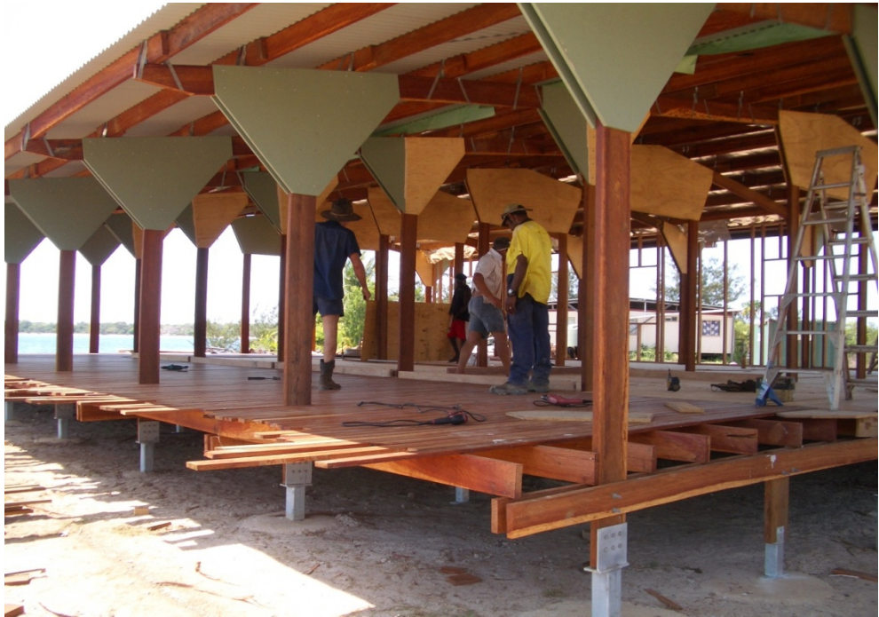
Fig. 6. The Dhanaya House during Construction
