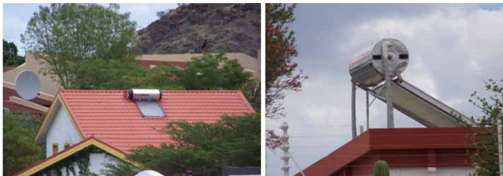
Fig. 2. Indirect Solar Water Heater Systems with heat collector. Source: Wienecke and Mawisa ,(2008).p.15.
