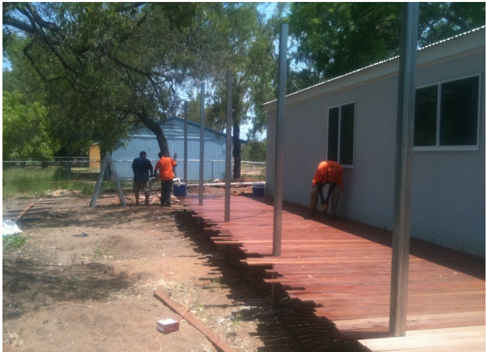
Fig. 9. Gumatj Men Constructing a Verandah on a Kit Home at Gunyangara
