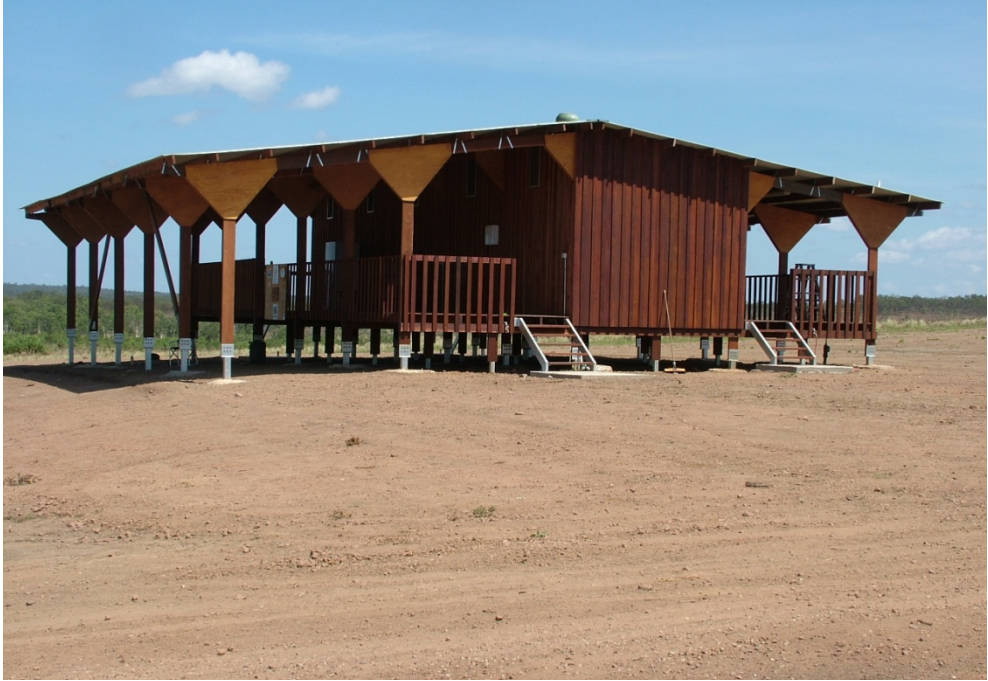
Fig. 5. The Garrathiya Five Room Bunkhouse
