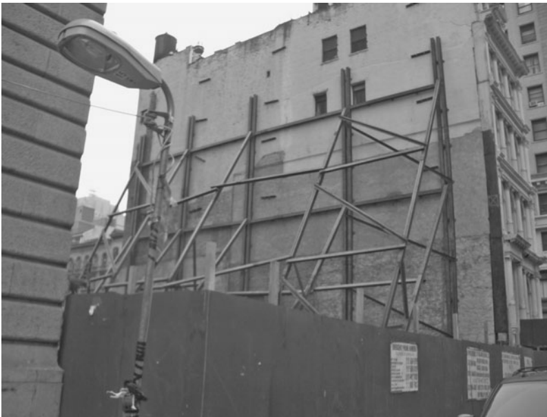
Exhibit 6-37 Bracing of wall.
