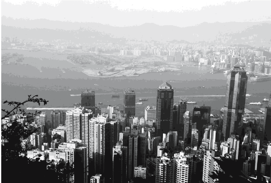
Fig. 4.7 Reclaimed land in West Kowloon, as seen from the south (Photo: Breitung, March 1998). With Hong Kong's skyline in the foreground, the low-rise character of the densely built-up area of Kowloon is easily identified at the back, to the right. The height restriction originates from the period when the district served as an airport landing corridor. At the centre of the picture, tunnel entrances and the railway station construction site mark the area of the then still undeveloped new land. Transport links to the airport are seen in the photo at the back, to the left.
