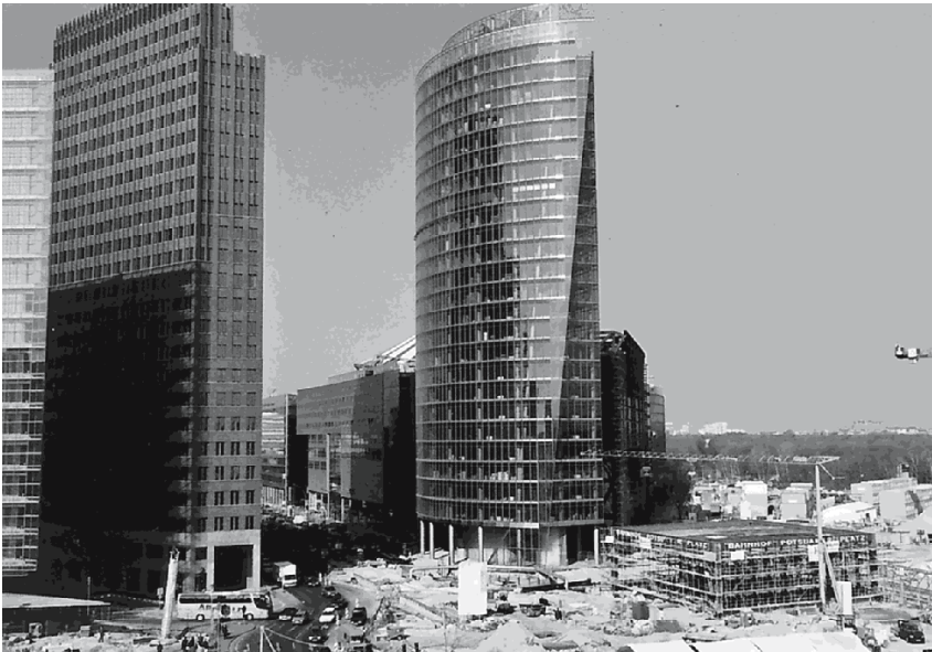
Photo 2.5 Office towers flanking both sides of Potsdamer Straße. The office block designed by Hans Kollhoff is to the left, the multiple-use Sony Centre complex on the right. The latter is due for completion in 2000 (Source: Lenz, April 2000).
