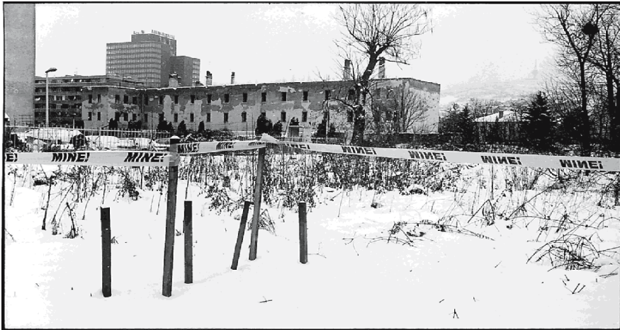
Fig. 5.2 Destroyed shack of the "Marshall Tito" barracks in Sarajevo, with minefields in the foreground (Photo: R. Schmid)
