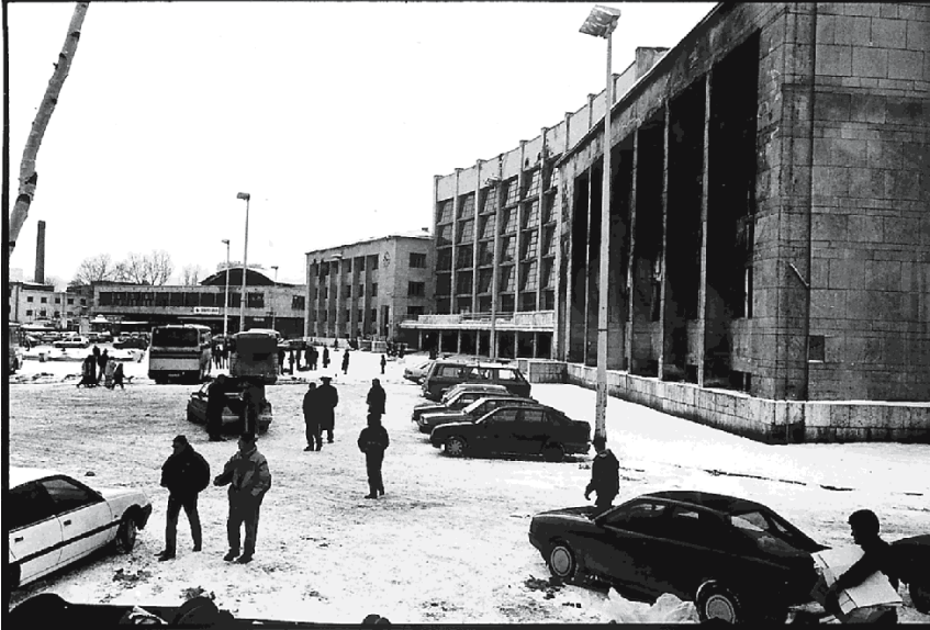
Fig. 5.7 Partially destroyed railway station of Sarajevo (Photo: R. Schmid)
