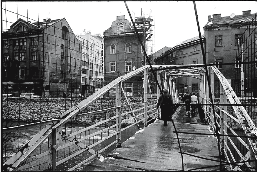
Fig. 5.1 Damaged bridge over the Miljacka river, Obala Kulina Bana, Sarajevo (Photo: R. Schmid)
