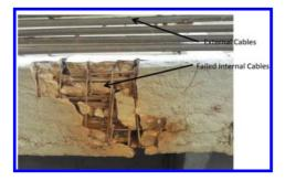
Figure 4. Cracks in damaged girder (soffit of girder).
