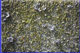
Figure 13. Dense biological covering affecting the façades of the ATM towers (Ivry-sur-Seine, 1963–1967). The biological covering is mainly composed of algae and lichens.
