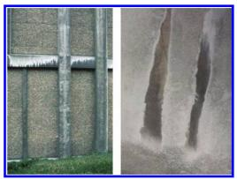
Figure 7. Example of black dirt deposits with different morphologies and thickness. Left picture: Saint-Joseph Church (Le Havre, 1951–1957). Right picture: Le Signal (Le Havre, 1959–1960).
