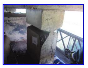
Figure 10. 3 mm Cracks and spalling to side of hinge: Pier 6.
