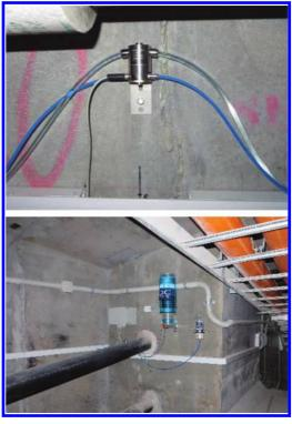
Figure 2. Installation of the monitoring system inside the concrete box girders of the Hunter Expressway.
