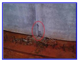
Figure 5. Crack of panel due to sliding restraint during stressing.
