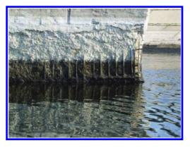
Figure 1. Frost damage on a hydraulic engineering structure in Saratov (Russia).
