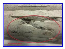
Figure 8. Honeycombing defect.
