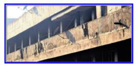
Figure 5. PGI Nehru Hospital Building Sector-12, Chandigarh: Damaged exposed concrete façade.
