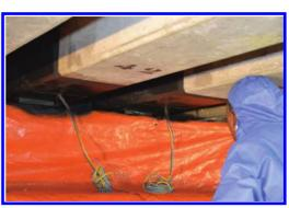
Figure 8. Applying the conductive coating  $(CAST^{3+}$  system).
