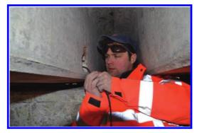
Figure 7. Restricted work space for concrete repair and CP installation.
