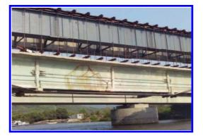
Figure 11. Main girders launched over the damaged span.
