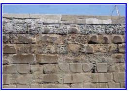
Figure 8. Pockets at block joints from 2013 survey.
