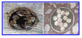
Figure 11. Transverse cable in Nels deck on left. Example of suitably bonded cable on right.
