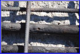
Figure 15. Despite heavily corroded tendons and 6 mm deep "pits", no fractures in the tendons were found at locations away from the couplers.
