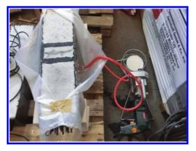
Figure 3. Crack injection by means of a hose pump.
