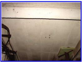
Figure 4. Repairs reinforced concrete floors with special mortars. Good conditions in service case (2004–2014).
