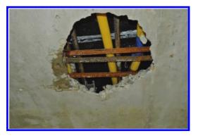
Figure 10. Void area below air duct with rebars and service cable ducts.
