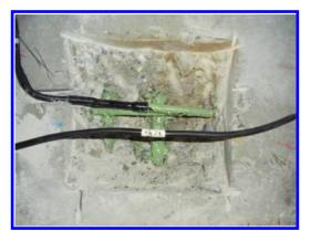
Figure 3. Cathode connection by welding to an exposed rebar in an opening at the column socket. After welding, the connection point was electrically insulated with an epoxy resin.
