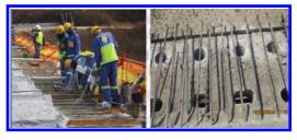
Figure 12. Cores introduced in deck cantilever
