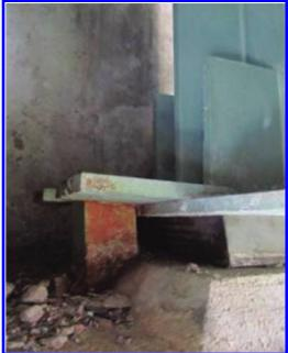
Figure 4. Right side bearing of the "la Sarraz" abutment.
