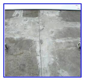
Figure 1. Premature failure of a crack repair due to thermal movement of plain concrete (Fort Bezuiden Spaarndam, part of the Defense Line of Amsterdam, 1897–1901, UNESCO World heritage site, intervention 1998, situation 2006).
