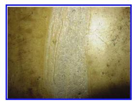
Figure 1. Soft concrete surface.
