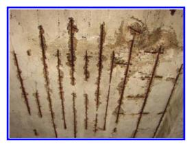
Figure 3. Medium level of deterioration at reinforced concrete floors. It's necessary repairs with special mortars (2004).
