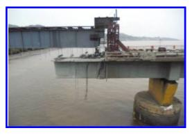
Figures 14. Lowering of girder segments by partly completed.
