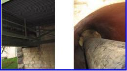
Figure 10. Water pipe behind the bearings "Ferreyres" abutment.
