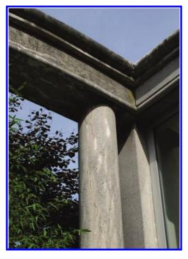
Figure 4. Prefab column made with coloured concrete and specially chosen aggregates, now showing cracks and leaching, indicating ASR (Giraffe compound, Zoo Blijdorp, Rotterdam, S. van Ravesteyn, 1940).
