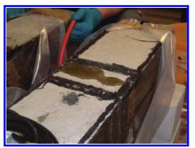
Figure 4. Complete injection of the crack.
