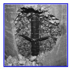
Photo 9. Exposed re-bar at 1st floor in No. 3.
