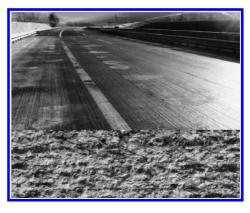
Figure 15. Finished bridge deck and final road surface after milling.
