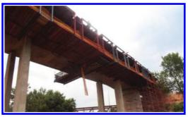
Figure 16. Deck construction frames and platforms.
