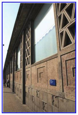
Figure 5. Several railway station built during the post—war reconstruction period were made with pre-fab concrete elements, other which special aggregates and surface finishes (for example railway station Enschede, H.G.J. Schelling, 1950).
