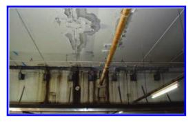
Figure 2. Moisture penetration through the joints between the slabs.
