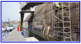
Figure 15. Concrete overlay on marina block foundation left over from the Hermitage construction.
