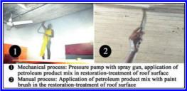
Figure 12. Application of petroleum base mix in restoration-treatment of roof surface in faculty room CCA Building.
