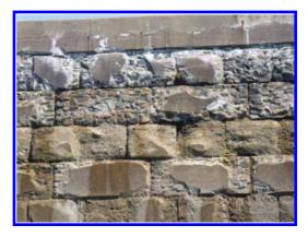
Figure 12. Loss of surface and other pockets at joints.
