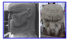
Figure 18. Monumental head sculpted in a concrete block by Carlo Sarabezolles for the bell tower of Notre-Dame des Missions church (Epinay-sur-Seine, 1932). Left picture: view of 1933. Right picture: view of 2009 evidencing a loss of sculpted details due to erosion/lixiviation.
