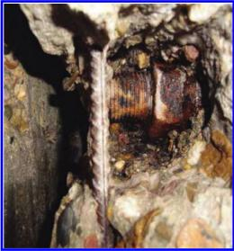
Figure 3. Surface corrosion of an anchor of a prestressing tendon.
