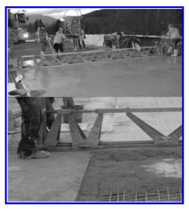
Figure 13. Casting of the bridge with crane bucket and manufacturing the construction joint.
