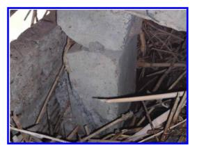
Figure 6. Splitting collapse of concrete hinge bearing at Pier 9.
