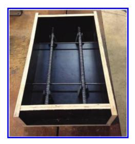
Figure 1. Typical slab arrangement.
