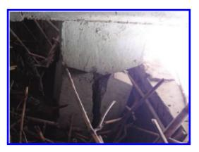
Figure 4. Splitting collapse of concrete hinge bearing at Pier 9.
