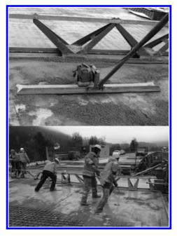
Figure 14. Compacting the first layer with wet screed and the second layer with vibrating beam.
