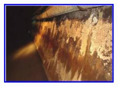
Figure 2. Liquefaction of the concrete segments surface layers.
