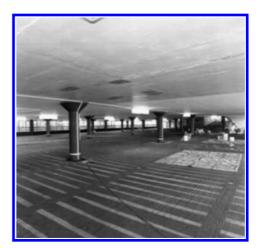
Photograph 2. Zebra deck anode installed prior to deck surfacing.
