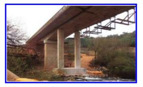
Figure 15. View of bridge showing one set of temporary supports and the support frames hanging from the deck.
