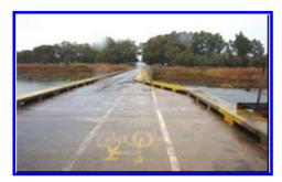
Low level bridge-reduced cross section.
