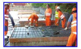
Figure 3. Concreting the R-UHPFRC strengthening layer.
