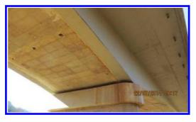
Figure 17. Soffit of deck showing new beam and widened pier head.
