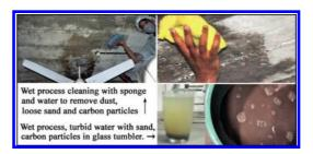
Figure 10. CCA Faculty Room roof surface: Wet process cleaning.
