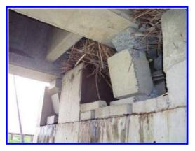
Figure 1. Collapsed concrete hinge bearings.
