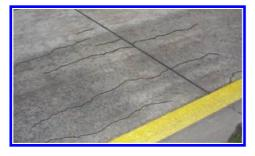
Figure 1. Advanced stage of ASR-damage with longitudinal cracking in the concrete pavement.
