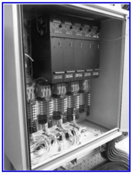
Photograph 15. Transformer rectifier with 5 power zones.
