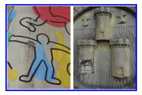
Figure 22. Carbonation induced corrosion can generate spalling, which means important loss of original material, but also a possible impact on the artwork understandability. Left picture: Keith Haring mural of Necker's Hospital (Paris, 1971). Right picture: High-relief of the bell tower of Dinan train station (Dinan, 1931).
