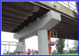
Figure 9. As-built CP system with 4 decentralized power supply and monitoring units.
