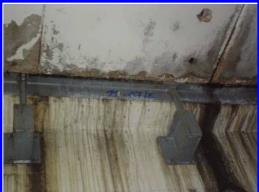
Figure 3. Steel girder construction to strengthen the supports.
