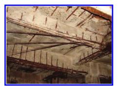
Figure 2. Deterioration from durability at beams. Maximum level of deterioration led to the disintegration of reinforcement.
