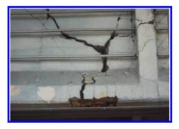
Figure 3. Cracks in damaged girder (Elevation of girder).
