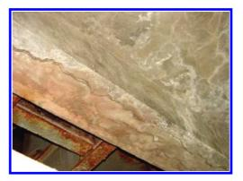
Figure 7. Strengthening beams with reinforced concrete. Bad conditions in service case (2004–2014): restarting the corrosion of reinforcement and new cracks in strengthening beams.
