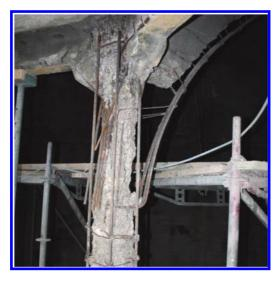
Figure 2. Large-scale removal of historic concrete during repair (circumambulation passageway Pilgrimage church, Brielle, H. Goossens (reconstruction), E.J. Margy, 1912).
