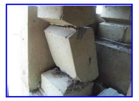
Figure 5. Collapsed concrete hinge bearing at Pier 9.
