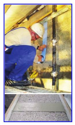
Figure 4. De-bonding materials. Top:acrylic-adhesive with HDPE-film, bottom: cement-based coat (StoCrete FB).
