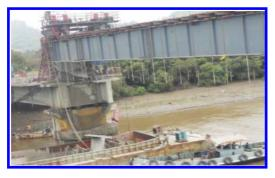
Figure 15. Lowering of existing damaged girders completed and last segment lowered in the barge.
