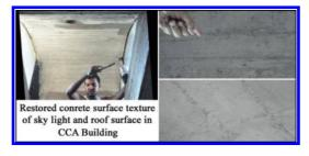
Figure 13. CCA Building faculty room "roof surface" showing, conserved and protected surface texture after restoration and treatment.
