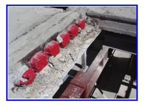
Figure 8. broken-off concrete in the damage support area.
