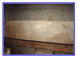
Figure 8. Strengthening beams with reinforced concrete. Bad conditions in service case (2004–2014): new cracks in strengthening beams.
