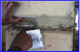
Figure 9. 2 mm Crack in throat of hinge: Pier 3.
