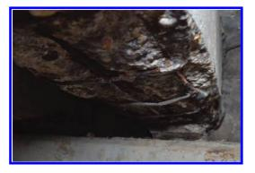
Figure 2. Concrete damage and corrosion of mild steel reinforcement.
