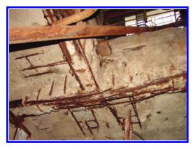
Figure 5. Major level of deterioration at beams. It's necessary strengthening with reinforced concrete (2004).
