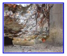
Figure 5. Severely damaged beam head after removing delaminated concrete.
