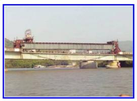
Figure 12. Main girders launched over the damaged span.
