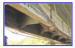
Figure 2. Bottom view of external pre-stressing.
