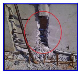
Figure 6. Defects of precast wall panels.
