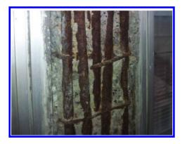
Figure 7. Corroded rebar.
