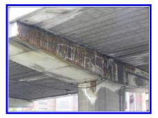
Figure 3. Concrete delamination on crosshead cantilever faces.
