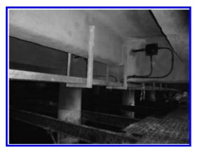
Photograph 14. Berth 4 Junction box and cable tray arrangement.
