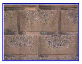
Figure 17. Wall of the city of Grenoble (end of 19th century). The erosion and lixiviation phenomena revealed the presence of aggregates and therefore evidenced that it was not cut stone, but fake stones made of natural-cement-based concrete.
