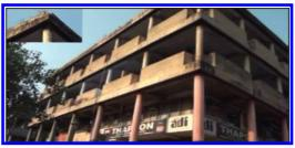
Figure 4. View of RCC Building, Sector 17, Chandigarh: Damaged surface texture due to decay and carbonation.
