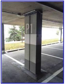
Figure 4. Column socket with discrete anodes (compare Figure 1).
