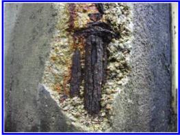
Figure 21. Wind tunnel erected between 1932 and 1934 to test aerodynamic performances of big size models (Meudon, 1932–1934). Due to the wind tunnel activity the concrete walls were carbonated on their entire thickness. In this monument, impressive corrosion facies were observed.
