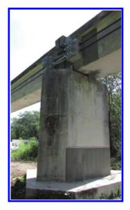
Figure 8. Reinforcement of the pier bases with composites.
