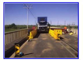
Figure 8. Limited width temporary accommodation of traffic.
