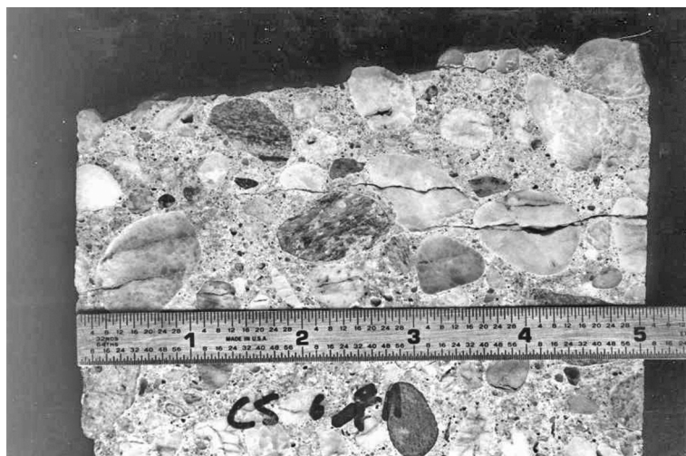
Fig. 4.5.1. This section is concerned with minimizing ASR, but it is nevertheless useful to know what ASR looks like. Here is a typical situation. Cracking parallel to the exterior surface of the concrete goes both through and around the aggregate particles. Also, although it is difficult to discern, the alkali-silica gel lines the surface of some of the cracks and air voids. (Photograph taken by Margaret Hanson Reed, WJE Northbrook IL)
