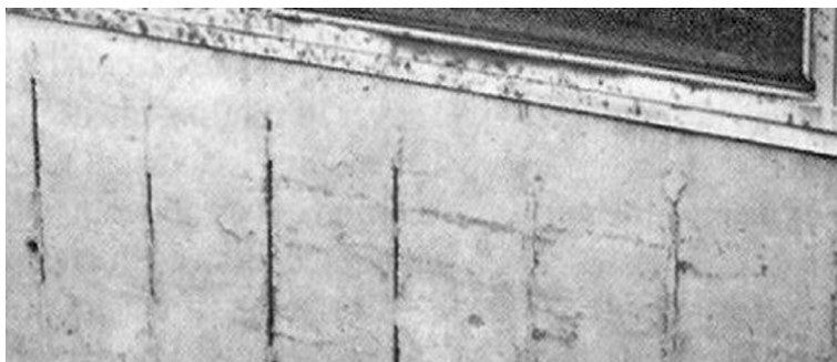
Fig. 6.1.1. Negative cover to reinforcement
