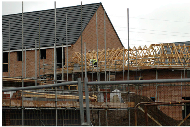
Figure 14.2 Typical construction site
