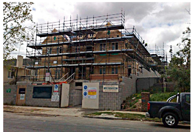
Figure 14.1 Construction site entrance
