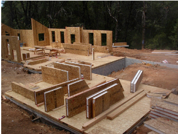
Figure 11.16 Insulated core panels
