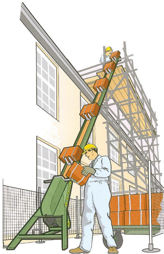
Figure 8.12 A brick elevator. Source HSE
