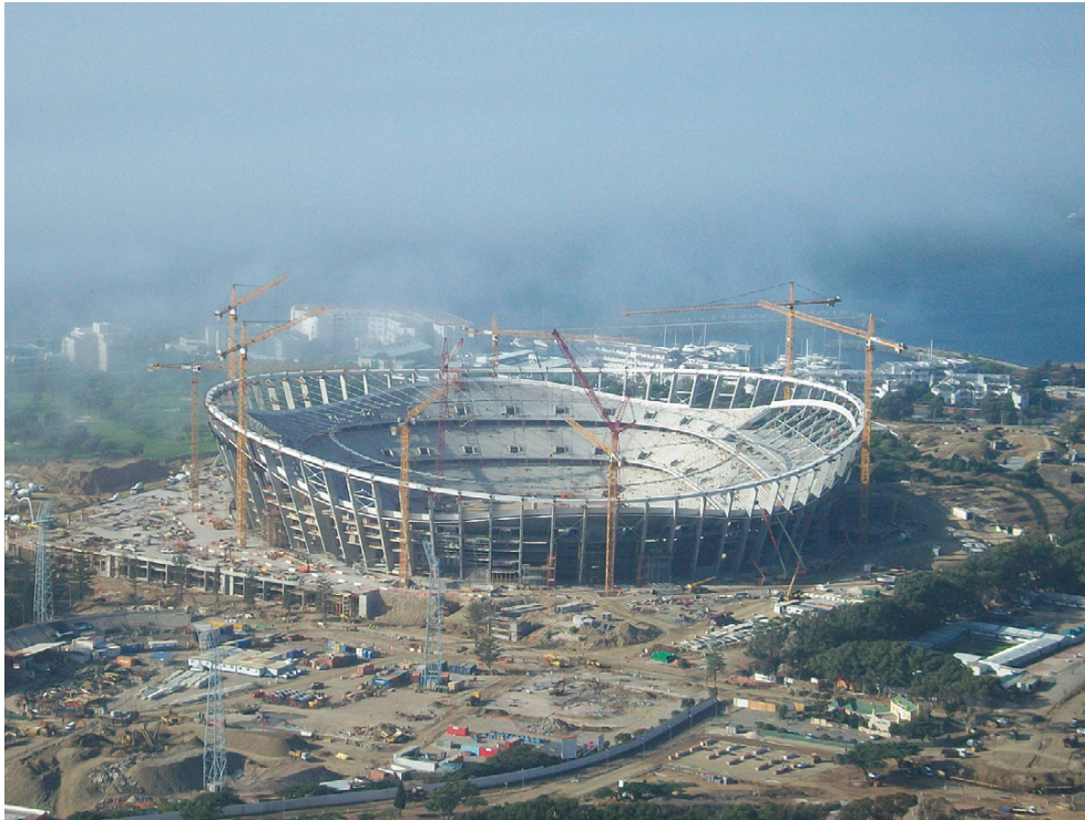
Figure 14.17 World cup stadium-under construction, Cape Town, 2009
