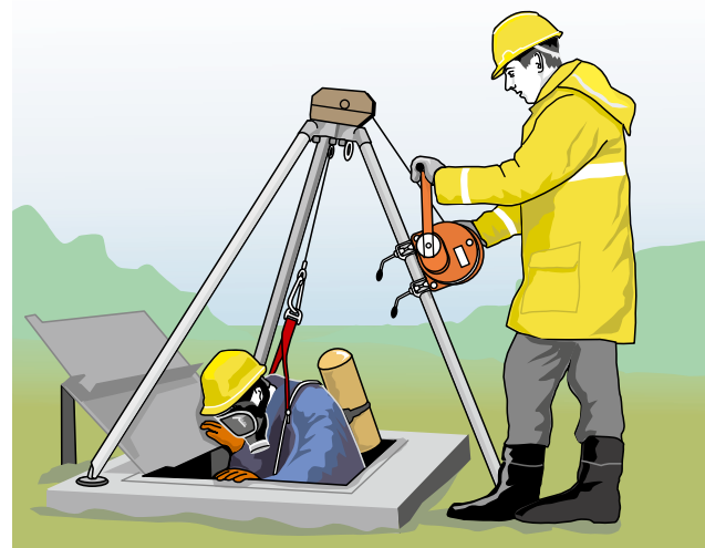
Figure 4.28 Entering a confined space with breathing apparatus, rescue tripod and rescue watcher
