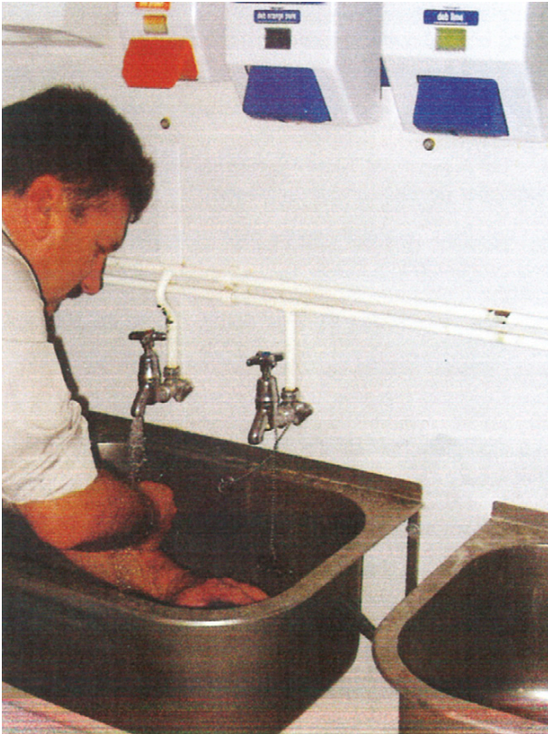
Figure 4.24 Welfare washing facilities: washbasin large enough for people to wash their forearms
