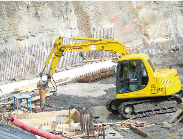
Figure 13.6 Breaker mounted on an excavator's jib to reduce vibrations
