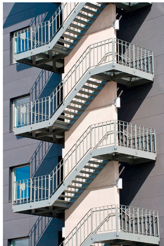
Figure 11.22 External fire escape from a multi-storey building. Extreme caution needed in winter and enclosure of staircase would be preferred for the UK climate
