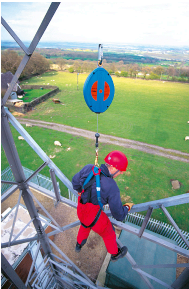
Figure 6.13 Fall arrest harness and device
