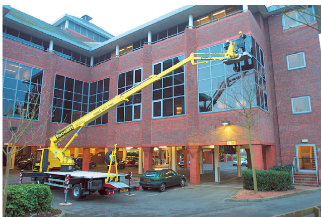
Figure 1.16 Contractors at work from a lorry-mounted MEWP
