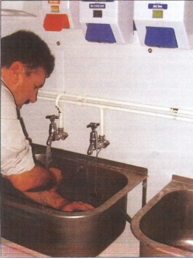
Figure 6.1 Welfare washing facilities: Washbasin large enough for people to wash their forearms
