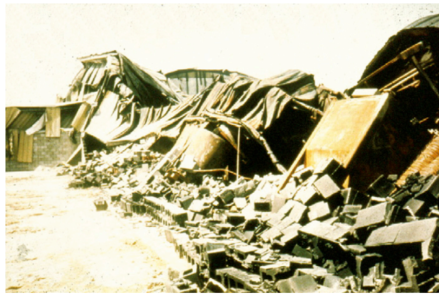
Figure 11.15 Steel structures can collapse in the heat of a fire
