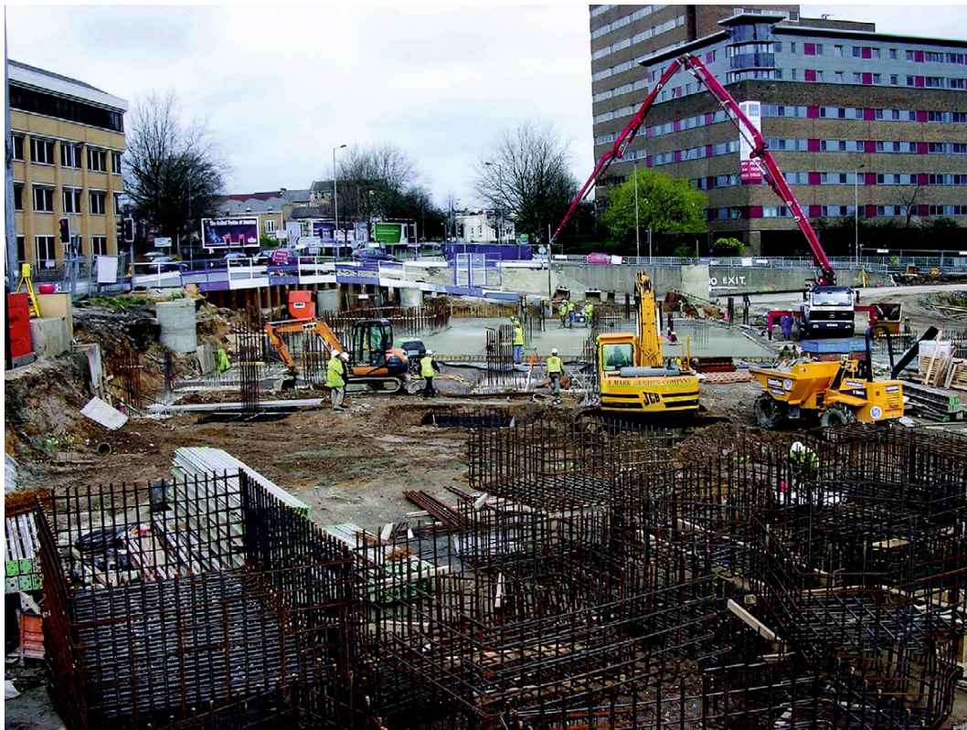
Figure 14.3 Groundwork clearance and foundations
