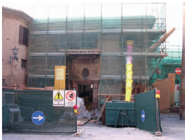
Figure 18.10 Construction site – Sienna.
