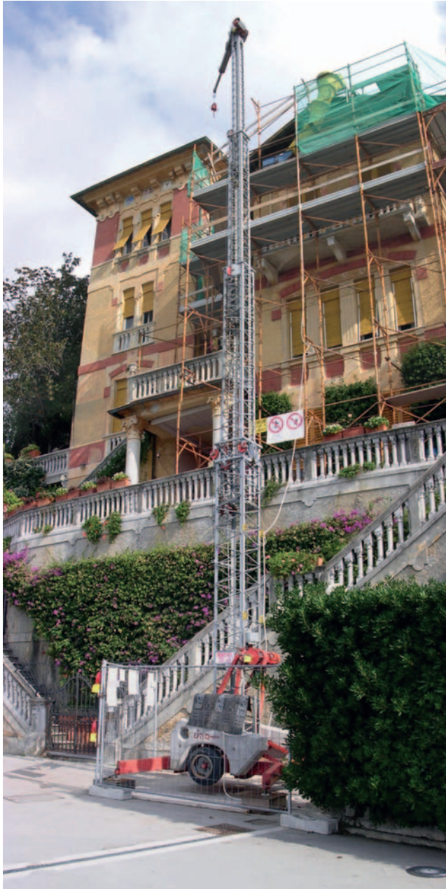
Figure 18.13 Mobile tower crane – Cinque Terre, Italy.
