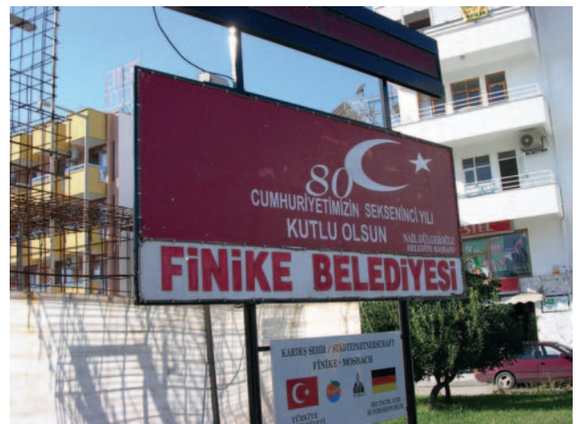
Figure 18.2 Local authority building site, Turkey.
