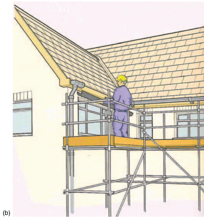
Figure 16.10 (a) Typical independent tied scaffold. (b) Fixed scaffold left in place to fit the gutters.
