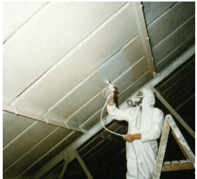
Figure 5.5 A lone worker – special arrangements are required.
