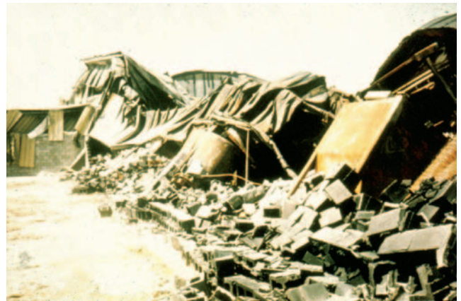
Figure 13.11 Steel structures can collapse in the heat of a fire.
