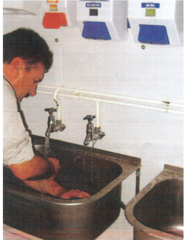
Figure 6.15 Welfare washing facilities: washbasin large enough for people to wash their forearms.
