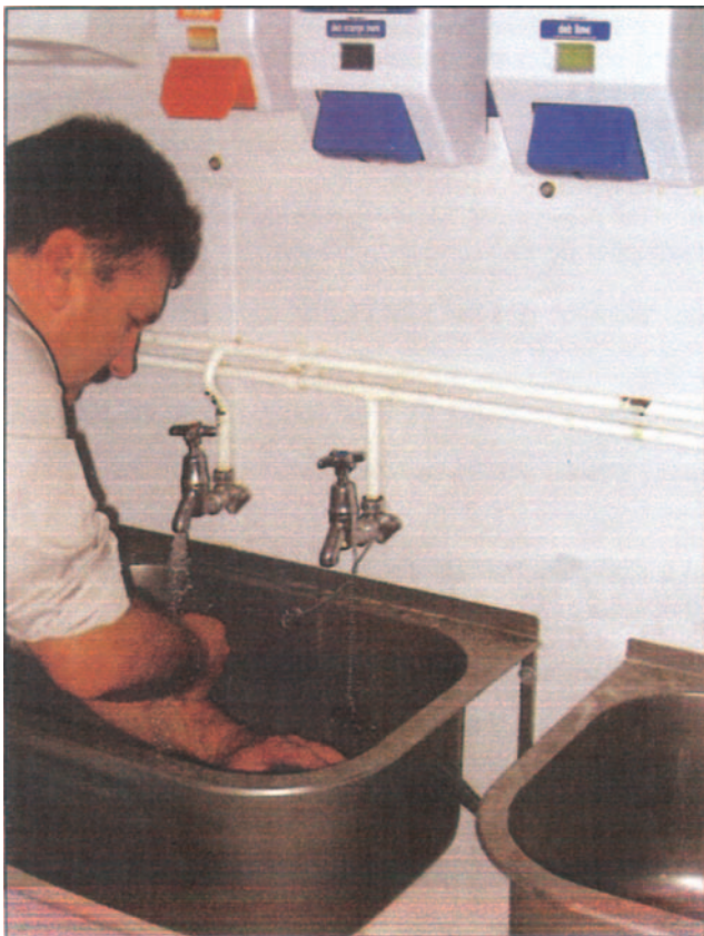
Figure 16.4 Welfare: washing facilities – washbasin large enough for people to wash their forearms.
