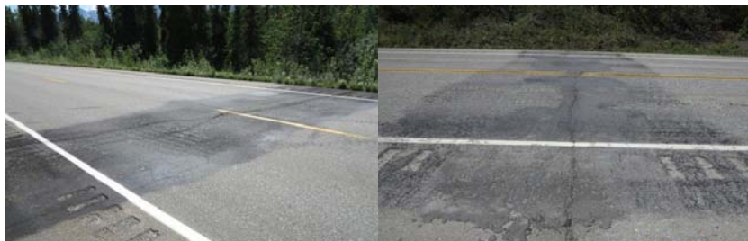
FIG. 12. Examples of patch/seal band maintenance of major transverse thermal cracks
