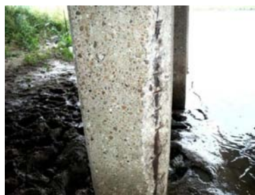
(f) Column exposed corroded rebar
