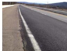
(c) Bobcat mill-and-pave
