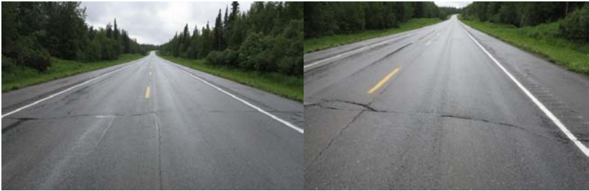
FIG. 11. Severe major transverse cracks with little influence on pavement performance beyond crack edges
