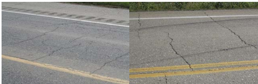
FIG. 10. Lessor thermal cracks showing same performance in wheel path and non-wheel path locations (common appearance)
