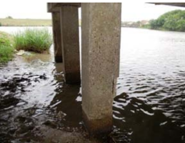
(e) Column with peeled off concrete
