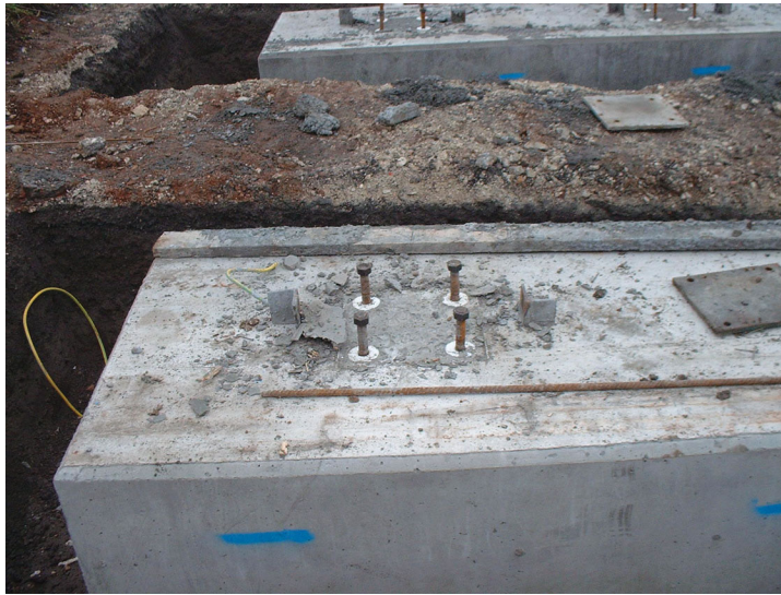
FIGURE 28.4 Holding Down Bolts With the Expanded Polystyrene Void Formers Still in Position Around Them
