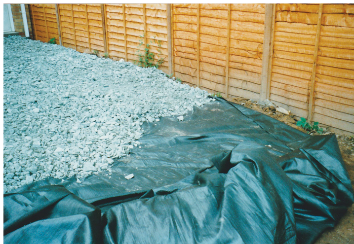
FIGURE 35.4 Typical Use of Geotextile to Stabilise a Driveway Before Placement of Block Paving
