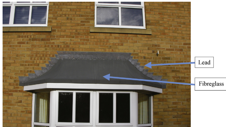
FIGURE 38.5 The Roof Section Over the Bay Window is Made out of Fibreglass to Look Like Lead
