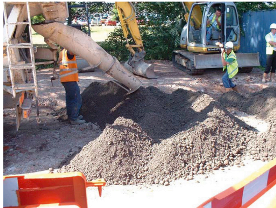
FIGURE 17.4 Semidry Concrete for a Road Foundation
