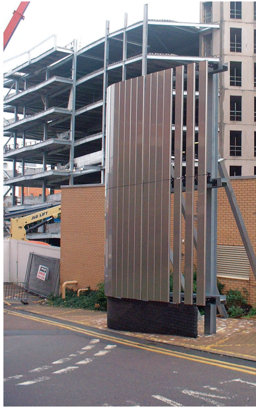
FIGURE 31.20 A Sample Panel of Stainless Steel Cladding Panels for use on the Car Park Behind that is Under Construction
