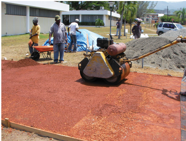
FIGURE 41.1 Roller Compacted Zero Cement Concrete in Jamaica
