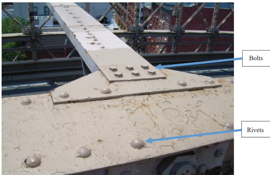
FIGURE 30.12 Bolts and Rivets on the Brooklyn Bridge in New York
