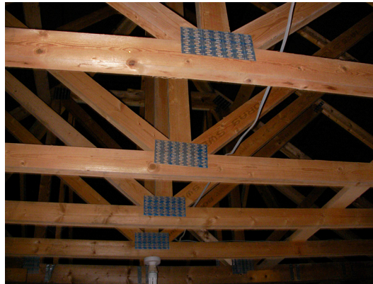
FIGURE 33.6 Typical Application of Metal Plate Fasteners
