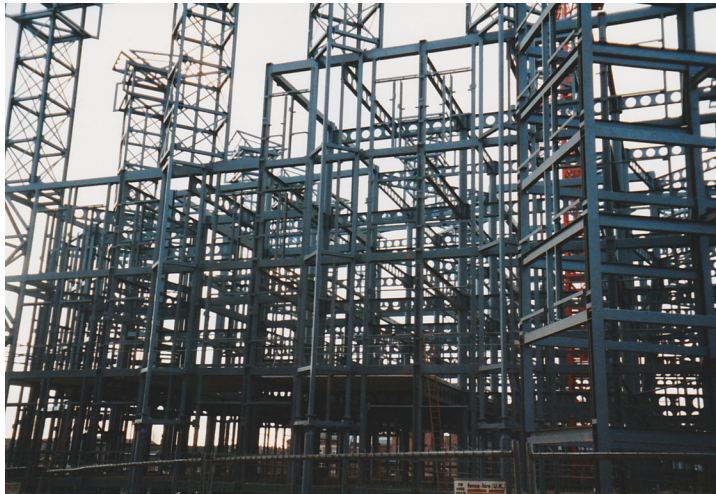
FIGURE 30.1 A Substantial Steel Frame for a Library That has High Loadings From the Books
