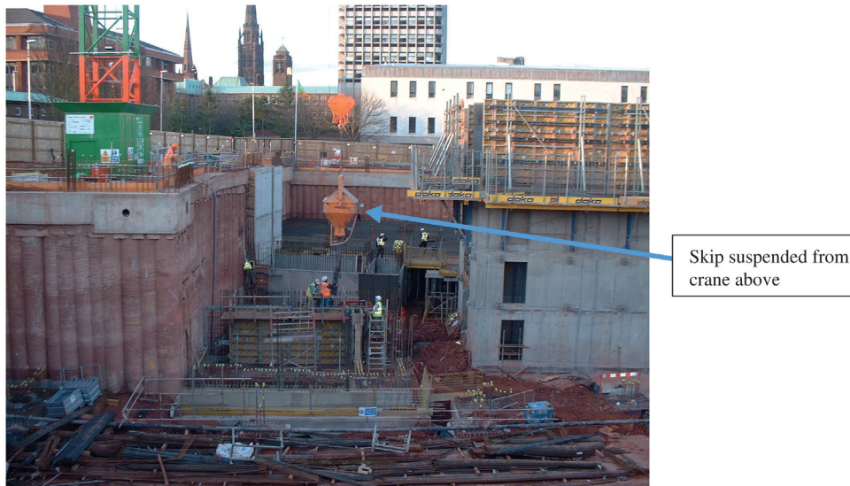
FIGURE 26.7 Concrete Placement From a Skip for a Below Ground Parking Garage
