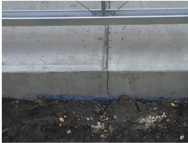
FIGURE 23.6 Crack Caused by Crack Inducer
