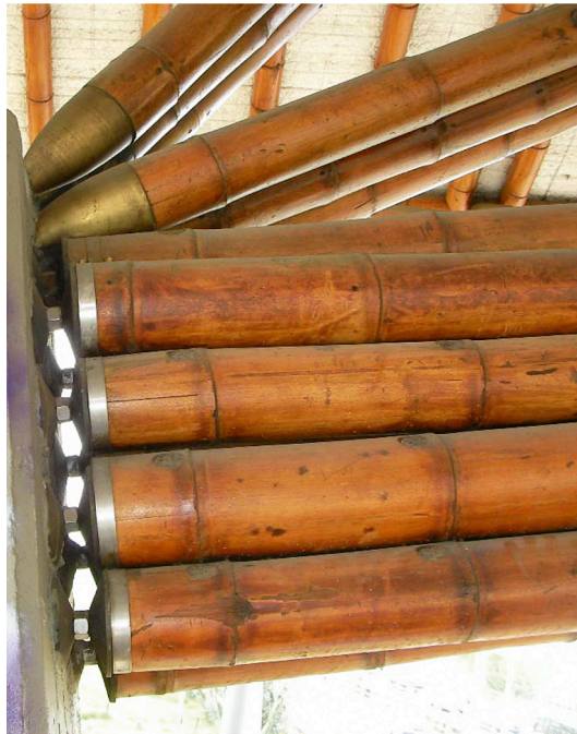
FIGURE 33.11 Tidy Metal End Connectors on Bamboo
