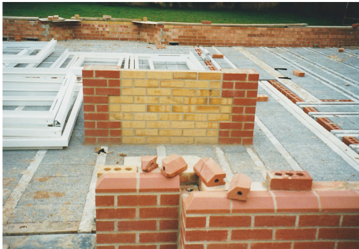
FIGURE 34.16 Sample Panel Built to Include Proposed Features of Finished Work
