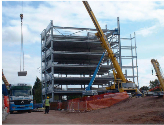
FIGURE 17.1 Lifting Precast Pretensioned Concrete Flooring Units onto a Steel Frame
