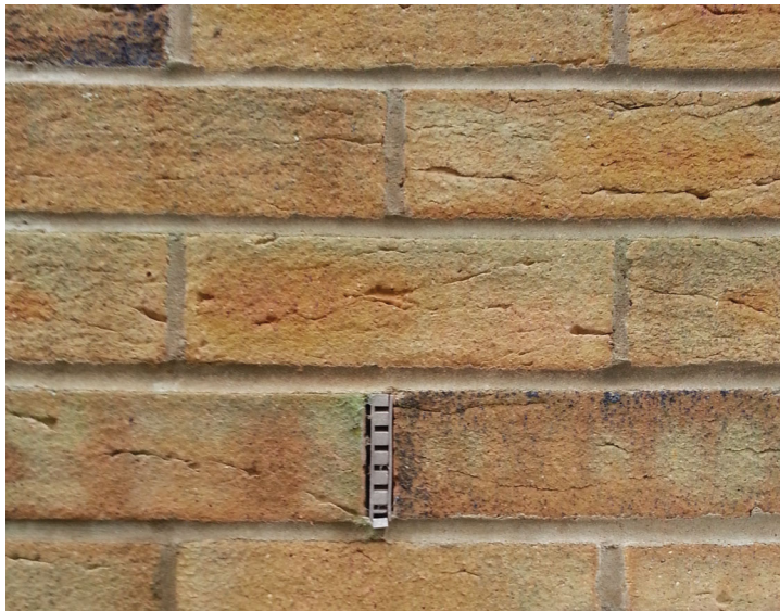
FIGURE 34.13 Weep Hole with Plastic Fitting in it to Keep it Clear
