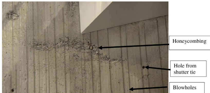
FIGURE 26.4 Defects in Concrete Surface
