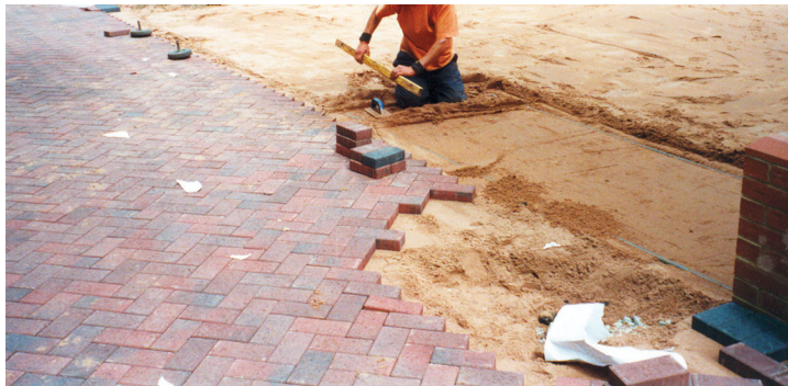
FIGURE 34.5 Brick Paving with Concrete Bricks
