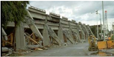
Figure 1. Cypress viaduct, collapsed in Loma Prieta earthquake.
