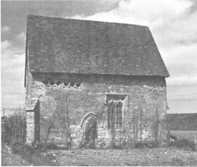
94 The chapel at Bradwell Priory, Buckinghamshire, before restoration (R.C.H.M.)
