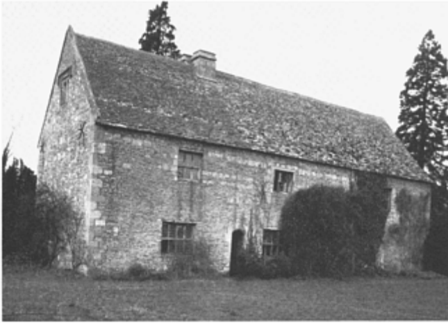
149 Late-medieval survivals in the detailing of doors and windows at the 'Priory', Marcham, in Berkshire, the building being otherwise characteristically early-modern in plan (R.C.H.M.)
