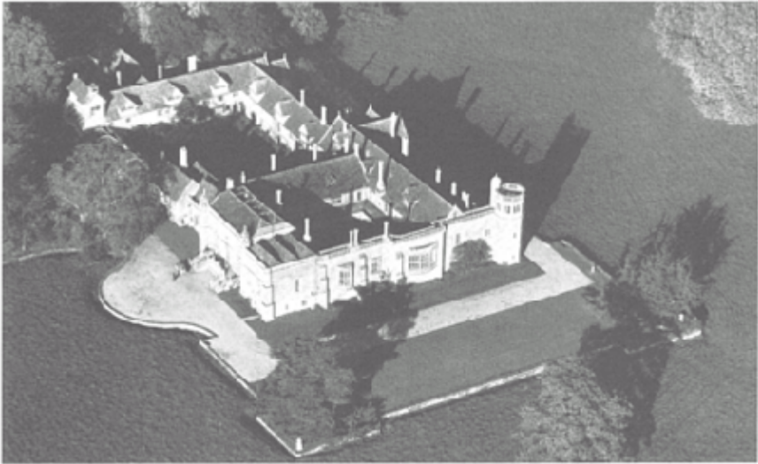
143 Sir William Sharington's re-use of the claustral buildings at Lacock Abbey, Wiltshire, later remodelled in the mid-eighteenth-century 'Gothick' style (Aerofilms)
