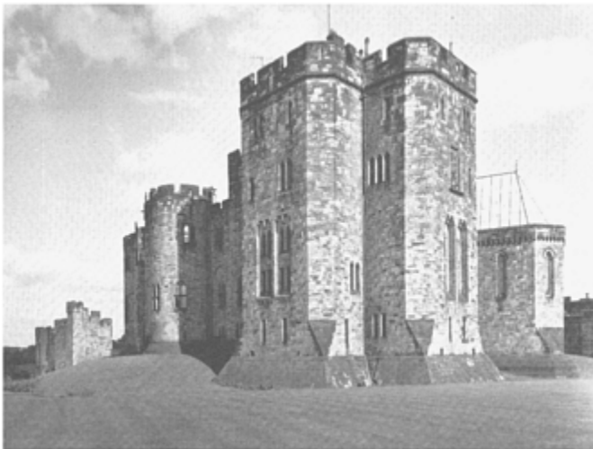
117 The keep at the great Percy fortress at Alnwick, in Northumberland, completed in the late fourteenth century (Hallam Ashley)
