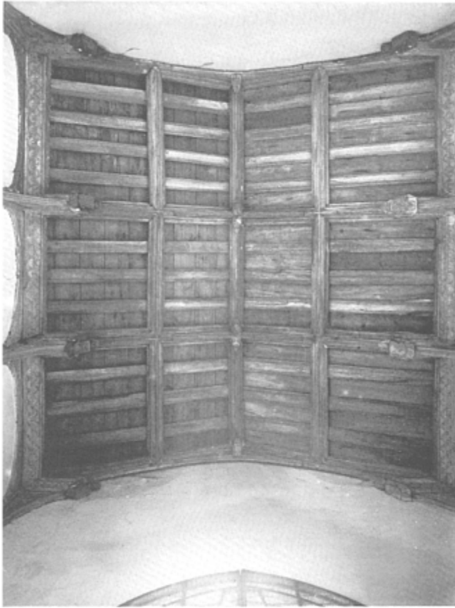
91 The porch roof at Swaffham Church, financed by William and Anne Coo who 'did make the Roffe of the porche'; fifteenth-century (R.C.H.M.)
