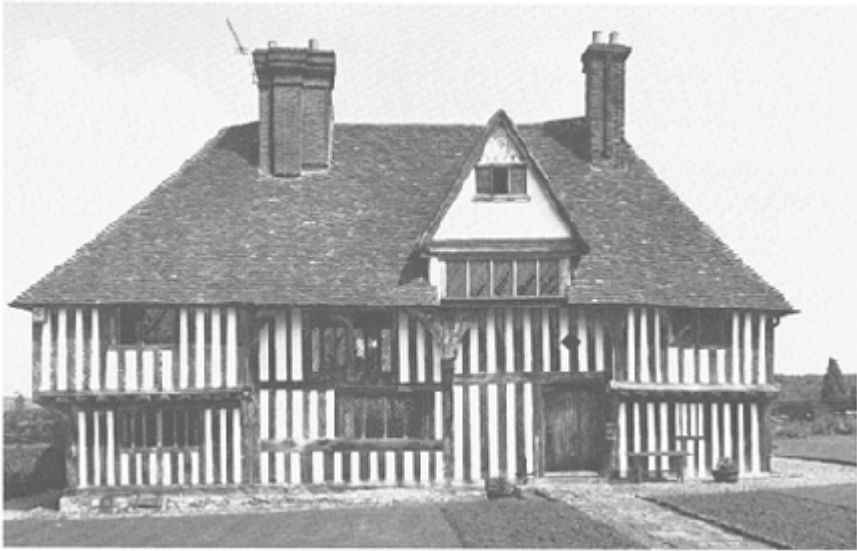
133 A Wealden house of classic plan at Synyards, Otham, Kent, the gable being an addition of 1663; early-sixteenth-century (R.C.H.M.)
