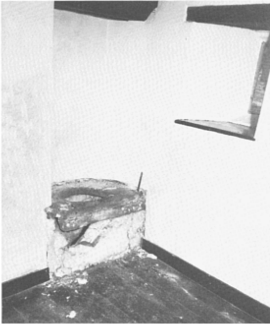
132 The indoor lavatory of the abbots of Glastonbury at Ashbury, in Berkshire, being one of the facilities newly provided at this late-fifteenth-century retreat (R.C.H.M.)
