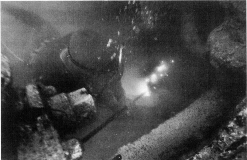
Figure 53. Geoff Kimpton cutting the Xantho engine with the thermal lance (M. McCarthy).
