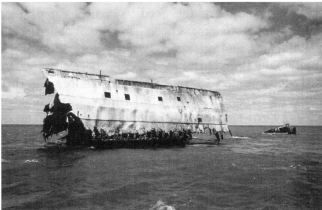
Figure 43 b. View of the SS Alkimos engine room in September 1999. The stem has collapsed into the sea (M. McCarthy).
