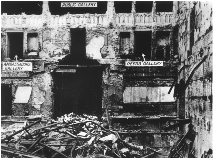
Fig. 5.26. Air raid damage: the House of Commons.
