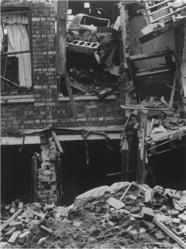
Fig. 5.23 ( left ). Manchester air raid damage.
