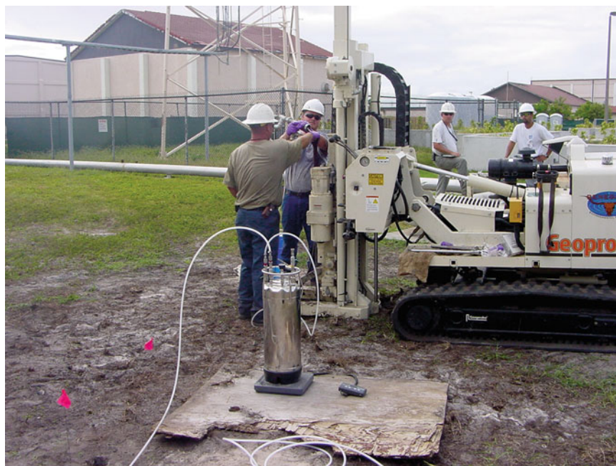
Figure 5.2. Photo of direct push injection of bioaugmentation culture.
