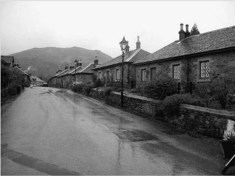
Conservation of the built environment in the village of Luss on Loch Lomond. Photo by Glyn Bissix.
