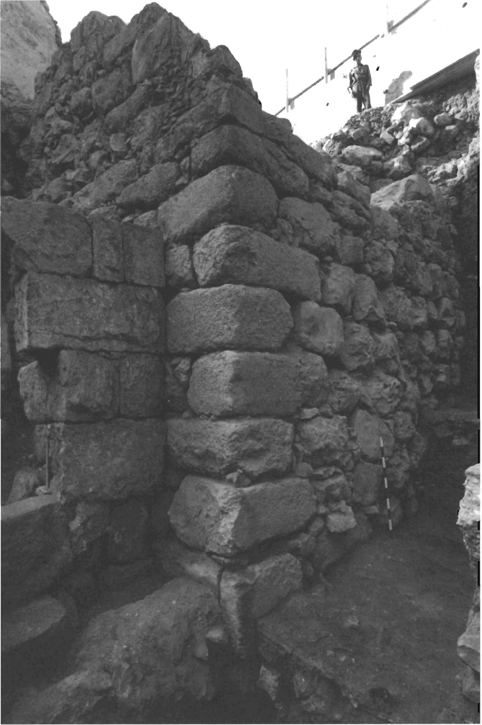
Fig. 7.7. Area W, corner of fortification W.4006–W.4030, the Israelite Tower
