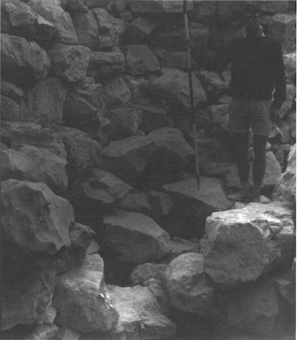
Fig. 16.4. Square A/XXIII, showing part of the stepped structure made of very large boulders laid in courses
