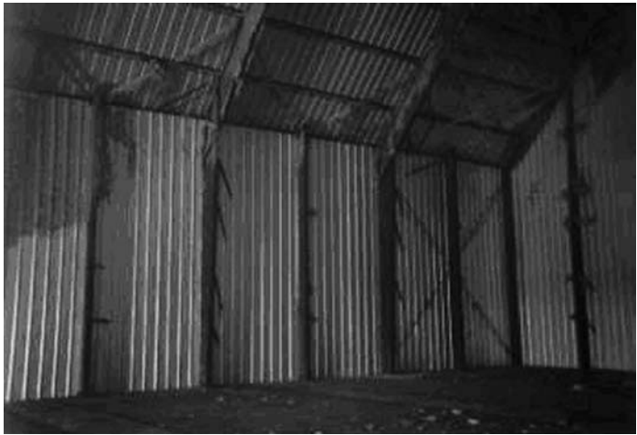
Figure 4-2. Interior framing.
