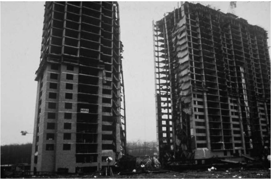
Figure 5-6a, b. Collapse of Skyline Plaza, Bailey's Crossroads. Courtesy National Bureau of Standards/National Institute of Standards and Technology.
