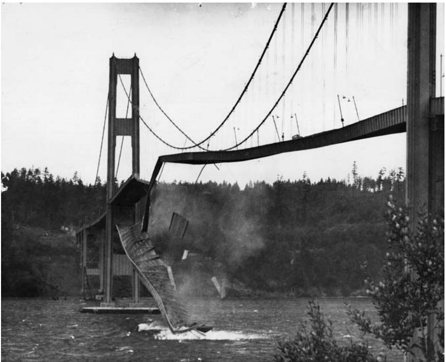
Figure 2-11. Tacoma Narrows Bridge collapse.
