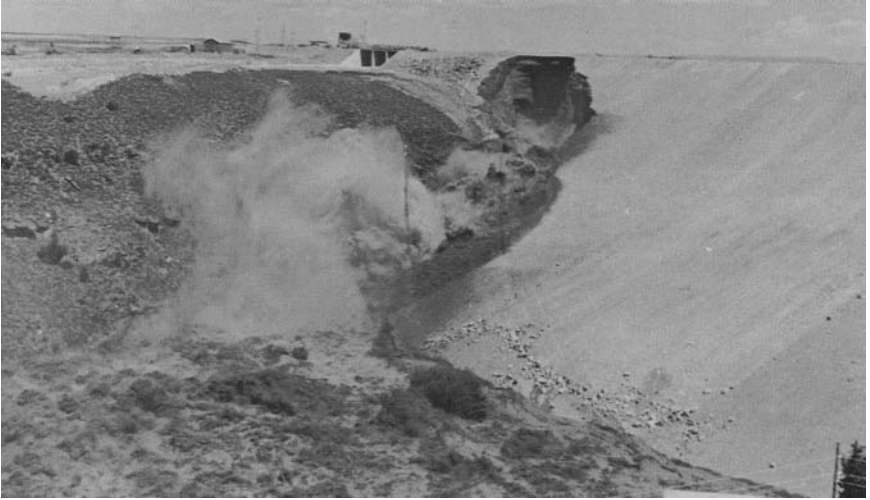
Figure 7-3c. Failure sequence, beginning of final failure. Source: Independent Panel (1976).
