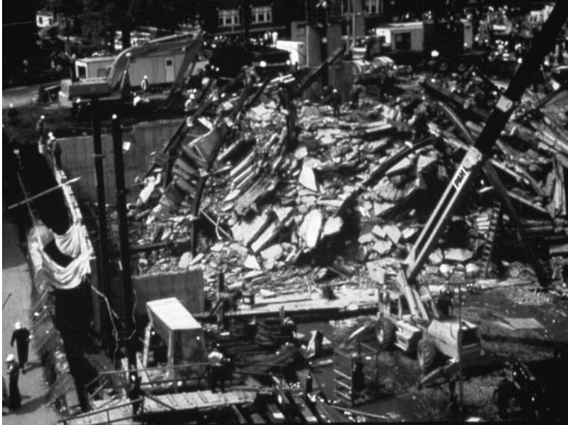
Figure 4-12a, b. The collapsed structure of L'Ambiance Plaza. Courtesy National Institute of Standards and Technology.
