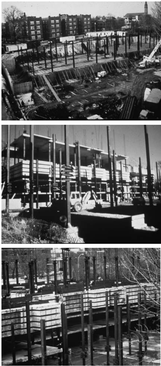
Figure 4-9. L'Ambiance Plaza Lift Slab Construction. Courtesy National Institute of Standards and Technology.
