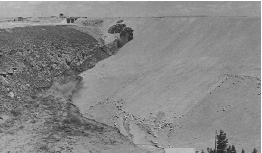
Figure 7-3b. Failure sequence, seepage widens. Source: Independent Panel (1976).
