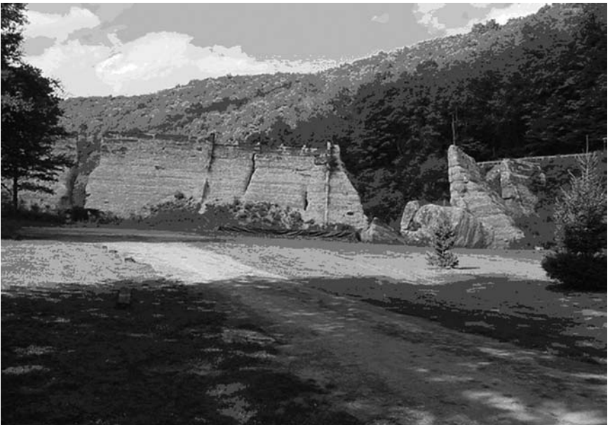
Figure 9-2. The failed Austin Dam.
