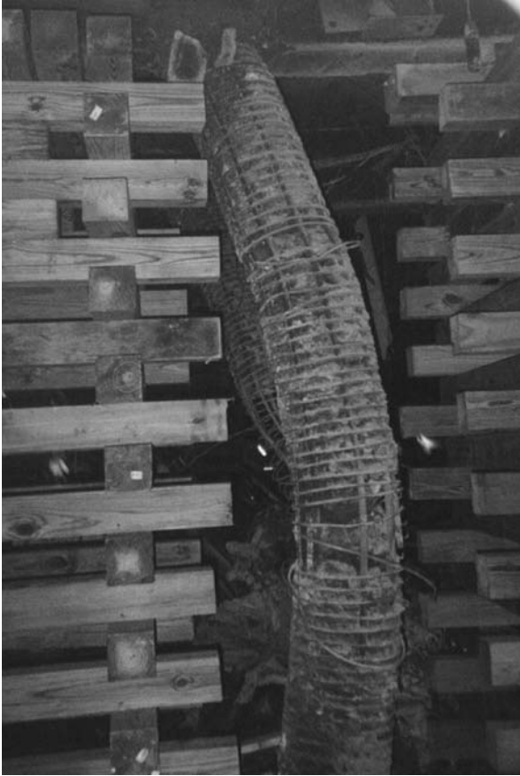
Figure 5-14. Damage to a spiral column.
