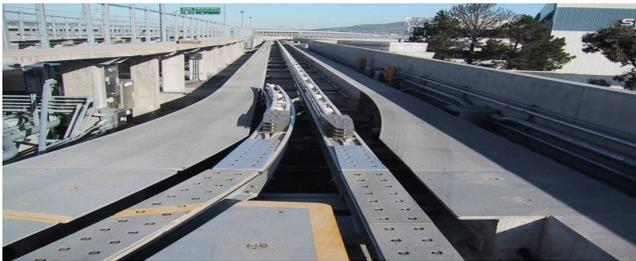
Figure 4: Bombardier Guideway Pivot Switch at San Francisco Airport
