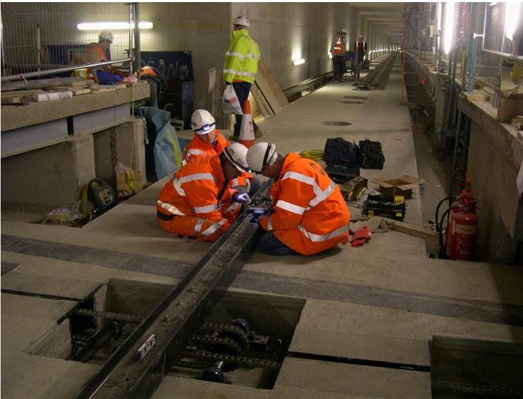
**Figure 7 - T5 concourse A crossover: Transit system guidebeam and switch installation**
