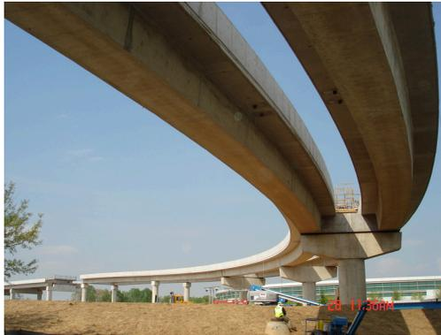
**Figure 4 – Cast-in-place Girders**
