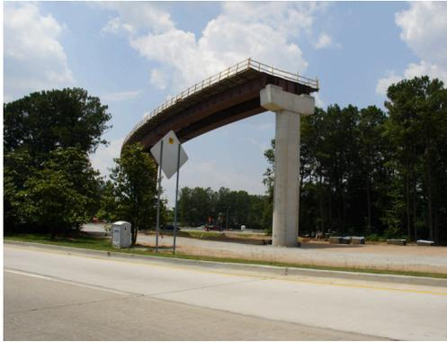
**Figure 5 – Steel “Tub” Girders**
