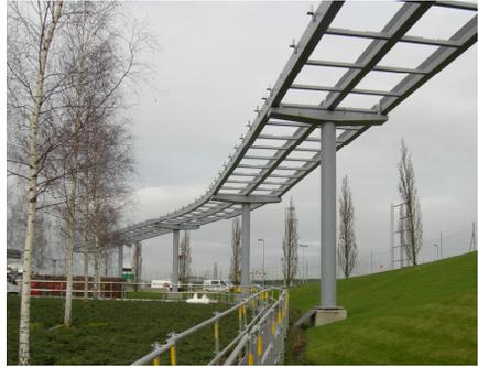
**Photo 1: elevated guideway steelwork**
