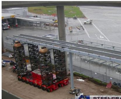
**Photos 6 & 7: installing spans beneath existing structures**
