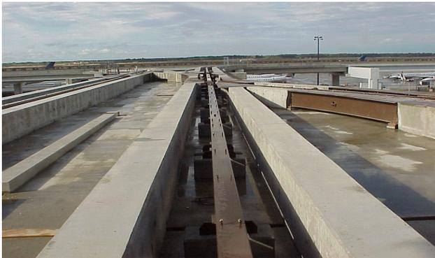
Figure 7: Guidebeam Located between Running Surface
