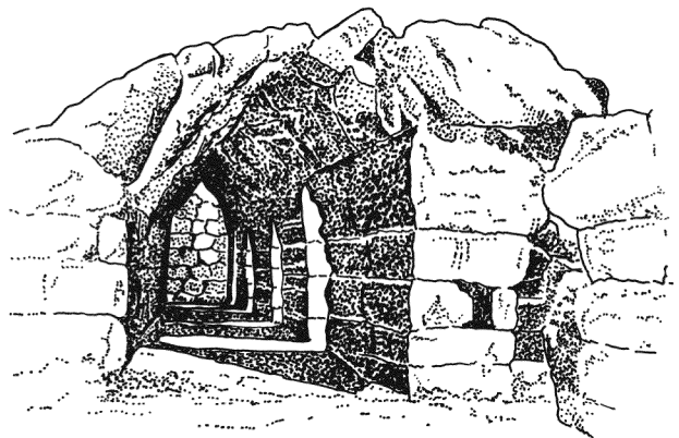
4.49 Storage vaults built into the interior of the massive fortification walls at the citadel of Tiryns near Nafplion. These rooms stored provisions for resisting prolonged sieges.
