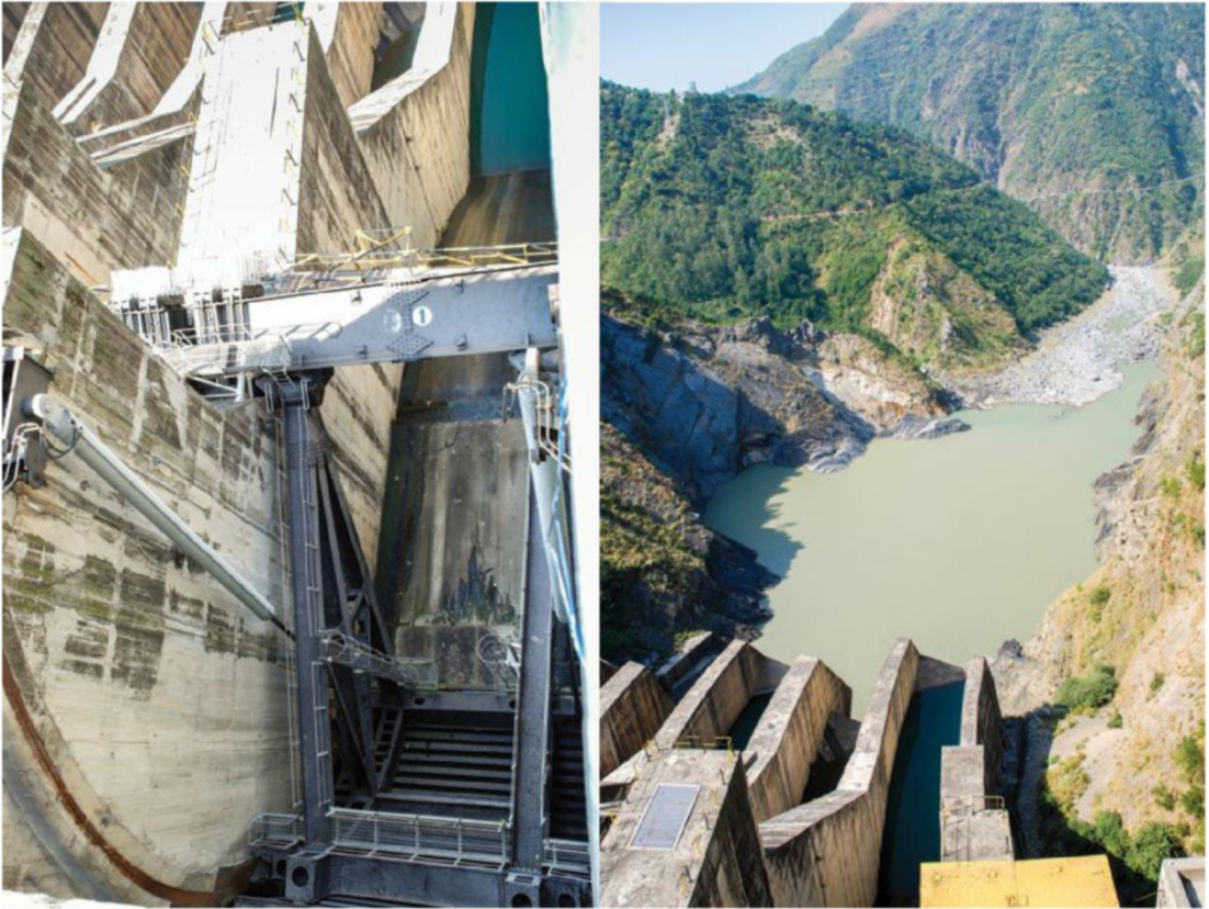
View of construction and spillway in Chamera dam, Himachal Pradesh.
