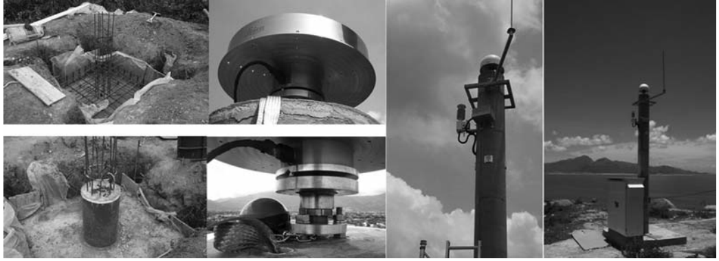
Figure 6-3. Building a reference station.
