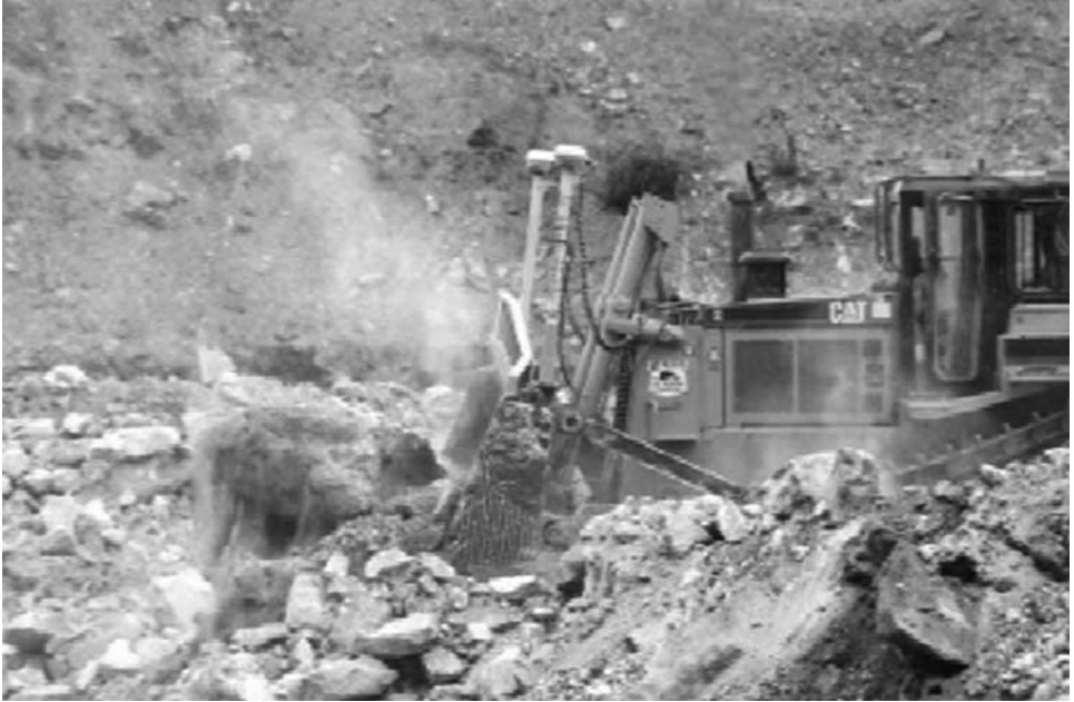
Figure 7-3. A GPS-controlled machine hard at work.
