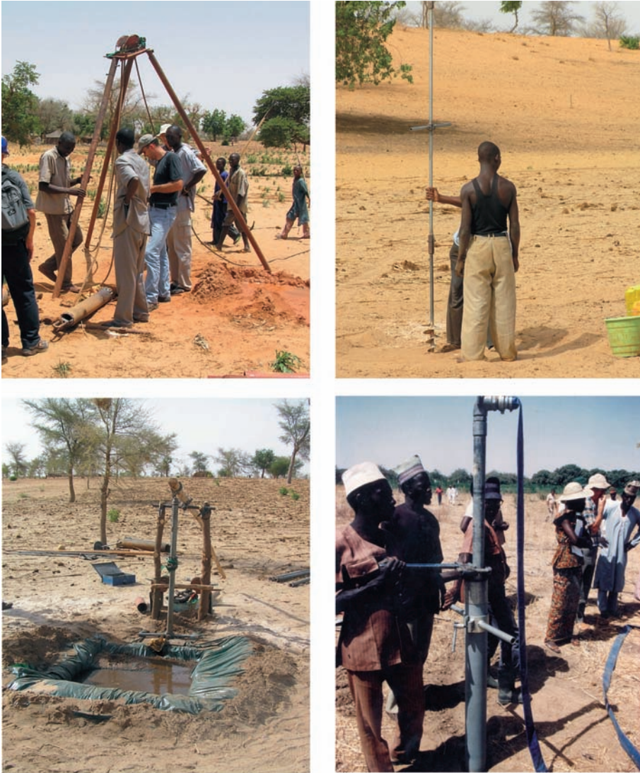
Figure 4. Examples of low cost drilling techniques. Top left hand percussion, top right hand augering, bottom left sludging, bottom right jetting or washboring.
