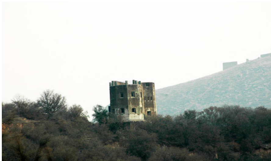
Fig. 3.34 Unexplored heritage structure Gopal Vilas Haudi (Hunting Tower) made by the erstwhile rulers amid the dense forests of Nahargarh Biological Park near Jaipur (Courtesy: Devendra Bhardwaj)
