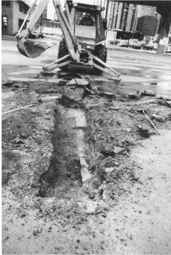
Figure 5.12. A brick foundation wall of the Tremont House, exposed during 1987 excavations. From Richard F. Carrillo, Sarah J. Pearce, Stephen Kalasz, and Daniel A. Jepson, The Tremont House (5DV2954): Historical Archaeological Investigations of an Early Hotel in Denver, Colorado (Denver: Colorado Department of Transportation, 1993); reproduced by permission.
