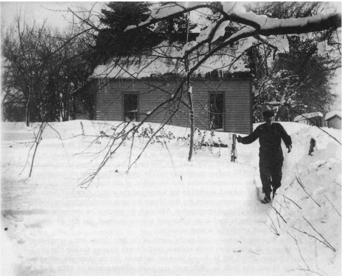
Figure 5.34. The Bee House, winter 1880. Photograph courtesy of Four Mile House Historical Park.
