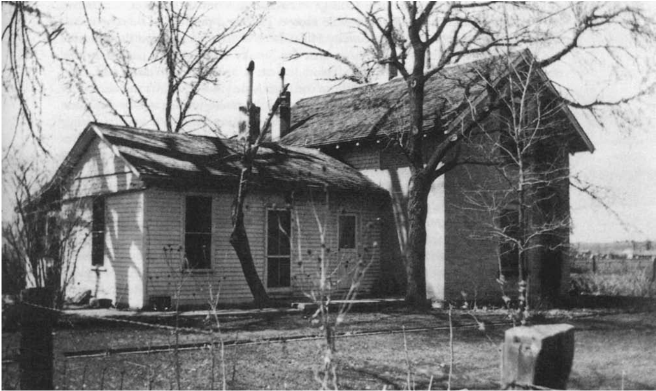
Figure 5.36. The Working House. Photograph courtesy of Four Mile House Historical Park.
